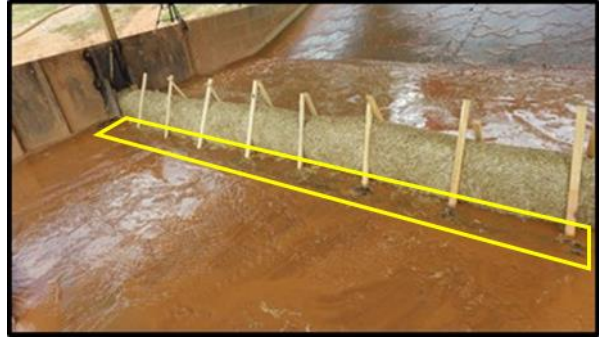
(b) sediment-laden flow - fabric underlay installation
