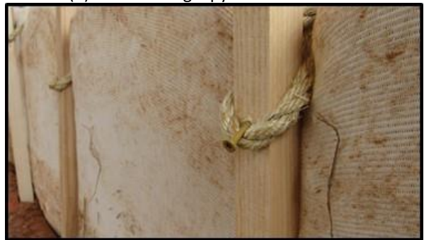
(f) rope installation – wood screw catch
