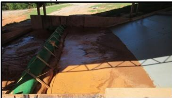
(g) SiltSoxx sediment deposition
