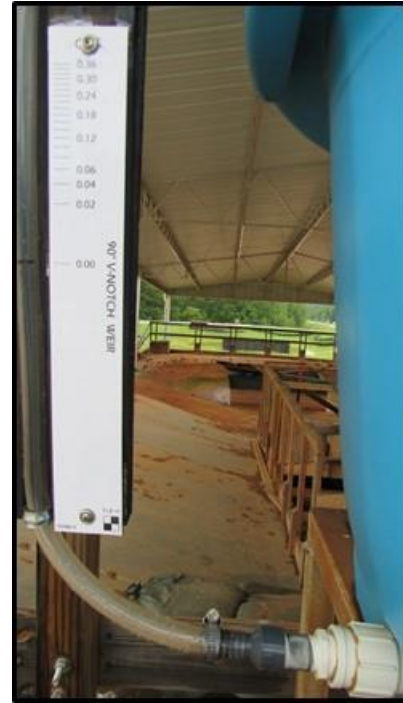
(e) flow rate monitoring
