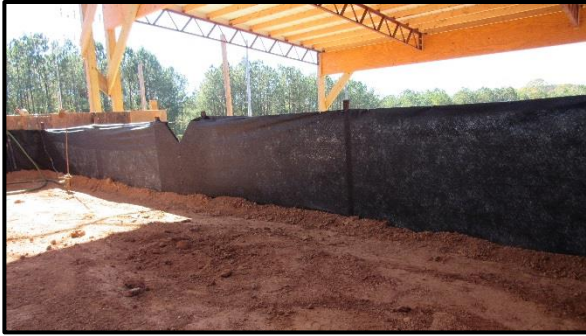
(a) upstream vantage point
