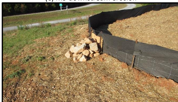
(g) field installation - downstream
