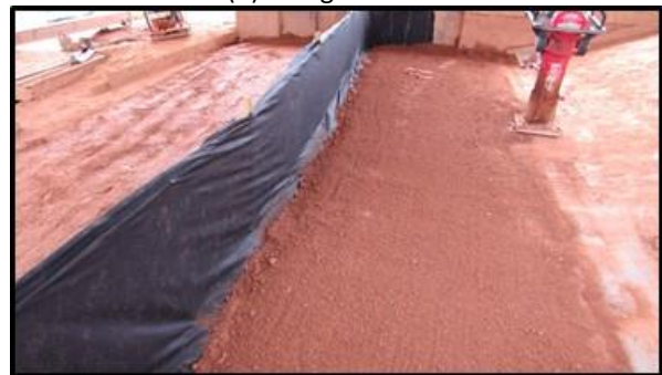
(f) offset silt fence installation
