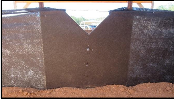
(c) front of weir
