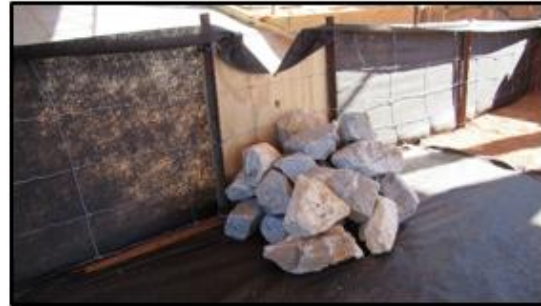
Figure 1: Sediment Barrier Installation
