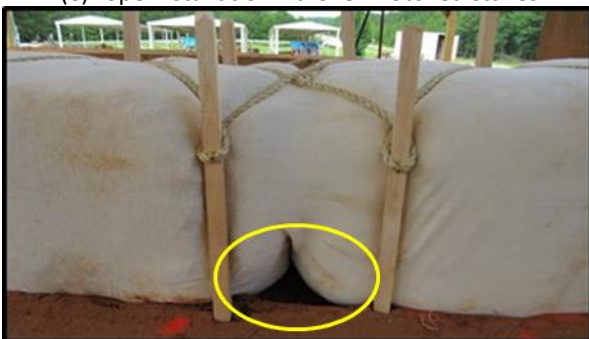
(g) rounded end abutment void
