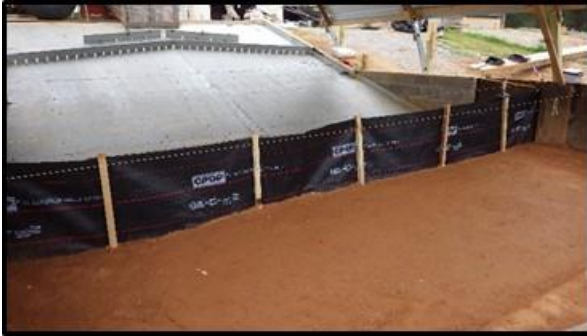
(a) system installation
