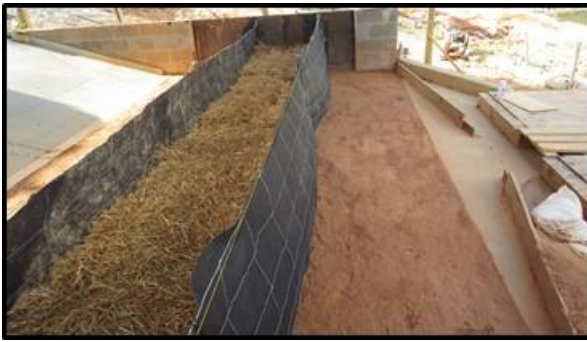
(a) SRB installation
