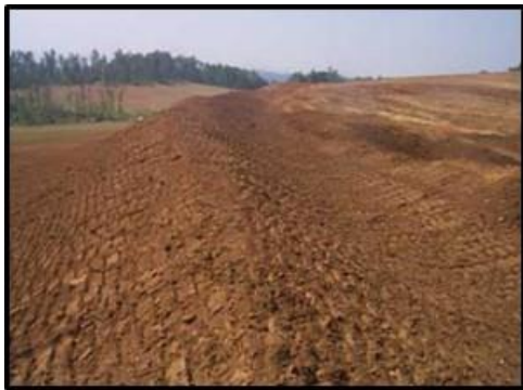
(a) compacted diversion ( AL-SWCC 2014 )
