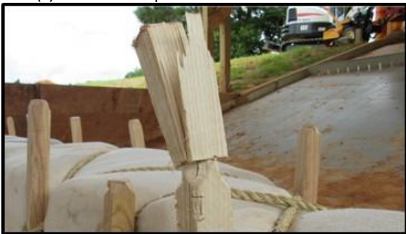
(e) rope installation - broken notched stakes
