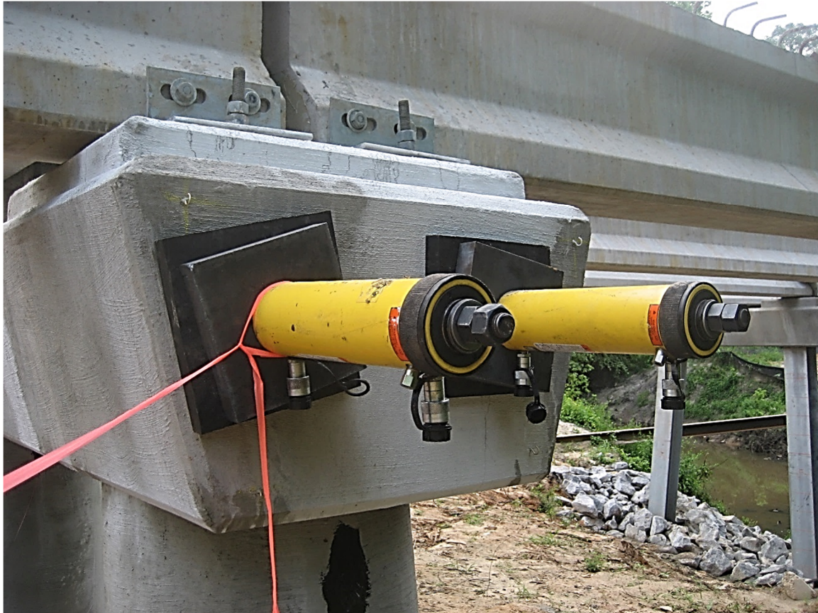
Figure 4-9 – Enerpac RRH3010 Hydraulic Jacks
