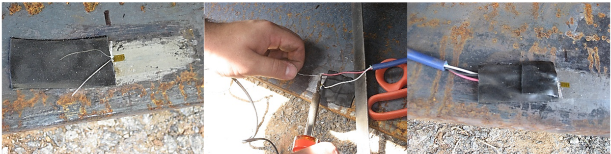
Figure 4-3 – Process of Wiring and Protecting Applied Strain Gage
