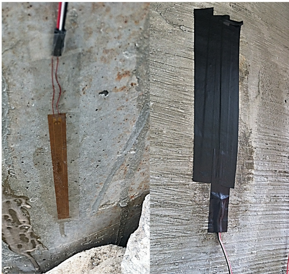
Figure 4-5 – Concrete Strain Gage and Initial Layer of Protection
