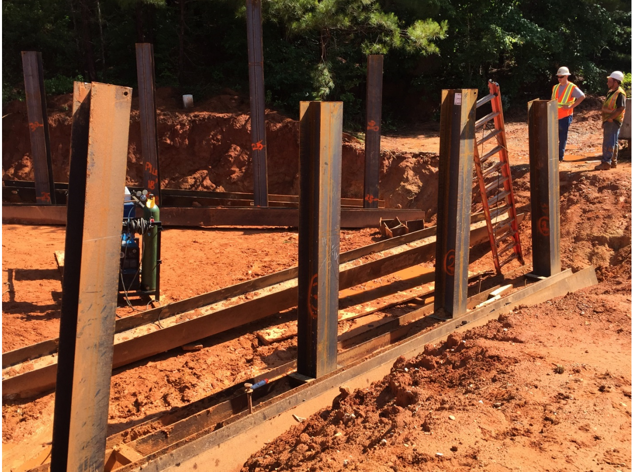
Figure 4-30 – AUNGES Piles Prior to Cut off and Cap Construction
