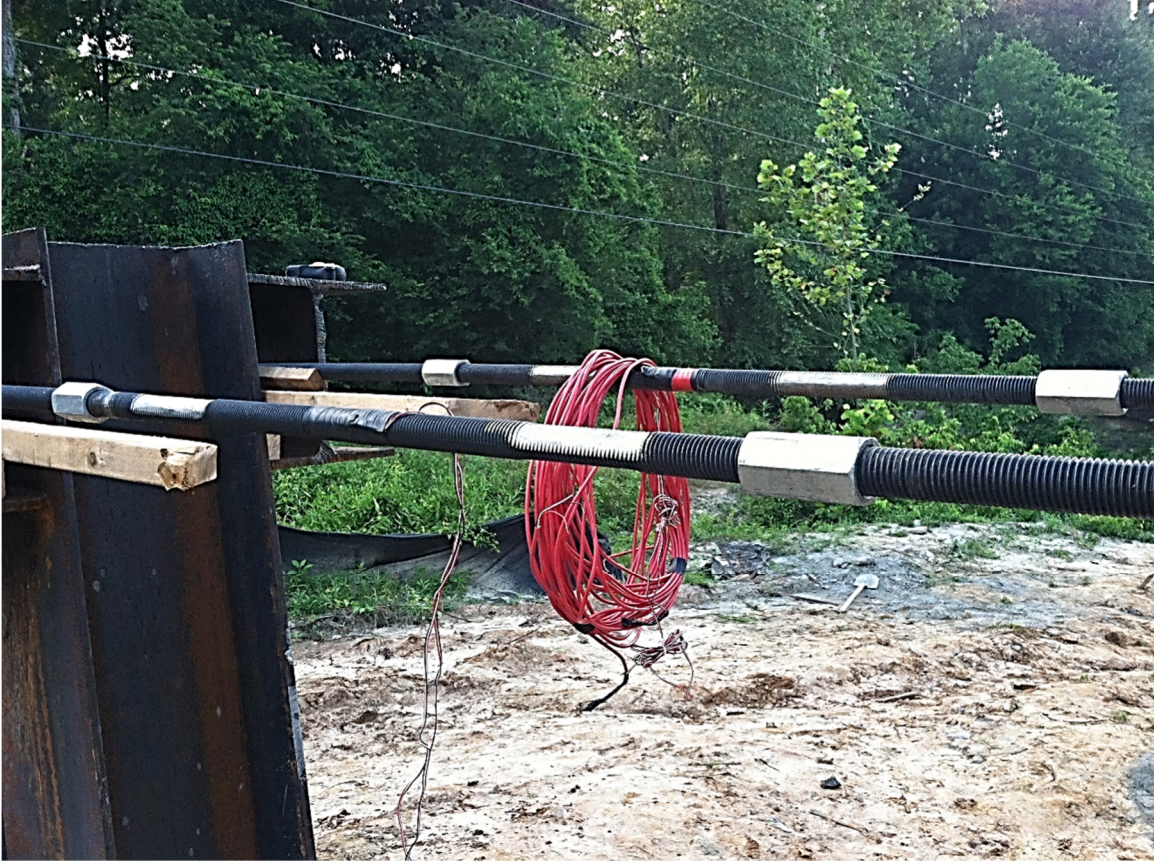
Figure 4-7 – Instrumented Threaded Rods prior to Load Testing
