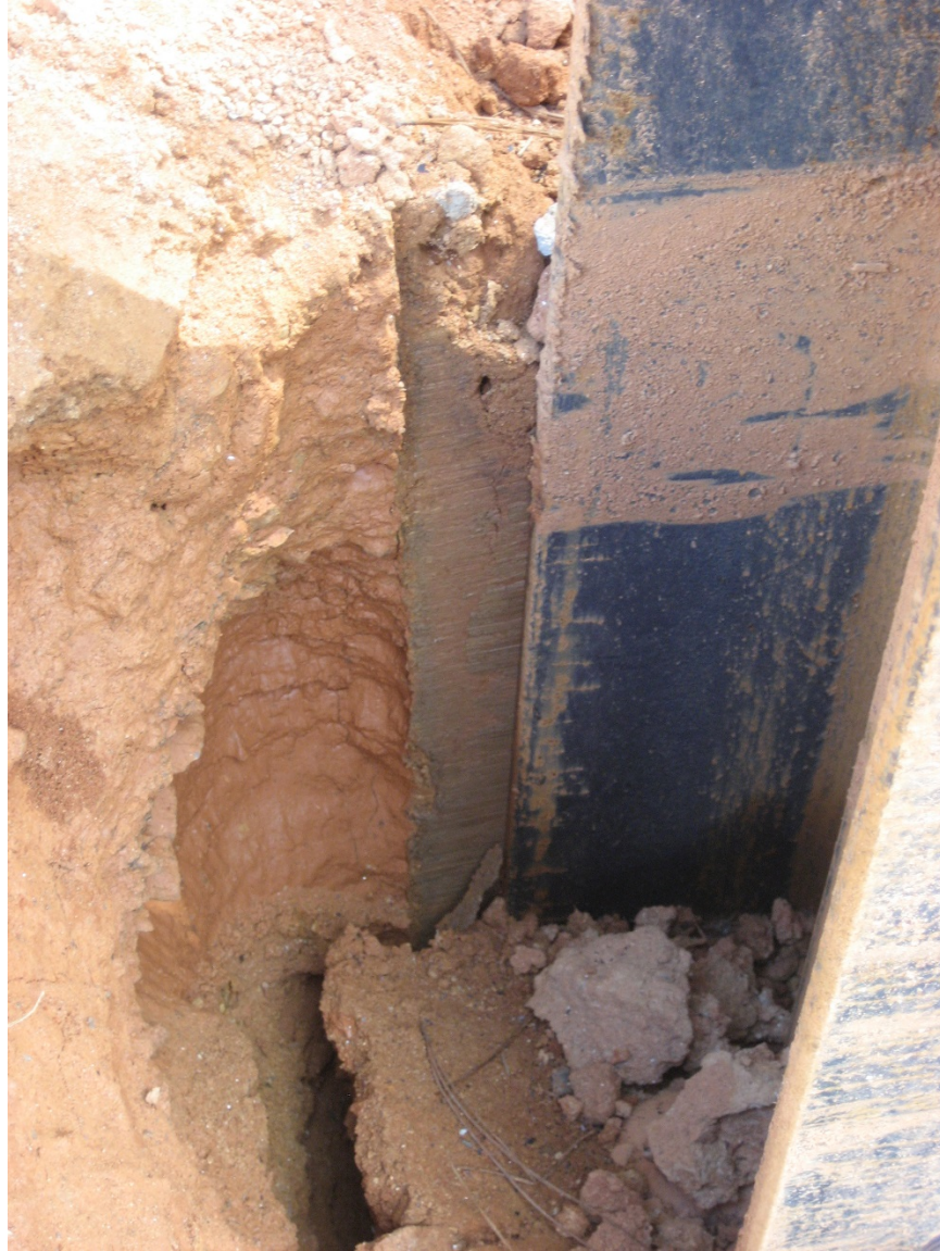
Figure 4-54 – Lateral Displacement of Test Pile
