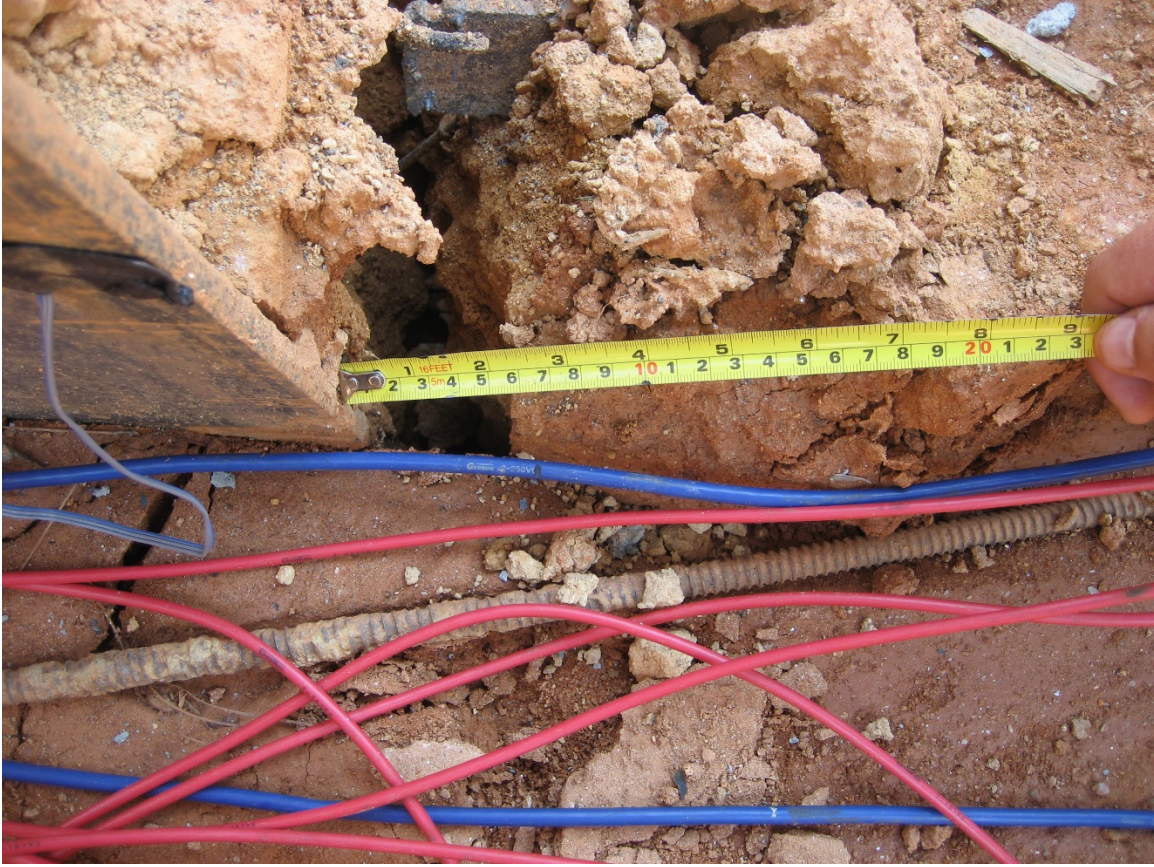
Figure 4-43 – Residual Drift due to Lateral Load Test
