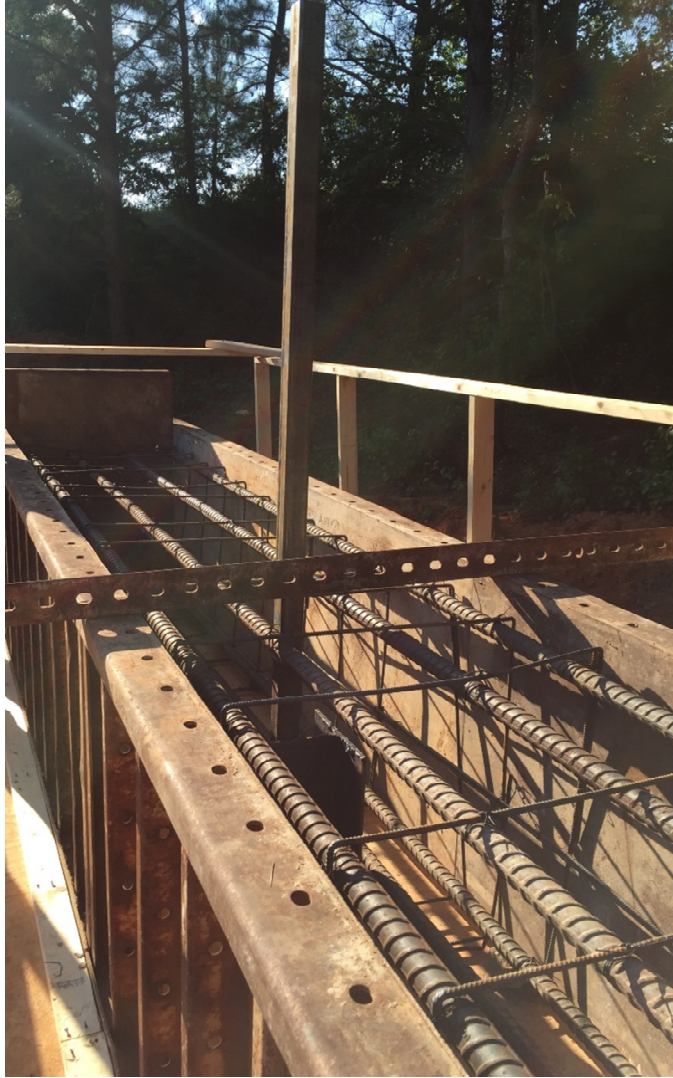
Figure 4-33 – AUNGES Pile Cap Reinforcement Cage
