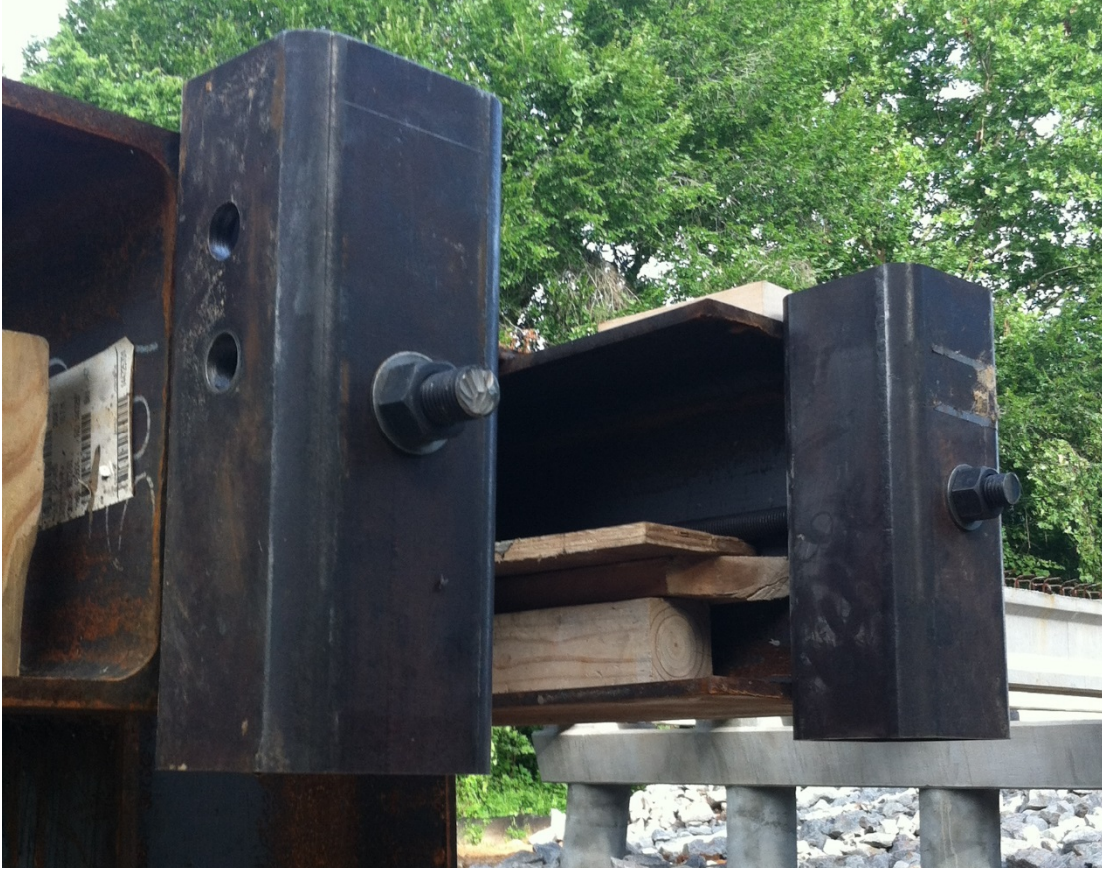
Figure 4-19 – Hollow Steel Tube Sections Bearing Against the Reaction Bent
