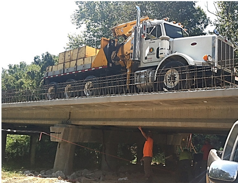
Figure 4-24 – Placement of Load Truck over the Edge Girder
