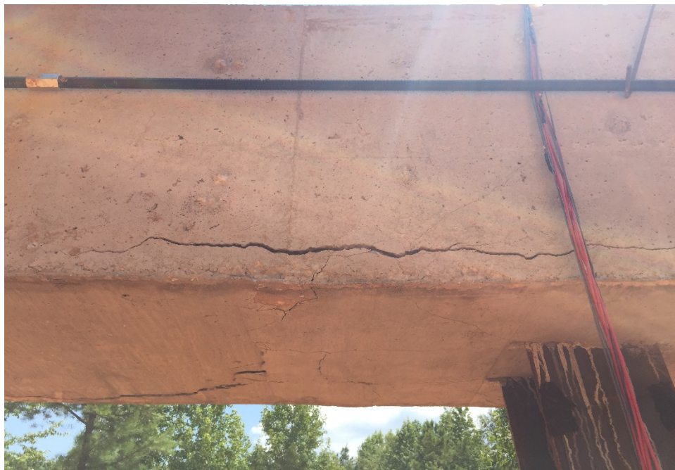
Figure 4-40 – Bent Cracking
