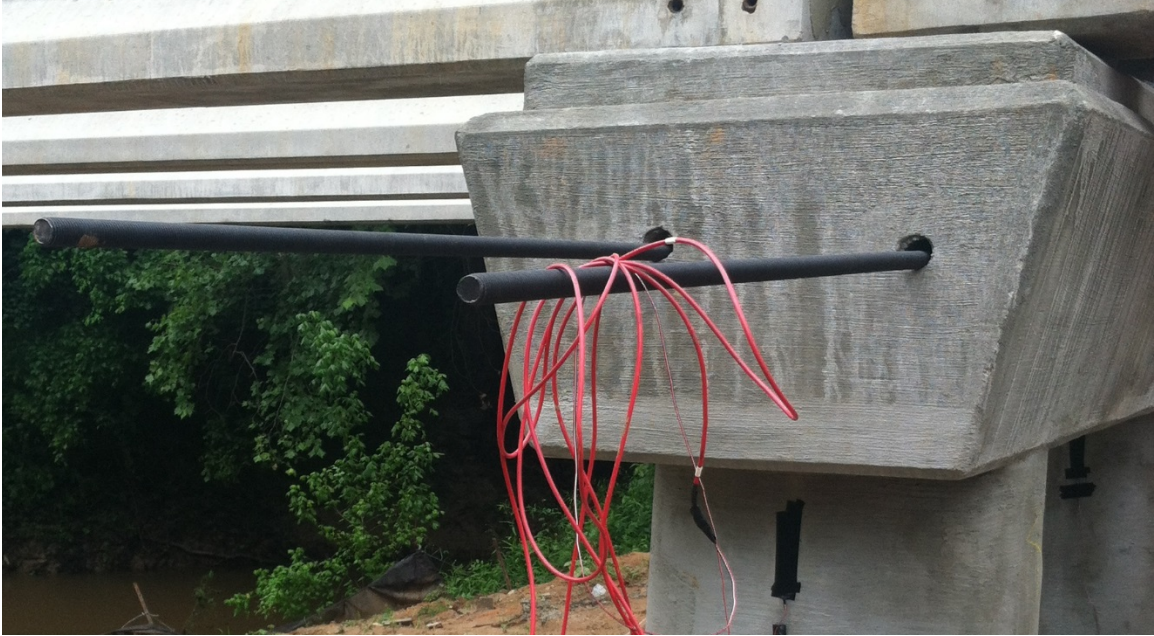
Figure 4-20 – Threaded Rods Passing through PVC Sheathing in the Bent Cap
