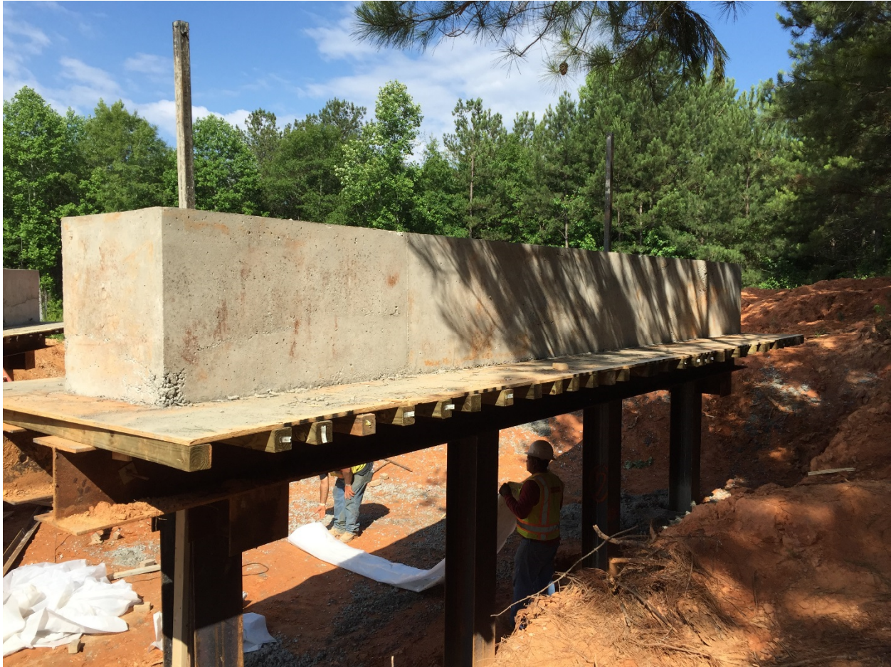
Figure 4-34 – Completed AUNGES Test Bent
