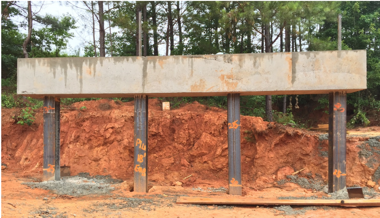
Figure 4-44 – AUNGES Vertical Pile Bent
