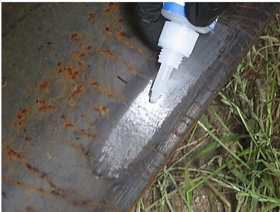
Figure 4-1 – Application of Epoxy to Prepared Strain Gage Location
