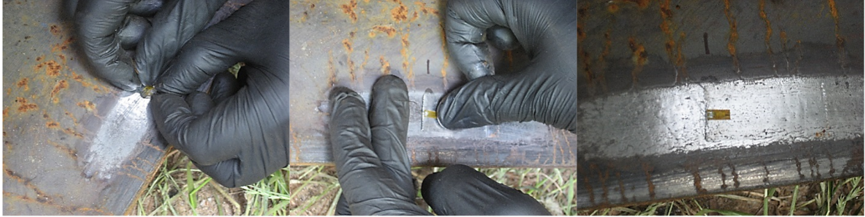
Figure 4-2 – Process of Adhering Strain Gage to the Steel Pile
