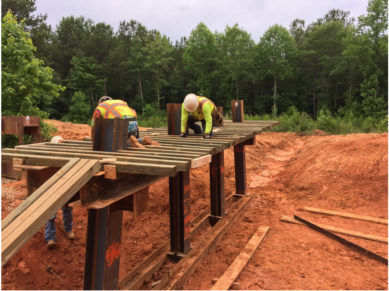
Figure 4-31 – AUNGES Pile Cap Construction
