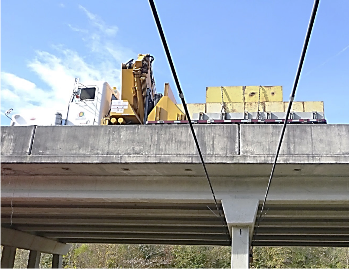
Figure 4-29 – Load Truck on Highway 331 Test Bent
