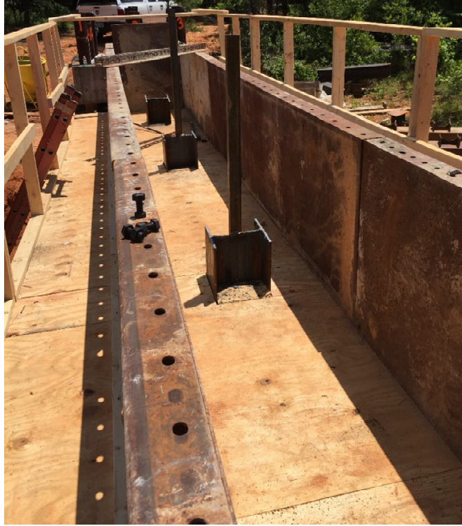
Figure 4-32 – AUNGES Pile Cap before the Addition of the Reinforcing Steel
