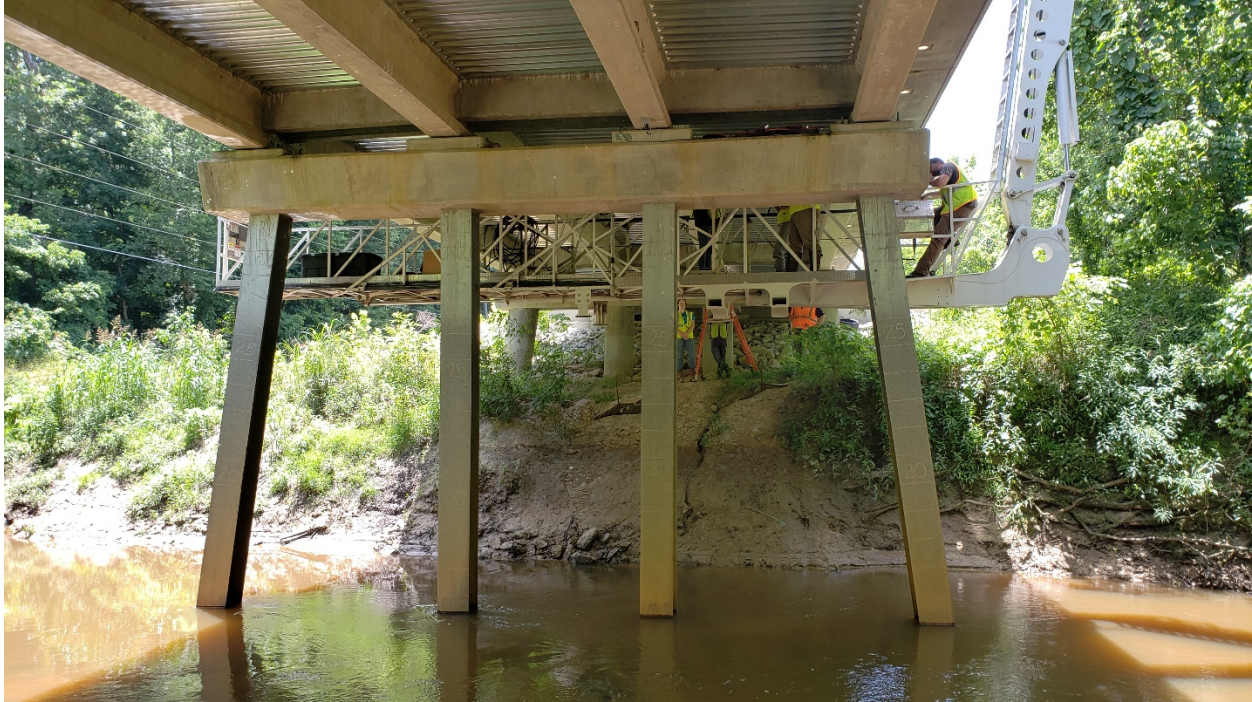
Figure 1-2 – HP Pile Bents Typical of Alabama Bridges
