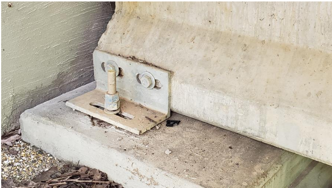
Figure 3-3 – Expansion Joint Connection
