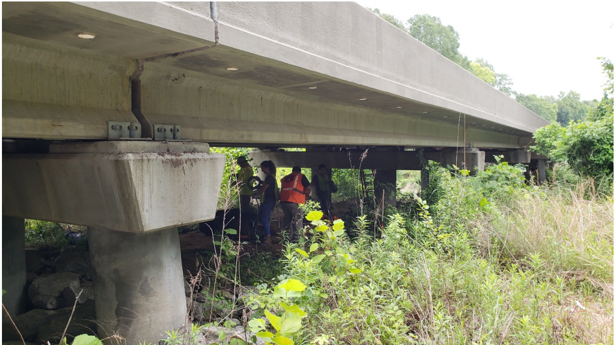
Figure 1-1 – Side View of a Typical ALDOT Multi-Span Bridge
