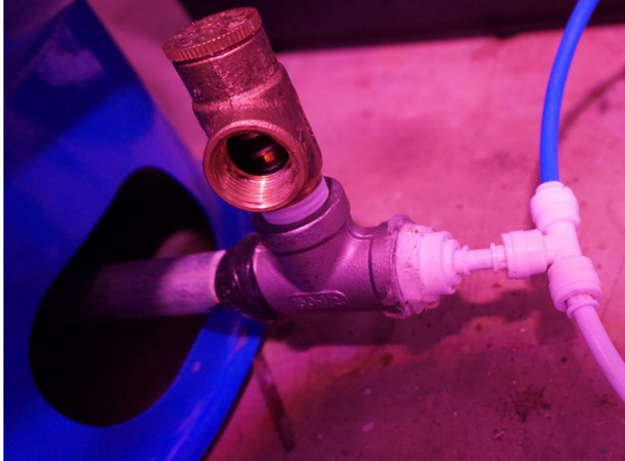
Figure 43: Pressure Relief Valve with 1/4" Total Reduction.
