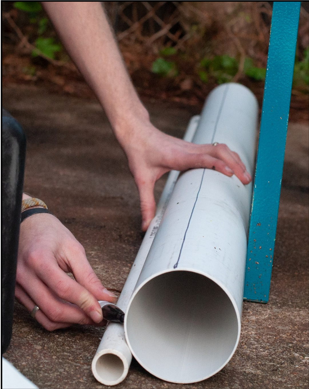
Figure 52: Step Four of Tower Fabrication.
