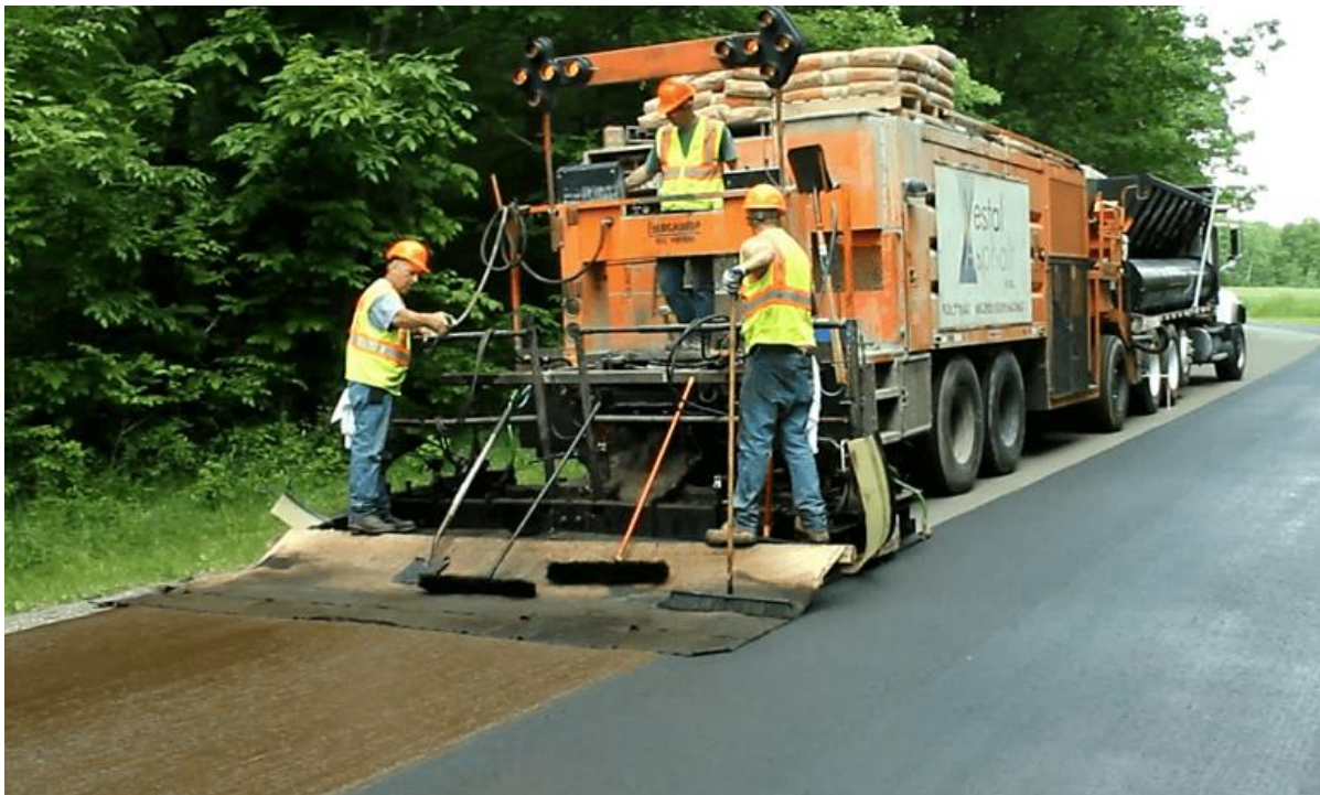
Figure 2-5 Micro surfacing application (37)
