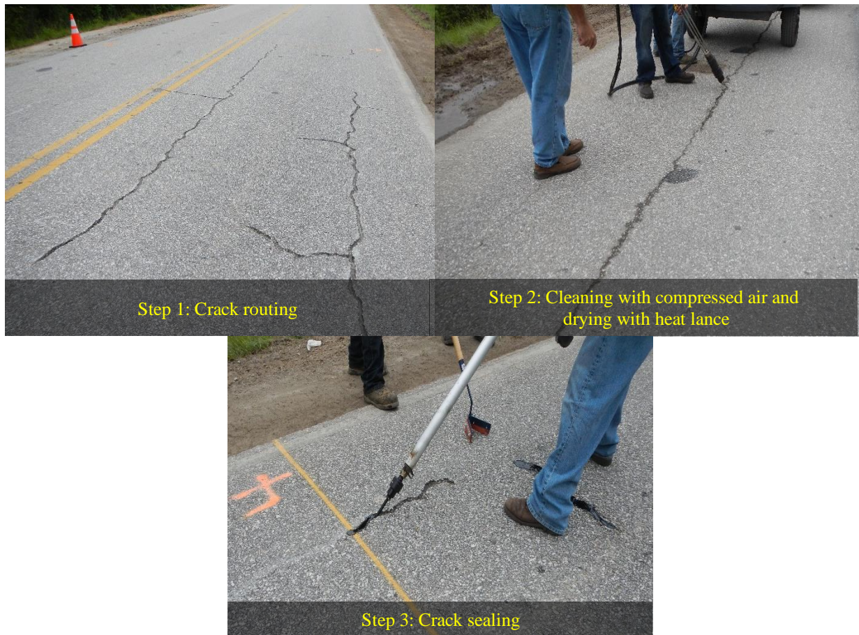
Figure 2-1 Crack rout and fill procedure (photos courtesy of NCAT)
