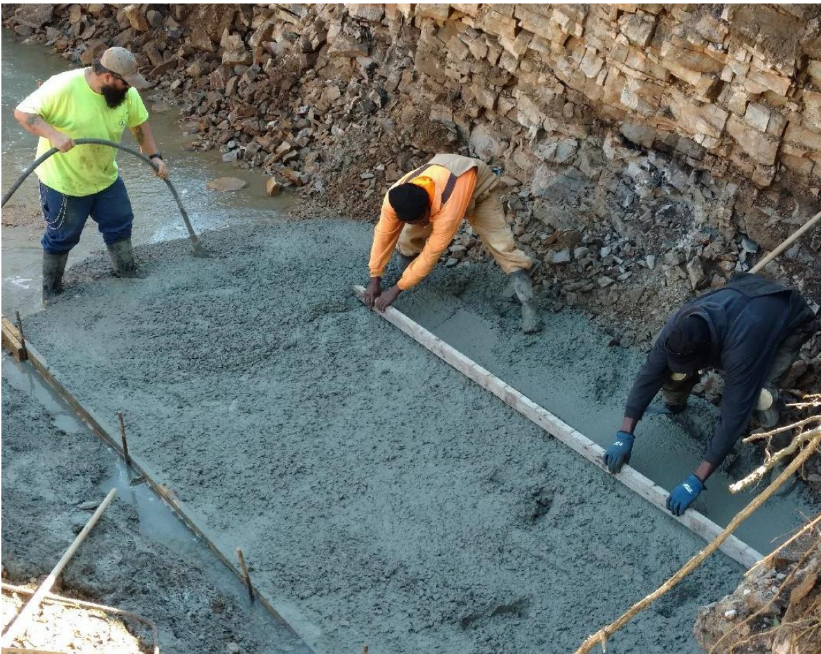
Figure 33. Construction of east abutment concrete levelling pad foundation.
