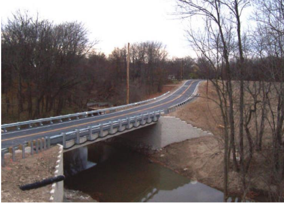
Figure 16. Bowman Road GRS-IBS in Defiance County, Ohio ( defiance-county.com )
