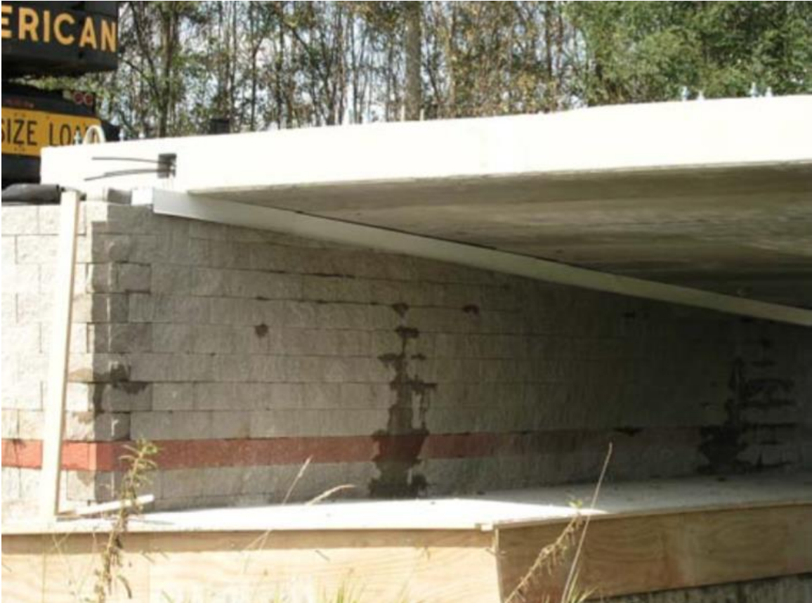
Figure 23. Aluminum fascia drip-edge (Adams et al. 2011a).
