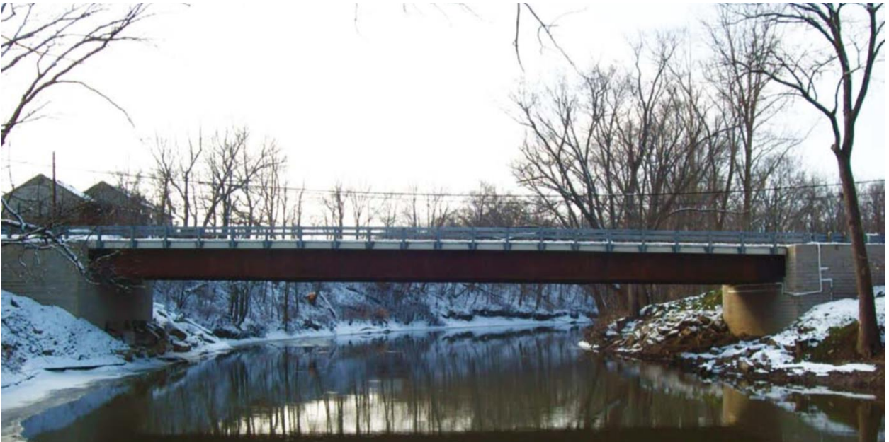
Figure 1. Defiance County, Ohio GRS-IBS spanning Tiffin River (Adams et al. 2011a).
