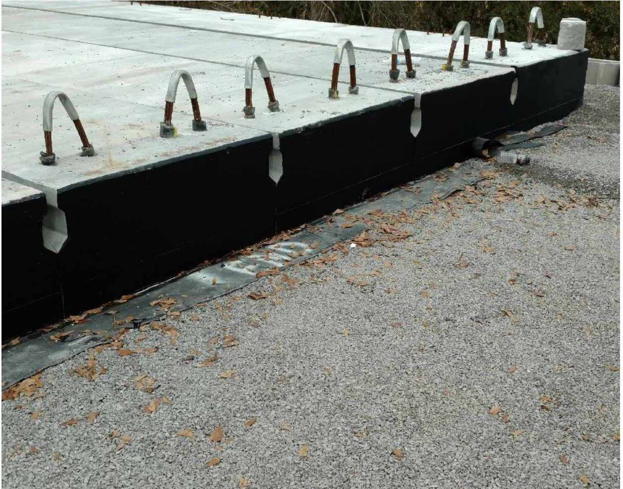
Figure 56. Bituminous coating on beam ends at Marshall County GRS-IBS.
