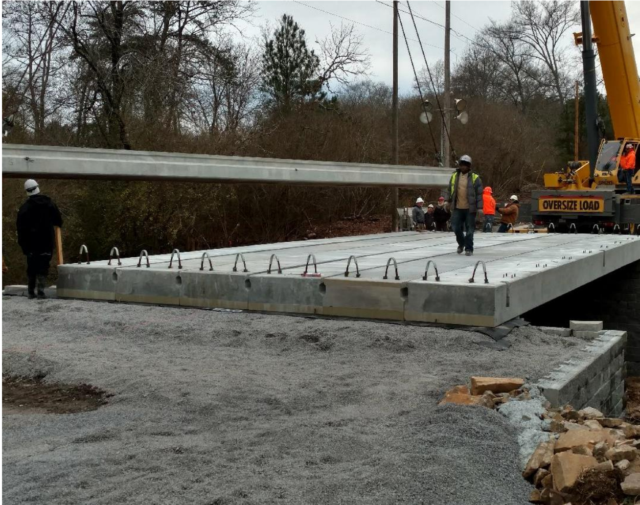
Figure 38. Placement of final precast concrete beam atop the beam seat.
