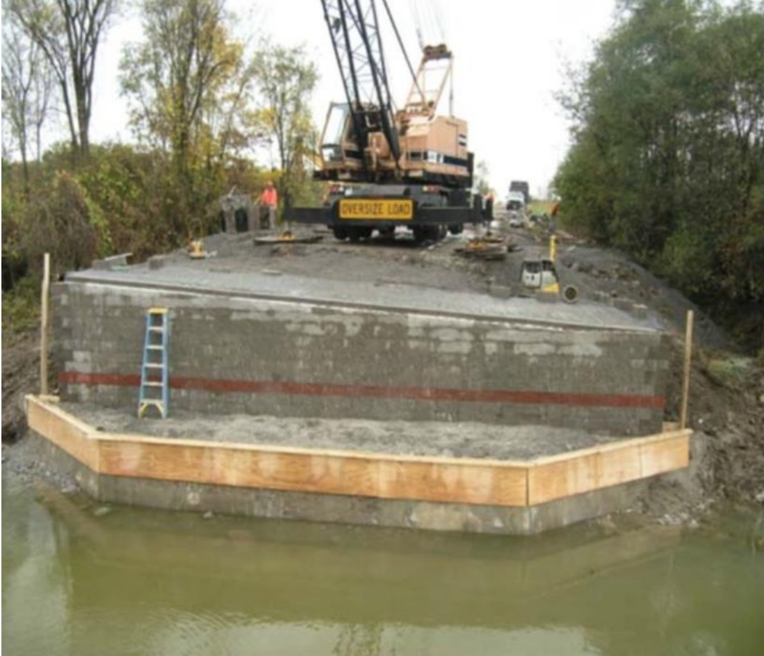
Figure 20. Superelevated GRS wall in St. Lawrence County, NY. It should be noted that this wall was constructed behind an existing concrete abutment (Adams et al. 2011a).
