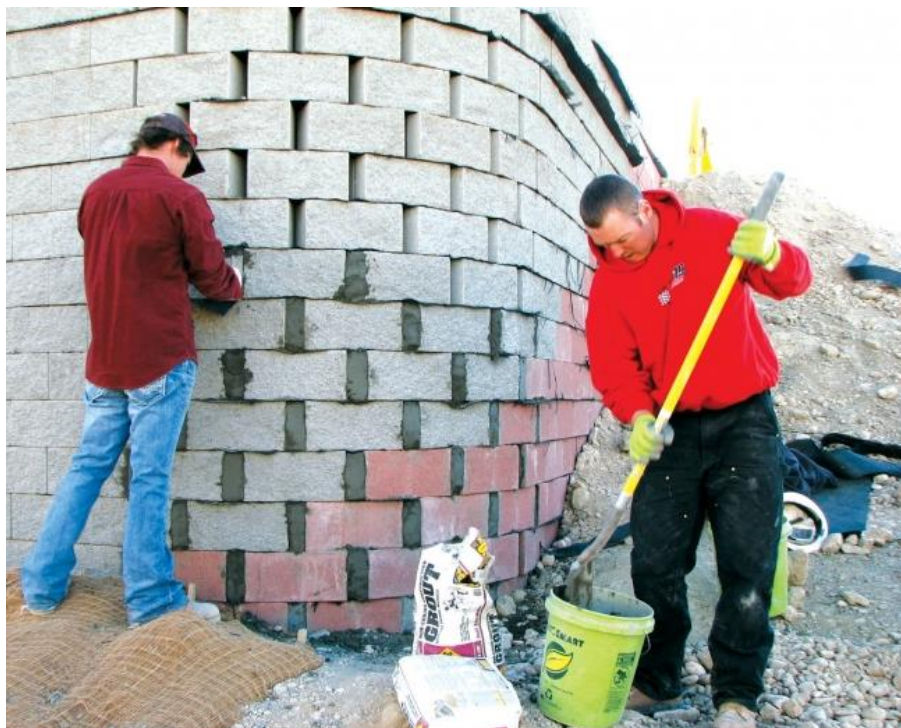
Figure 21. Filling cavities in wall with non-shrink cement (Abernathy 2014).
