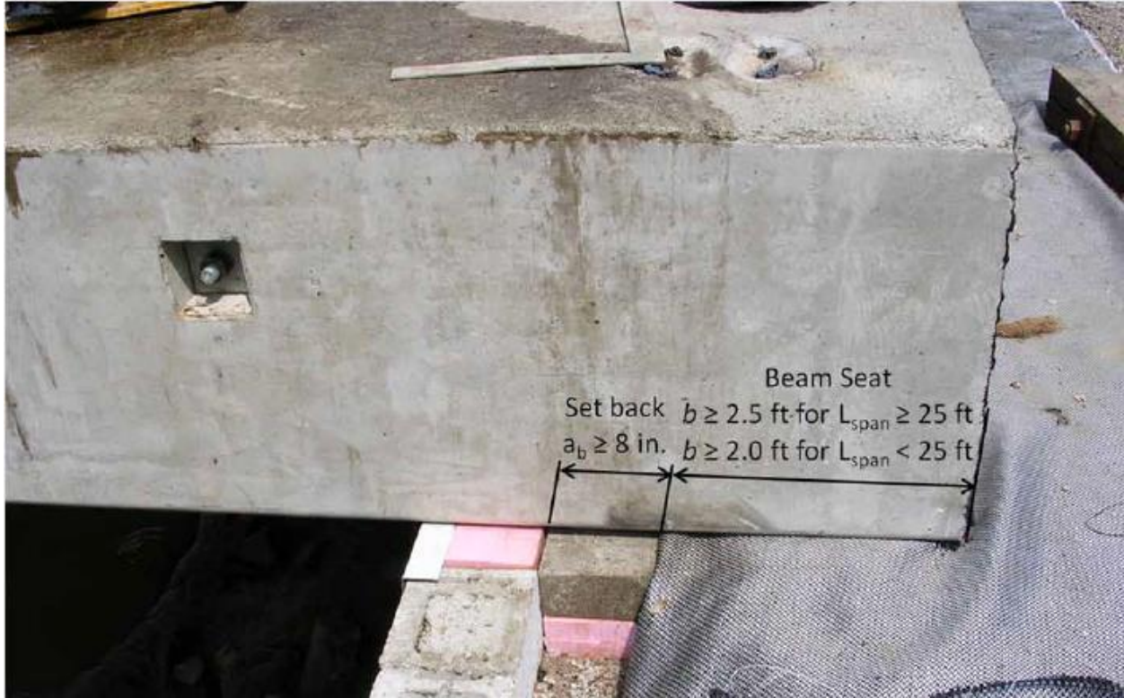
Figure 24. Bridge beam seat and setback distance dimensions (Adams et al. 2011a).
