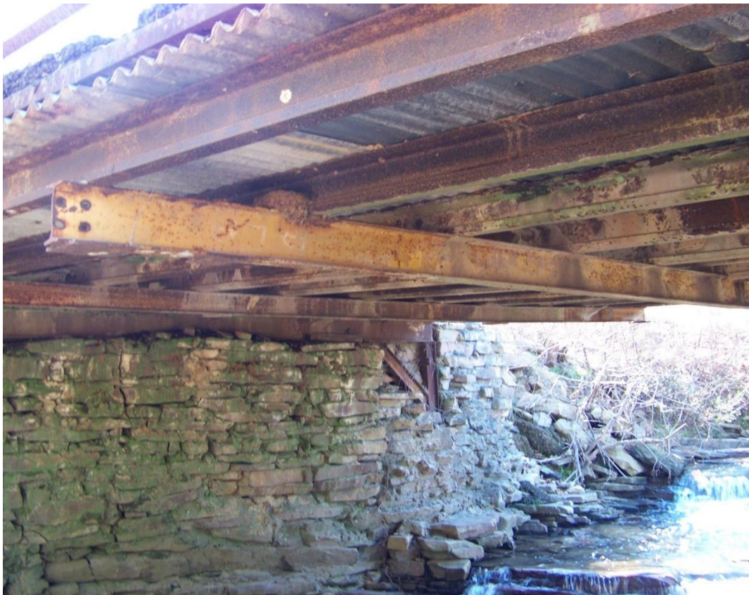
Figure 32. Existing Bridge Superstructure and Abutments.
