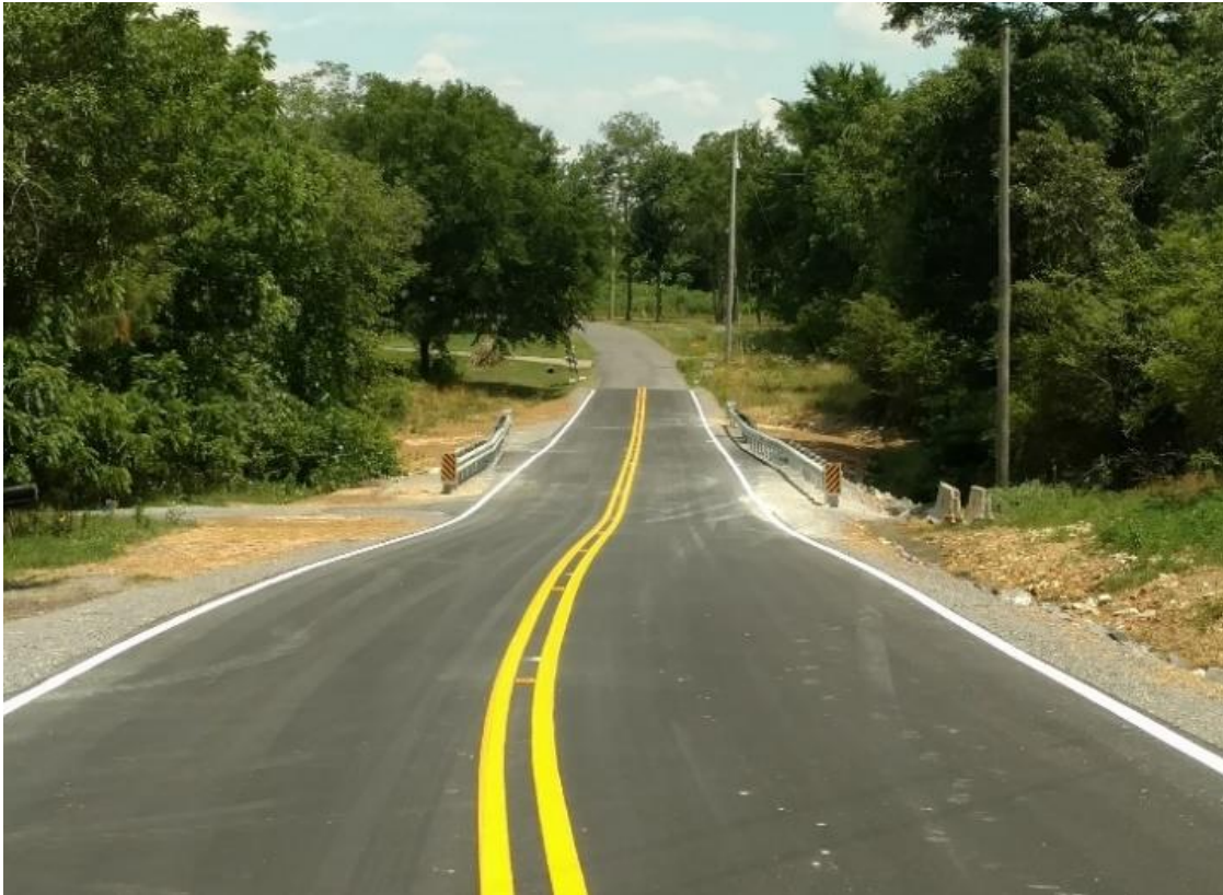
Figure 39. The completed GRS-IBS over Turkey Creek in Marshall County, AL (from Hogan 2018).
