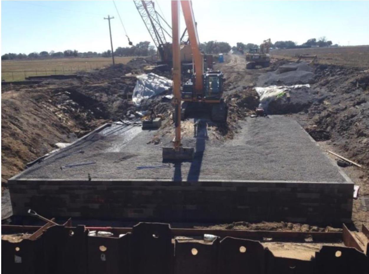
Figure 14. Maree-Michel GRS abutment construction behind cofferdam (Rauser 2016).
