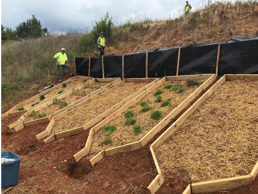
Figure 6. Completed plot installation
