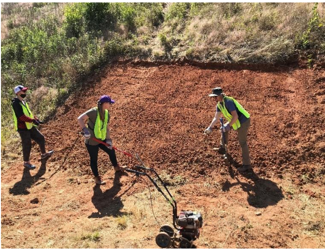
Figure 4. Initial Land Preparation (May, 2020)
