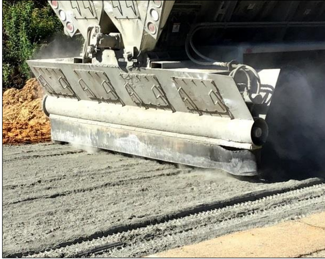
a) Application of Cement
