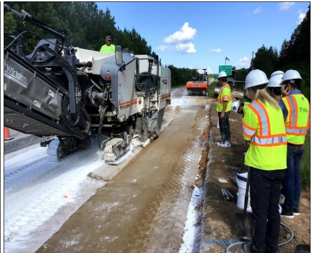
d) Mixing Soil and Lime Together
