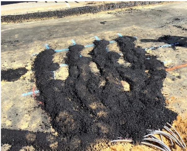
c) Final Protection of Strain Gauges
