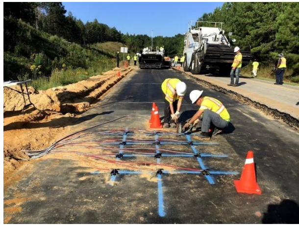
b) The Final Array of Strain Gauges
