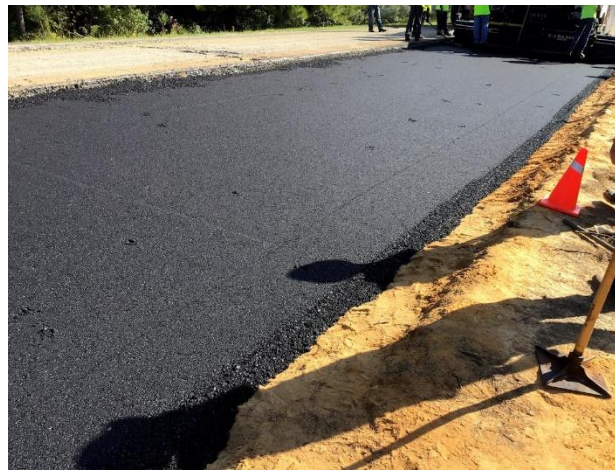
b) AC Layer Before Compaction
