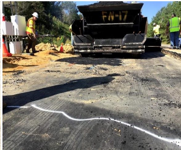
d) Paver Approaching Protected Gauges.
