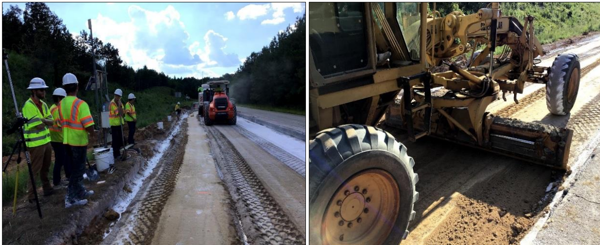
a) LTS Compaction
