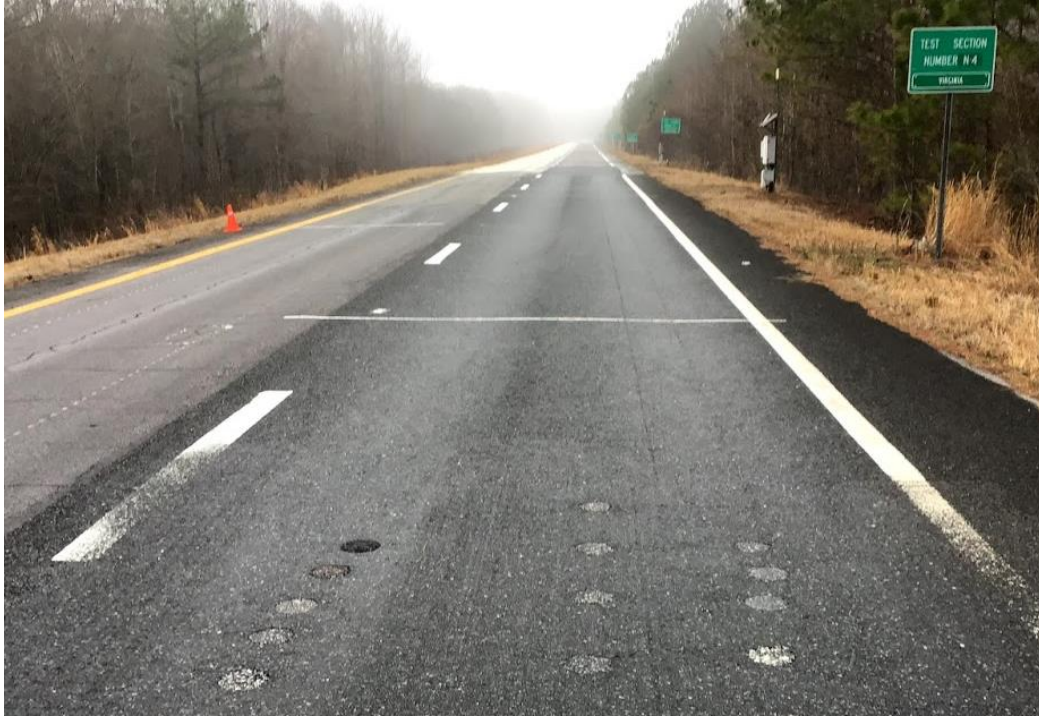
Figure 5.8 The View of the CCPR (N4) Surface Pavement Section (Date Taken: 01/25/2021).
