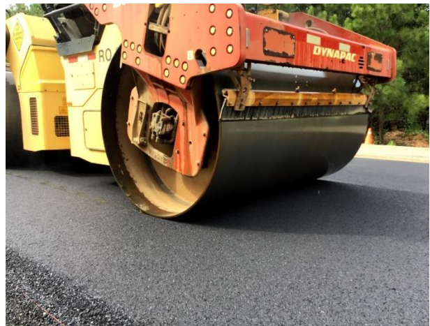
d) Finalizing S2 Construction (top layer)
