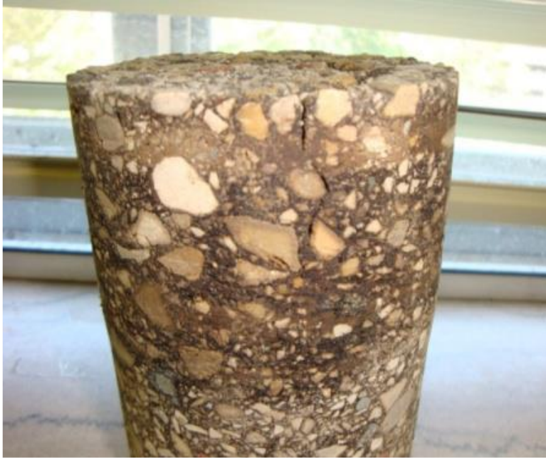
Figure 2.3 A Top-Down Crack on a Stabilized Foundation Pavement (Wen et al. , 2014).
