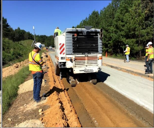
b) Mixing Cement and Soil
