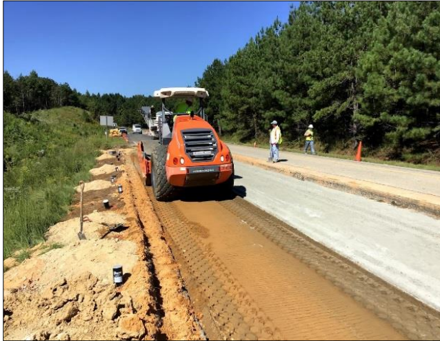
c) Compaction of the Layer
