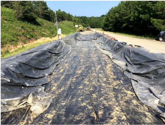
c) Subgrade Tarp Protection.
