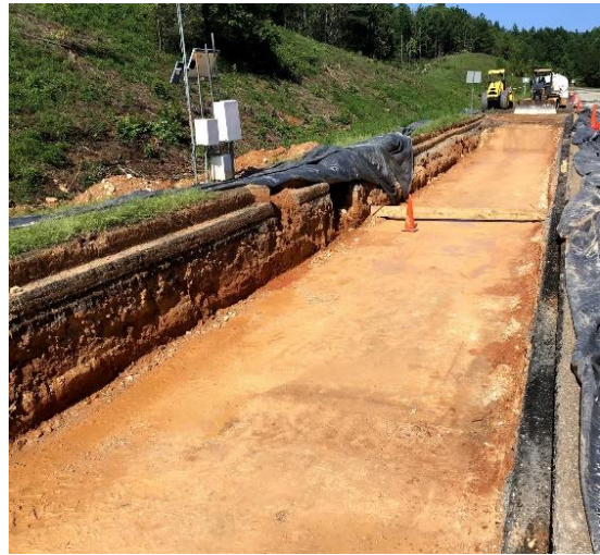
d) Subgrade Sun Drying
