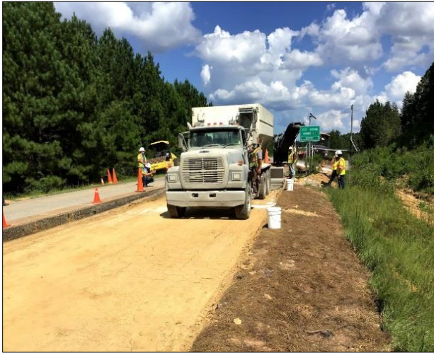
a) Self-unloading for lime application
