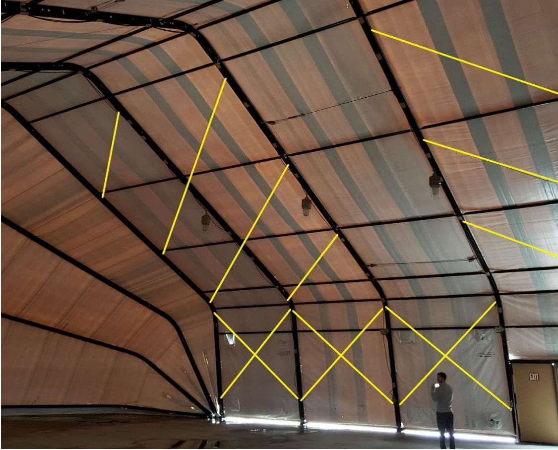
Figure 3.1-13. LAMS wall and roof cable configuration.
