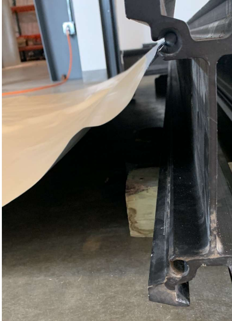
Figure 3.1-15. Kedered fabric attachment to the framing members.
