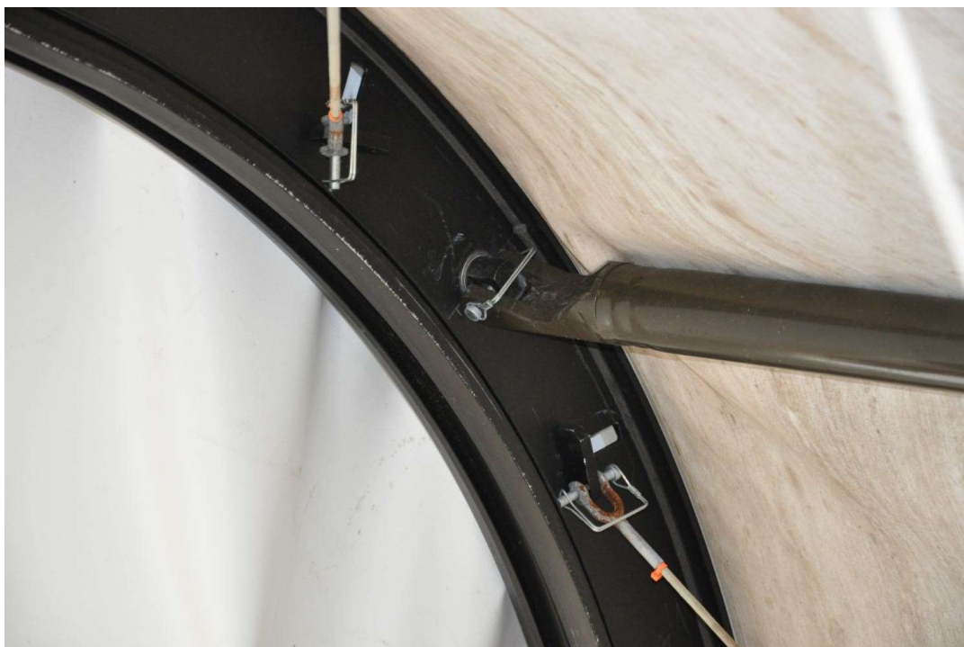
Figure 3.1-10. Purlin, roof, and wall cable connection
