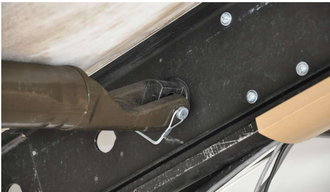
Figure 3.1-9. Purlin connection
