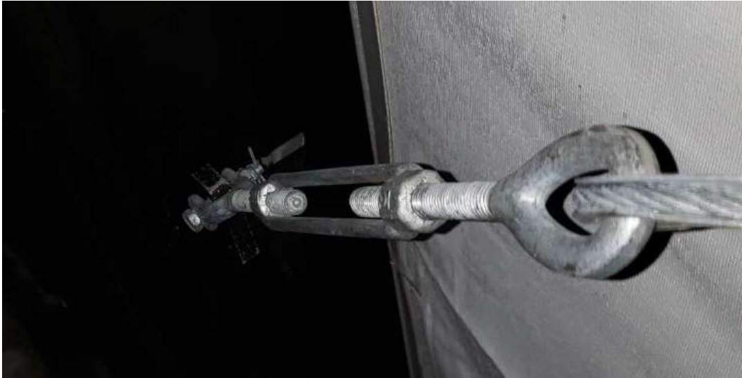
Figure 3.1-11. Wall cable connection to columns.
