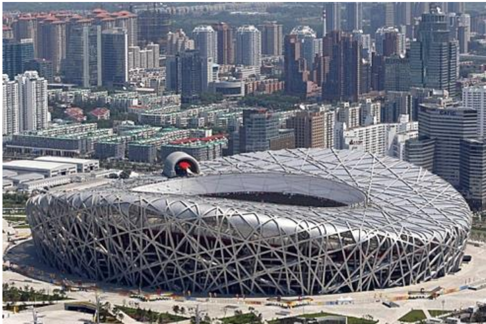
Figure 3.5 Flowing, Bird's Nest Stadium for the 2008 Beijing Olympics (Morari, n.d.).
