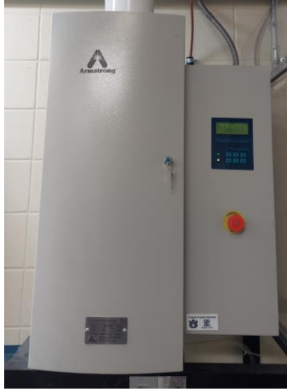
Fig. 12: HumidiClean Series HC-6100 industrial steam humidifier up to 15 kW
