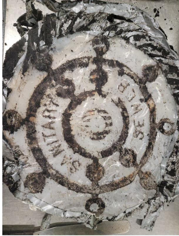
**Figure 16:** Manhole Cover After Scraping
