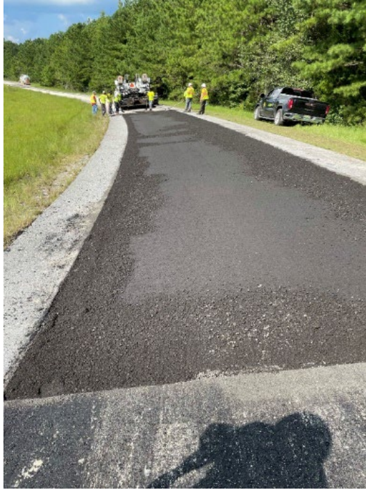
Figure 26 – Foamed Asphalt with Active Filler Section
