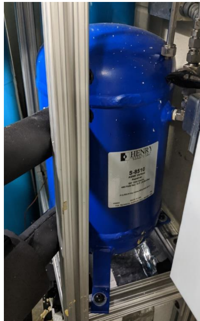
Figure 3.20: Liquid receiver
