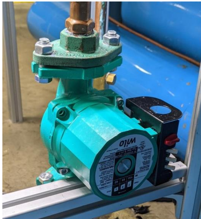
Figure 3.18: Secondary refrigerant centrifugal pump
