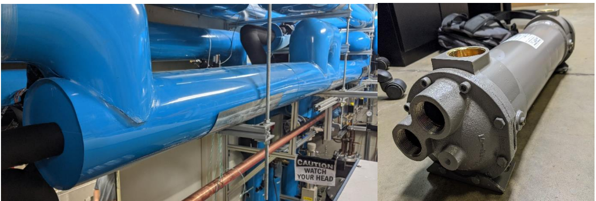
Figure 3.19: Tube-in-tube condenser (left, insulated) and shell-and-tube condenser (right)
