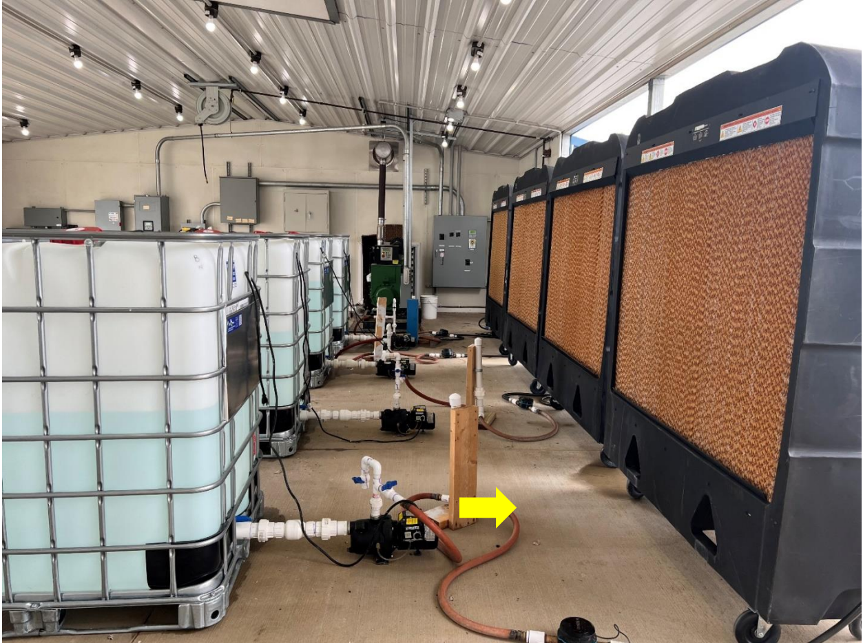
Figure 1: Four portable evaporative cooling systems fitted with new paper pads. Stationary IBC tanks were plumbed into each evaporative system through a pump and water meter. The yellow arrow is pointing at the supply water sampling ball valve.
