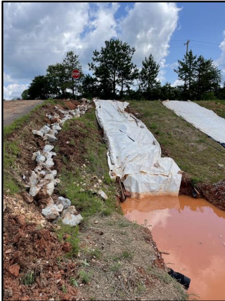
Figure 3-17: Improved Drainage Channel
