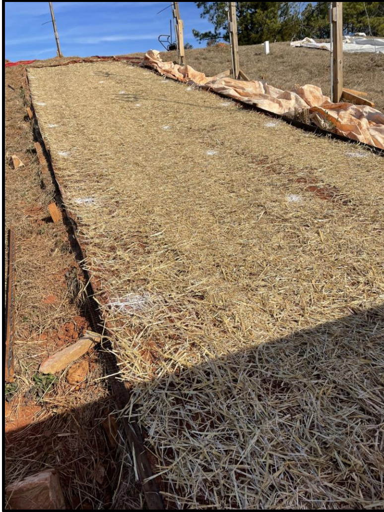
(a) Single-Net Straw Blanket Pinning Figure 3-8: ECP Installation
