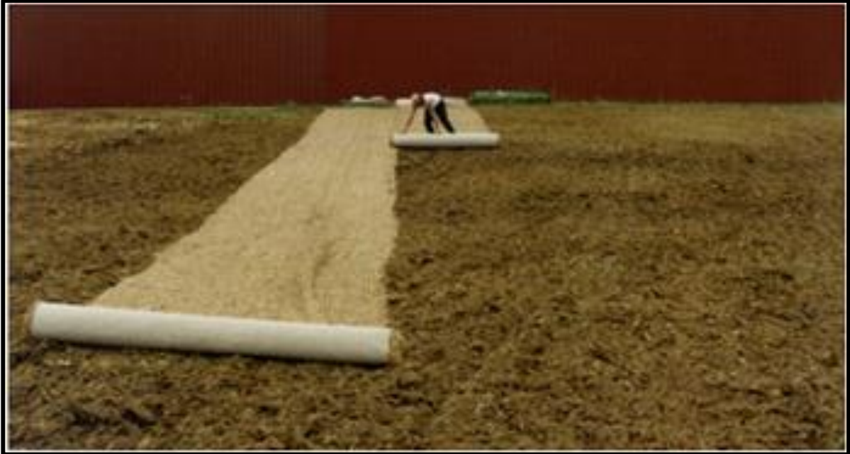
Figure 2-8: Deploy RECP (ECTC 2014).
