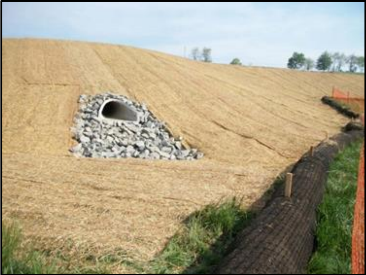
Figure 2-2: Erosion Control Blanket (Granite Seed 2024)
