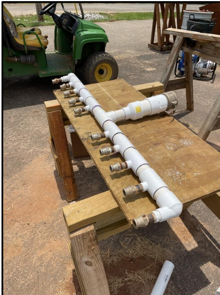
Figure 3-14: Improved Water Supply Manifold
