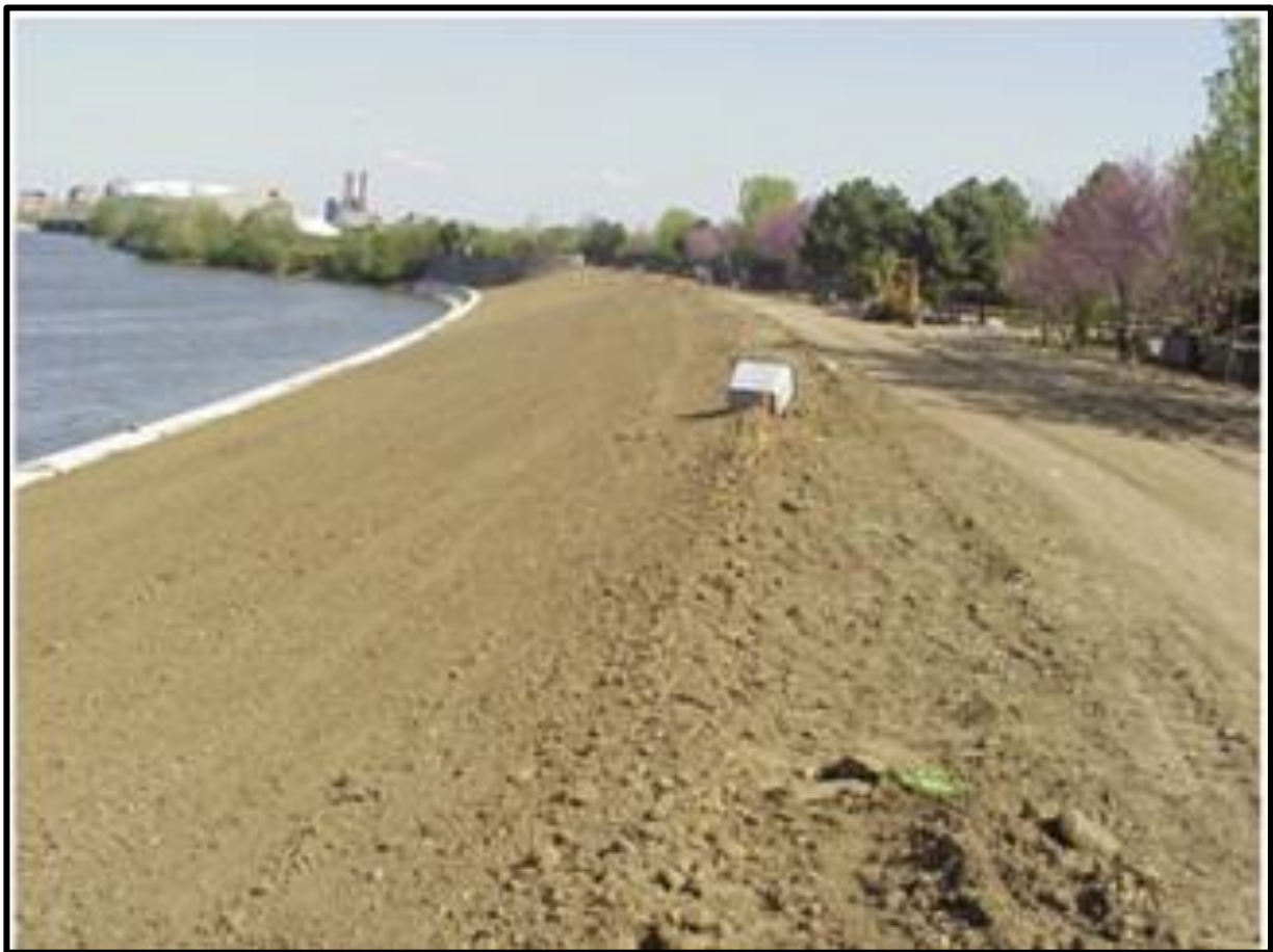
Figure 2-4: Prepared Installation Site (ECTC 2014).
