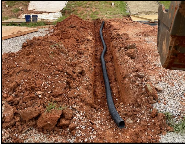
Figure 3-18: Slope Drain Installation
