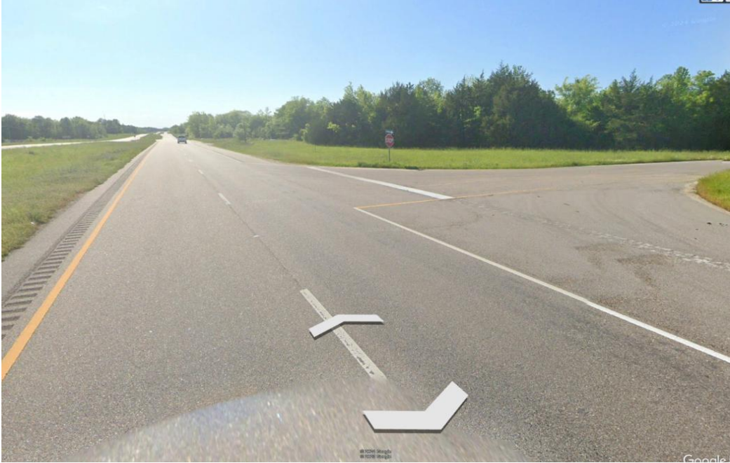
Figure 4.10 Presence of ramp as potential contributor of RL degradation
