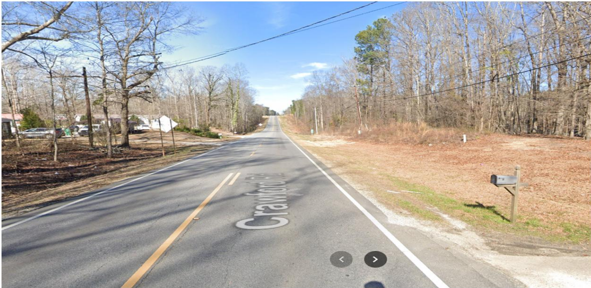
Figure A4 A rural two-lane location with multiple single-vehicle ROR crashes occurring within a 0.5-mile segment with RL of WREL < 250 mcd/m 2 /lux
