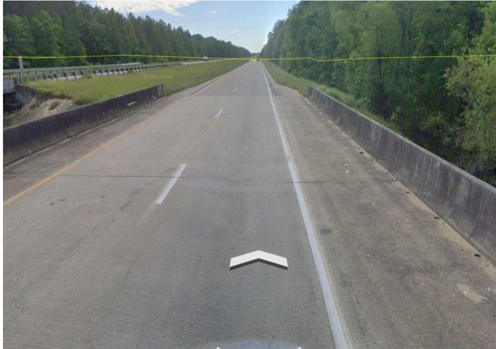
Figure 4.9 Bridge as potential contributor of RL degradation
