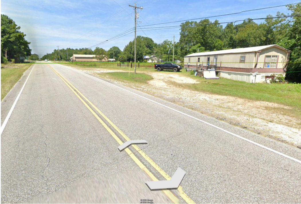
Figure 4.12 Residential driveway as potential contributor of RL degradation
