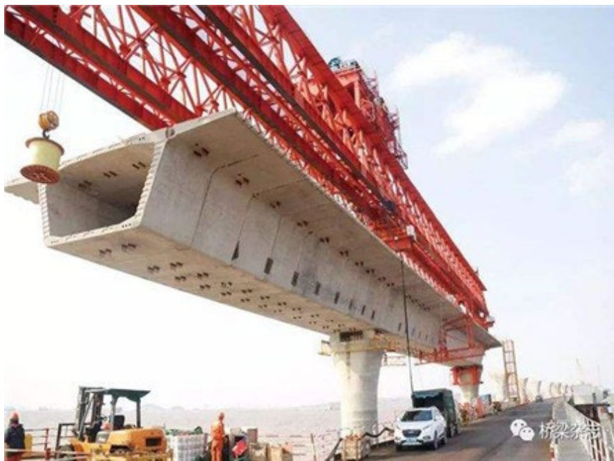
Figure 1-1 Segmental Bridge Structure. Source: Datai Crane (2024)
