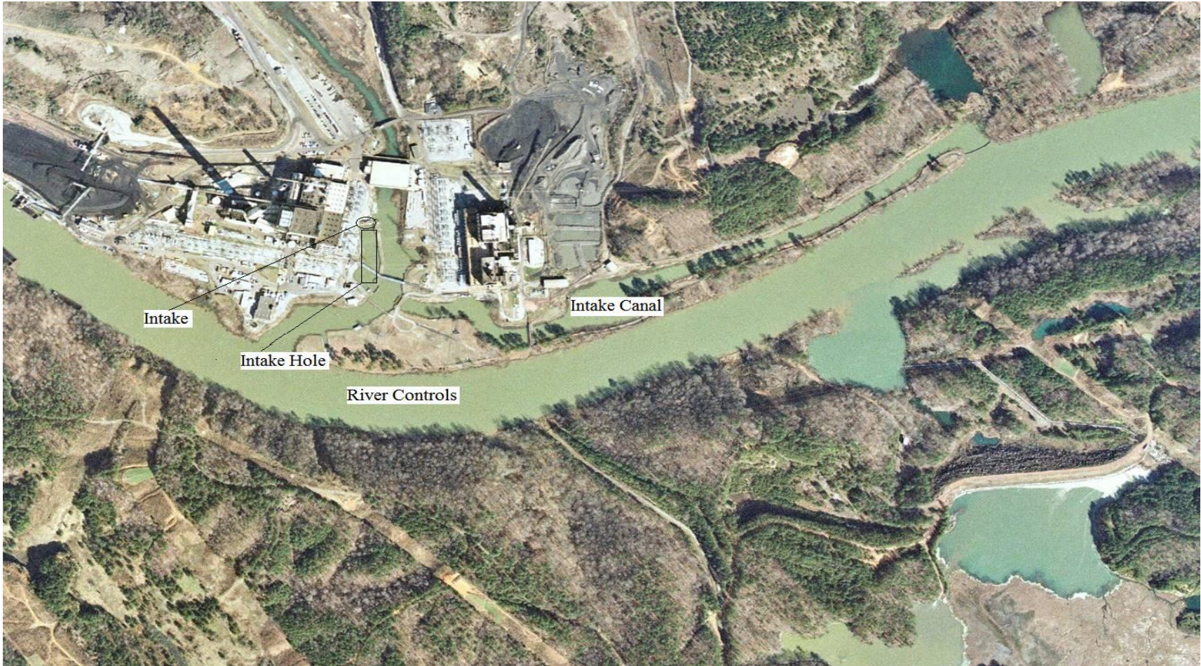
Figure 1. Plant Gorgas intake structures and associated intake canal perpendicular to the Black Warrior River with sample collection areas indicated.
