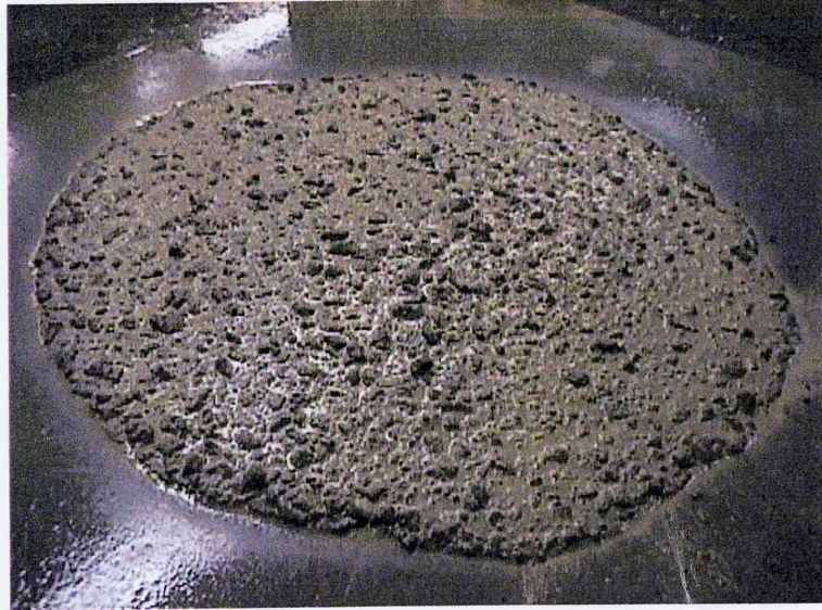
Figure 2-5: Typical visual stability index rating of 1.0 (PCI 2003)
