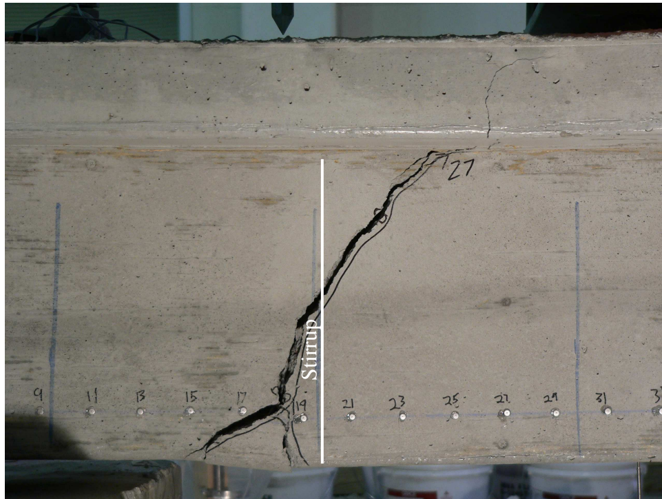
Figure 5-18. Diagonal crack location of specimen SCC-M-W
