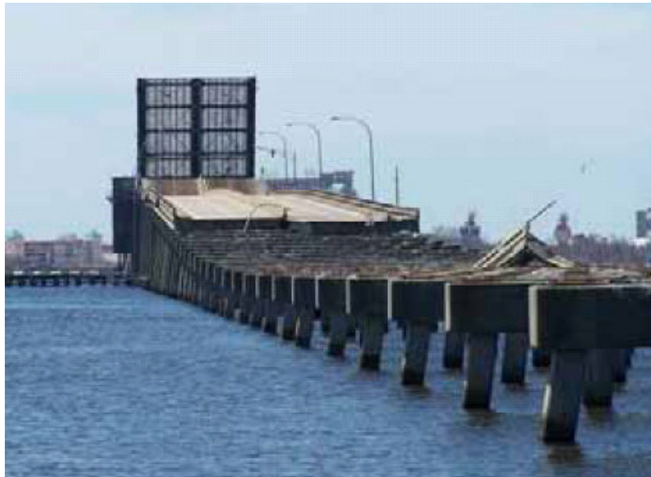
Fig. 2.24 Photo looking west toward Biloxi of Hurricane Katrina damage to U.S. 90 Bridge over Biloxi Bay (Douglass et al, 2006).
