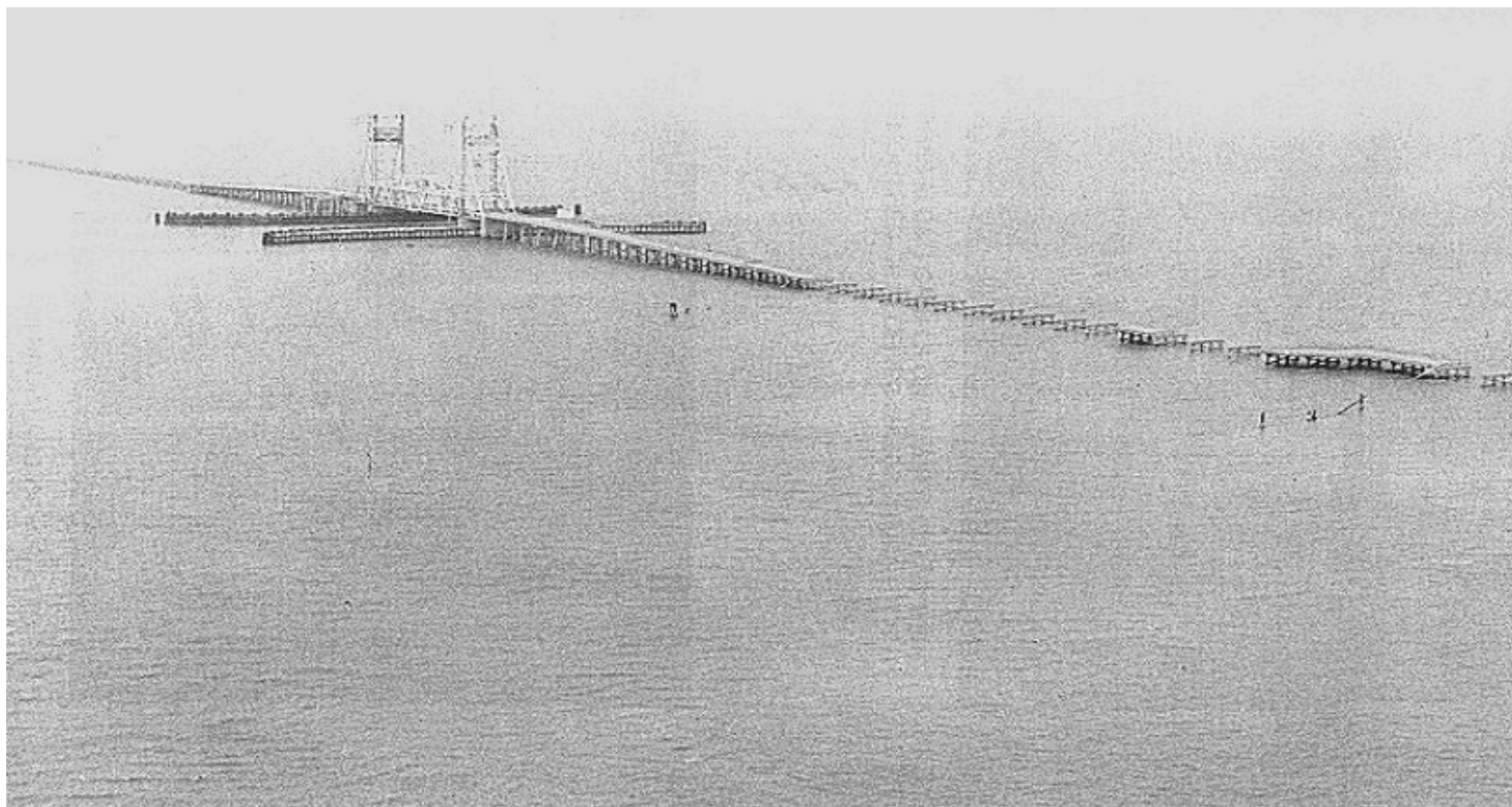
Fig. 2.38 Aerial View of Dauphin Island Bridge Showing Damage Near Lift Span at Intersection of Gulf Intracoastal Waterway Channel (US Army, 1981).
