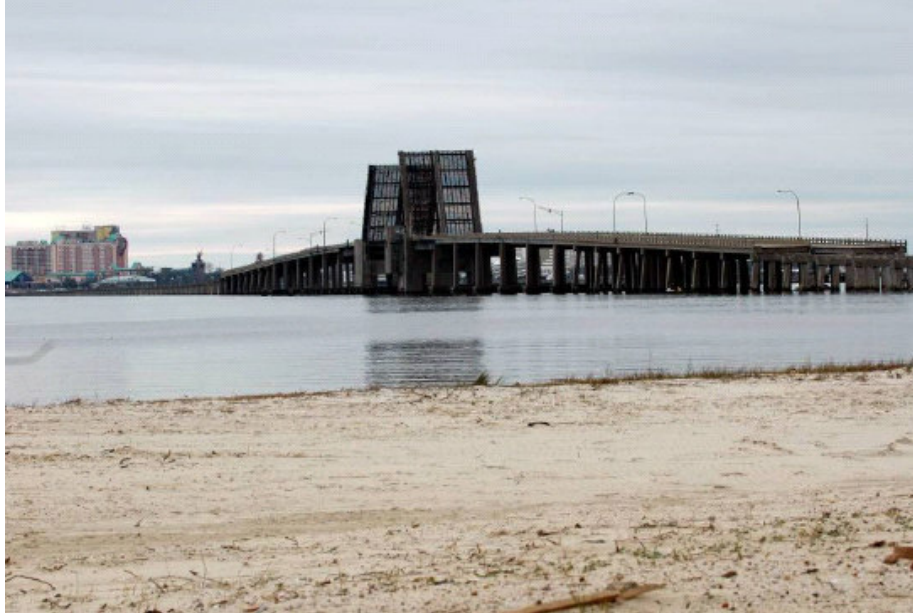
Fig. 4.13. Photograph of U.S. 90 bridge over Biloxi Bay showing high spans which were not knocked off pile cap bents during Hurricane Katrina (This photo was taken 2/19/06 looking west from Ocean Springs.)
