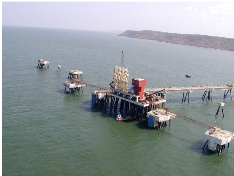
Figure 3.18 Typical jetty head (courtesy Kier) (McConnell et al., 2004)
