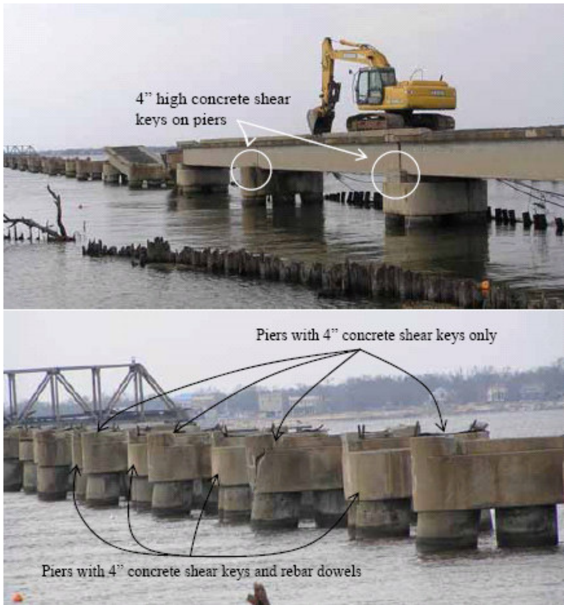
Fig. 3.42 CSX railroad bridge at Bay St. Louis, MS with remaining spans (top) and the supporting piers (bottom) (NIST, 2006).
