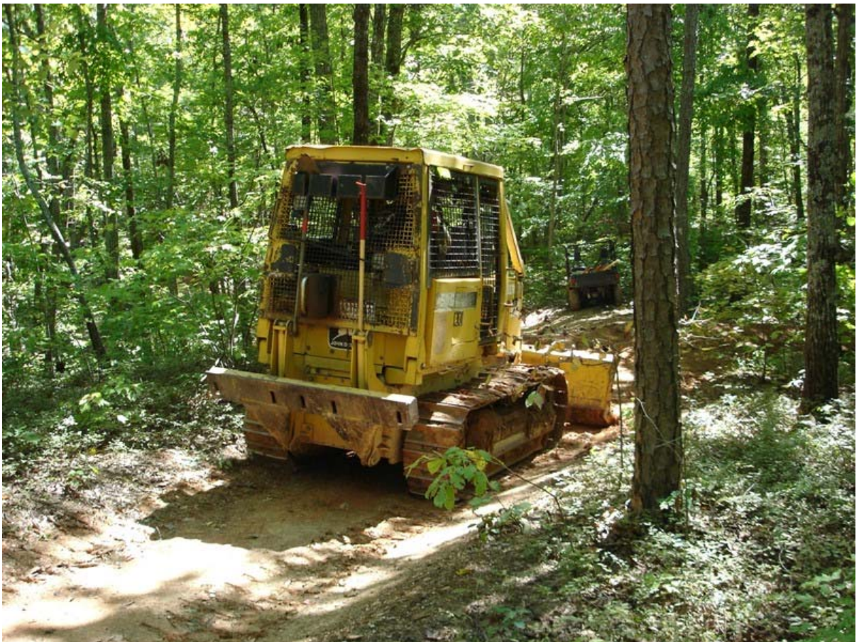
Figure 3.3 -- US Forest Service bull dozer performing maintenance.
