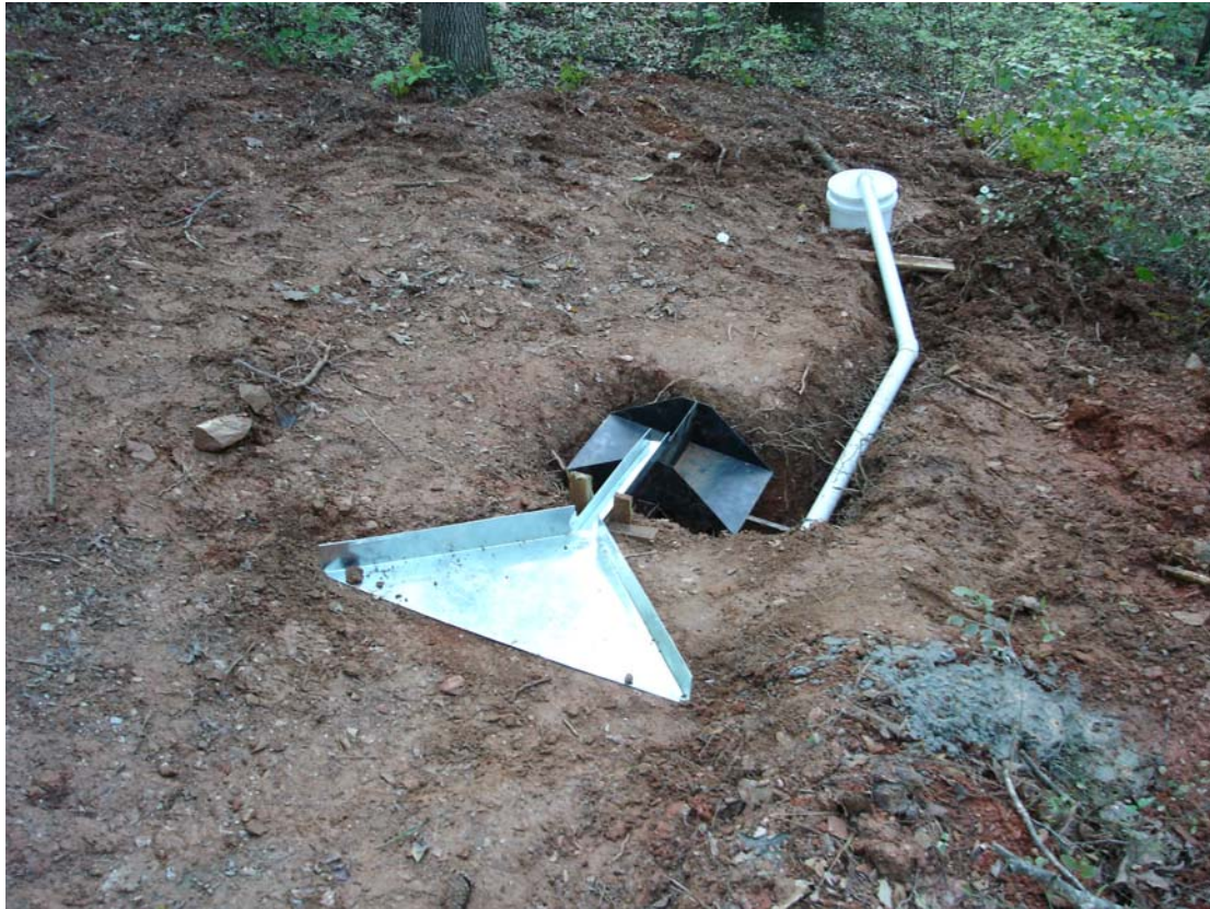
Figure 3.4 -- Tipping bucket sampler during installation on the mild slope.
