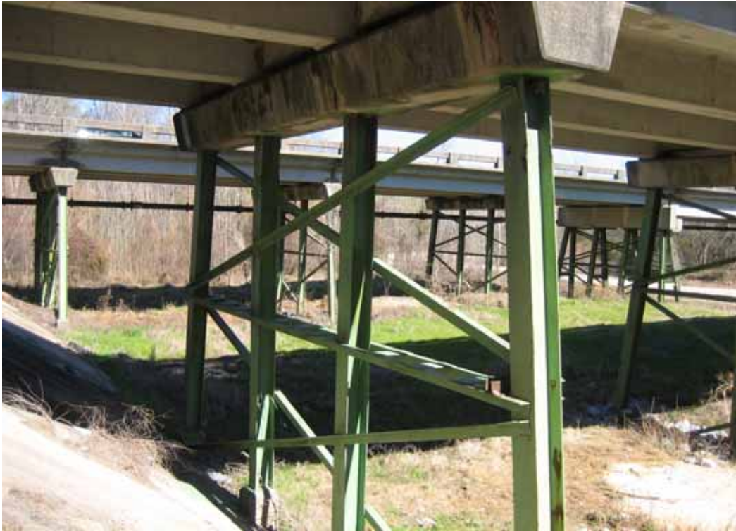
Figure 2.1 Typical Bridge Bent Configuration
