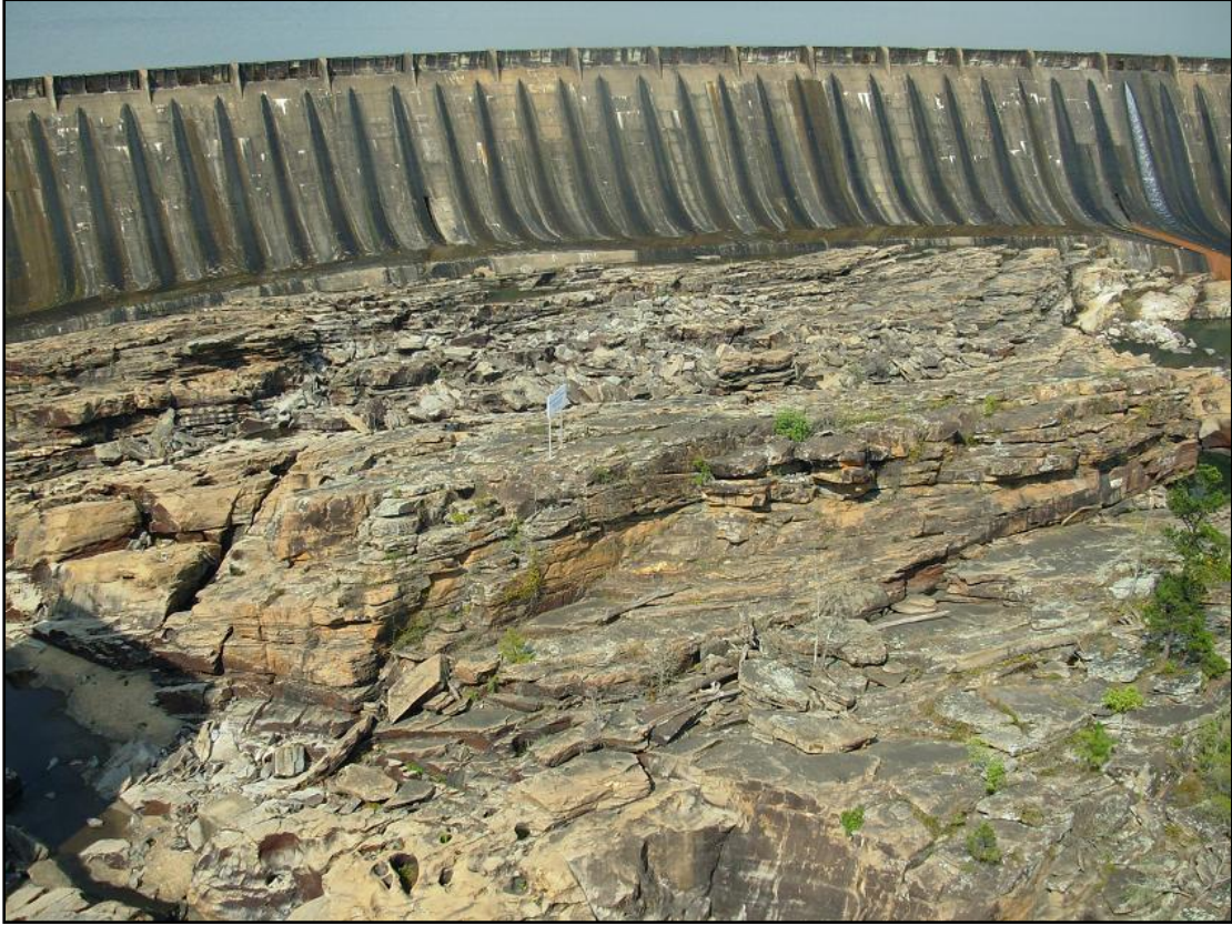
Figure 7. Pavement exposure of Farmville Metagranite at base of Thurlow dam looking north. Note the shallow dip of the unit toward the north.
