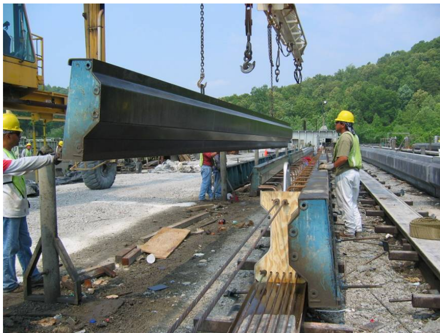
Figure 3-11: Placement of Side Forms
