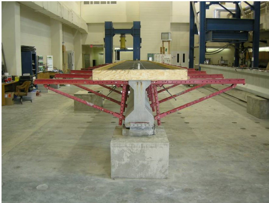
Figure 3-24: Bridge Overhang Brackets and Plywood Formwork
