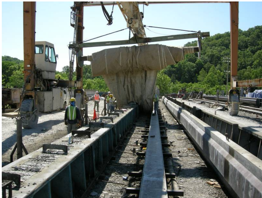
Figure 3-20: Placement of Curing Blankets
