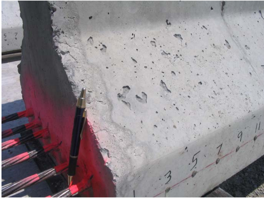
Figure 3-22: Formed Surface of STD-M Girder
