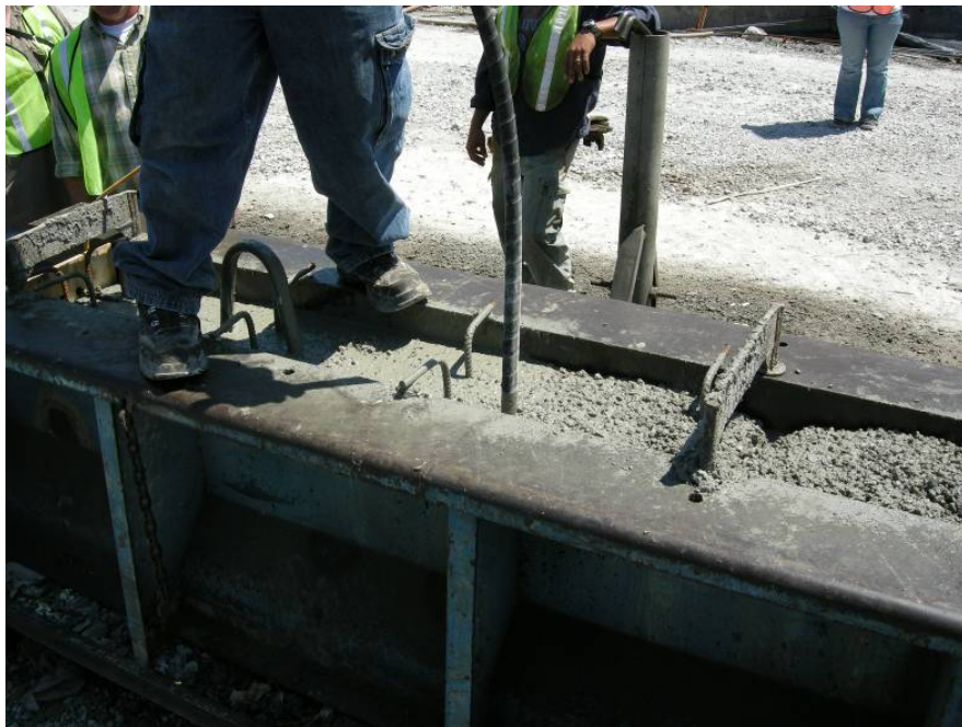
Figure 3-12: Internal Vibration of Conventional Concrete
