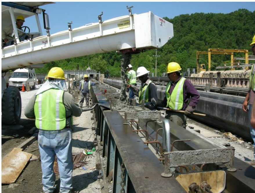
Figure 3-14: Placement of SCC from Concrete Delivery Vehicle at East-End Discharge Point
