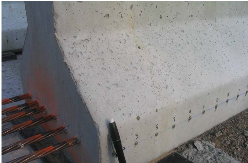
Figure 3-23: Formed Surface of SCC-HS Girder
