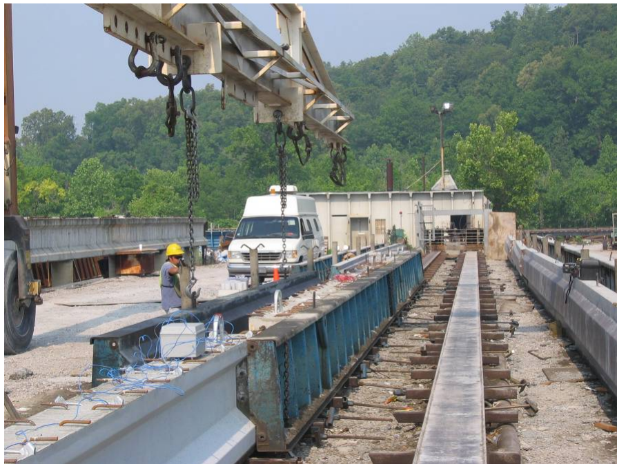
Figure 4-4: Side Form Removal
