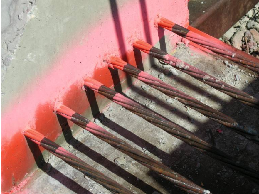
Figure 5-2: Strand Painted to Provide Benchmarks for Draw-In Measurements
