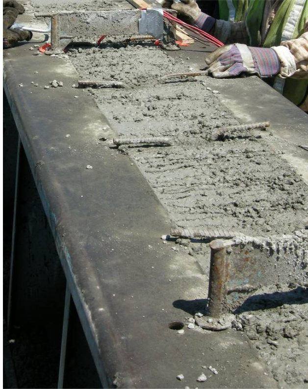
Figure 3-19: Raked Top Surface of Girder STD-M-1
