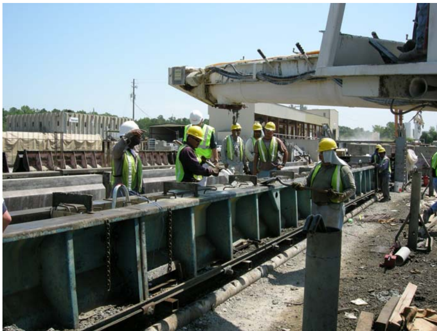
Figure 3-17: Girder Casting Completion at West-End Discharge Point
