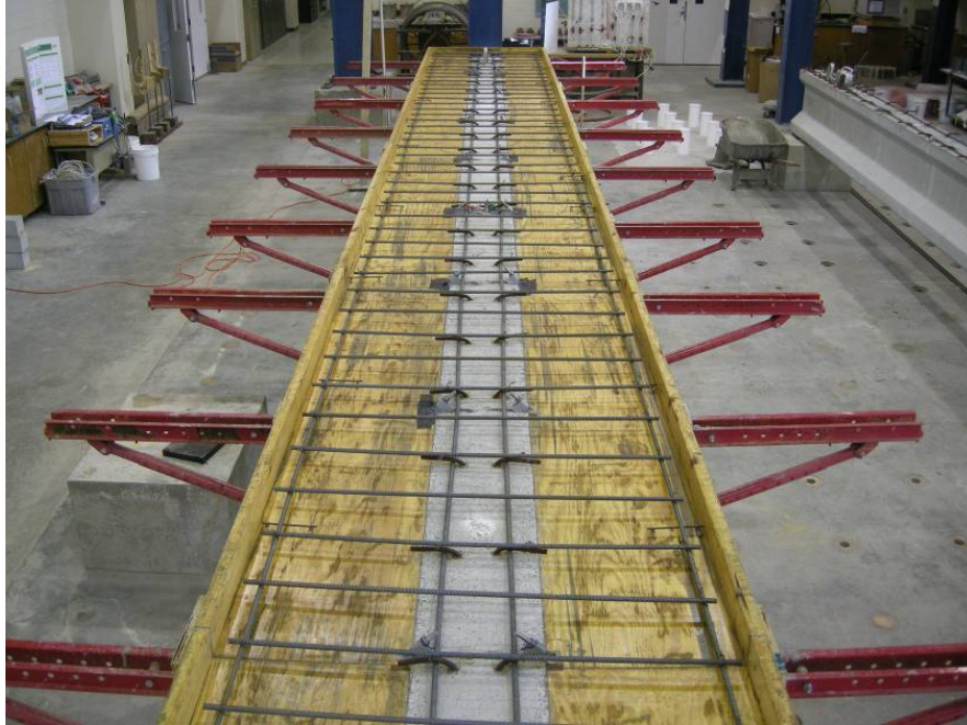
Figure 3-25: Slab Reinforcing Steel
