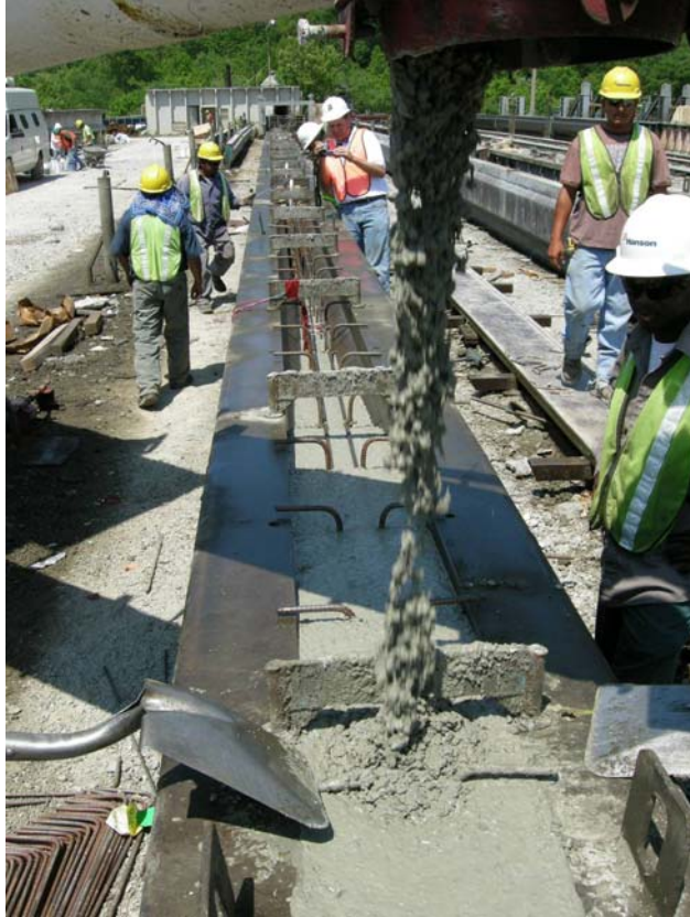
Figure 3-16: Concrete Level Prior to Relocation to West-End Discharge Point
