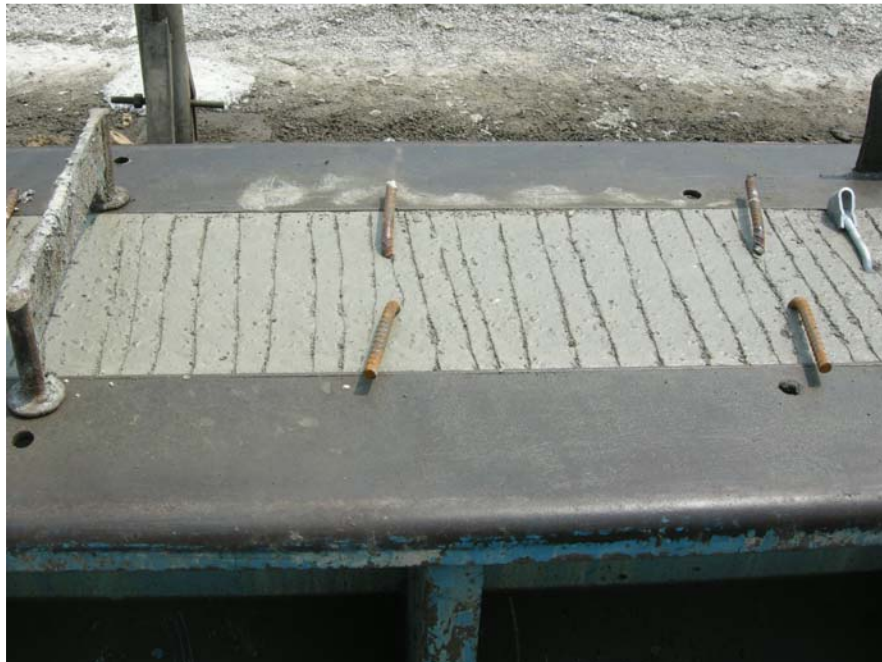
Figure 3-18: Raked Top Surface of Girder SCC-MS-1
