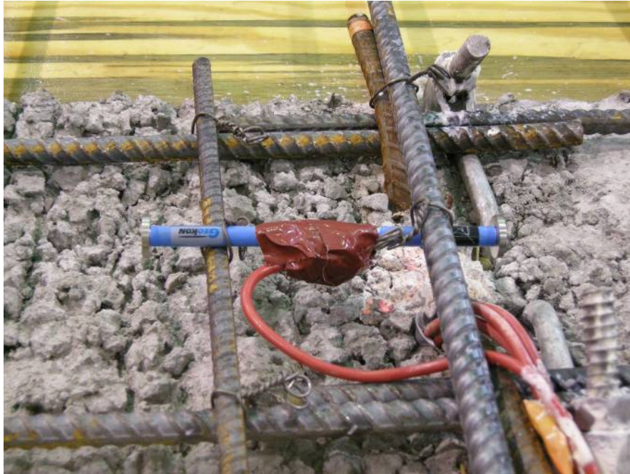
Figure 6-32: Typical Conventional-Slump Concrete Girder Surface
