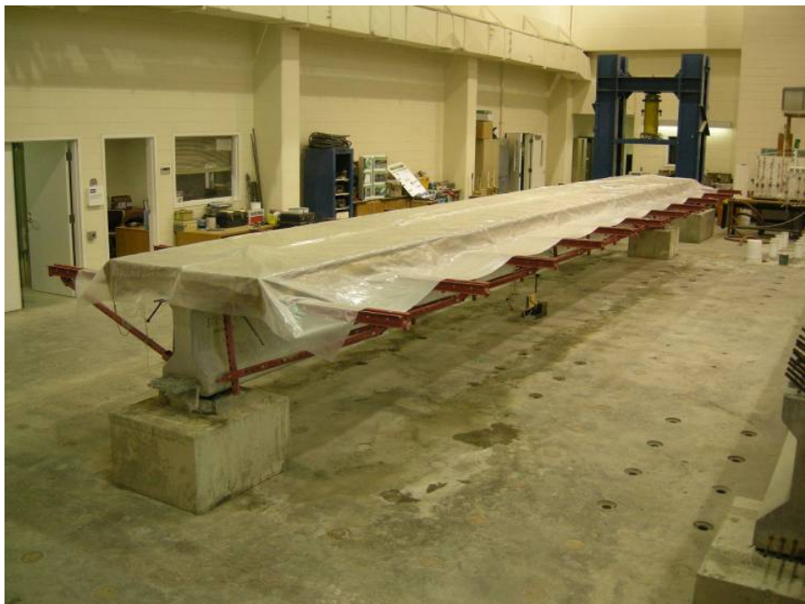
Figure 3-27: Application of Wet Burlap and Plastic
