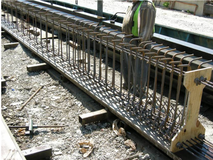
Figure 3-10: Mild Steel Reinforcement
