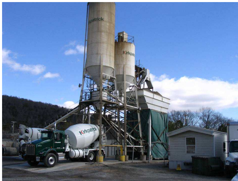
Figure 5.14: Loading of concrete truck with raw materials
