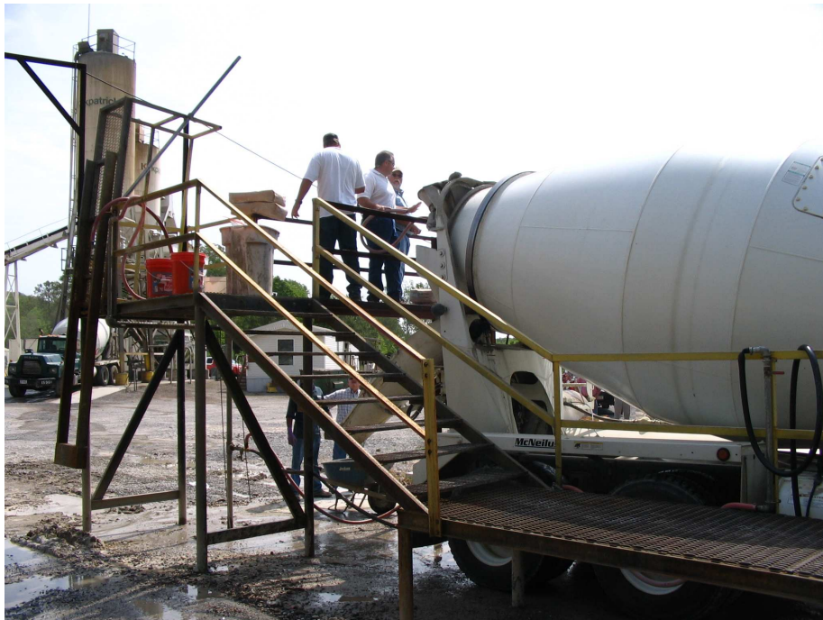
Figure 5.16: Addition of HRWR admixture and limestone powder into concrete truck
