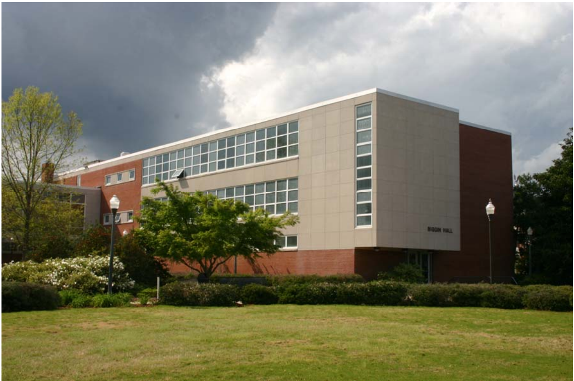
Figure 28: Exterior Picture of Biggin Hall
