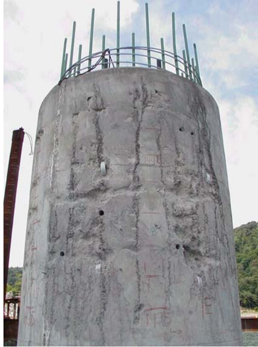
Figure 3.25 – Example 2 of Bleed Channels and Surface Streaks due to Bleed Water Traveling along the Casing (photograph courtesy of Dr. Dan Brown)
