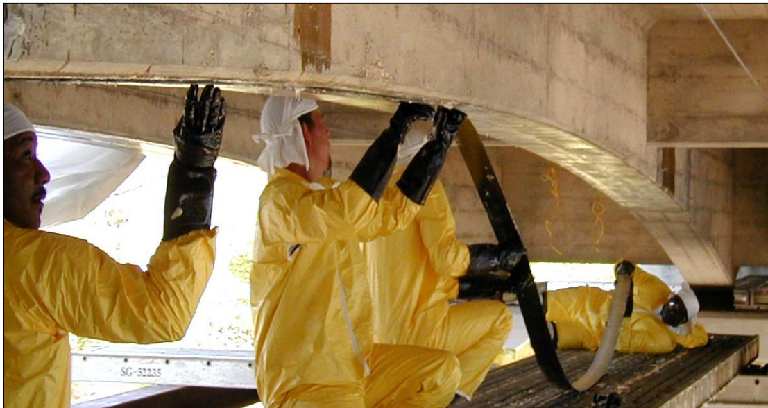
Figure 4.10: Application of the Composite Strip to a Girder
