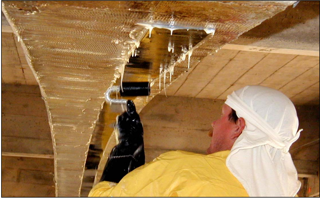
Figure 4.11: Seating an FRP Strip Using a J-roller
