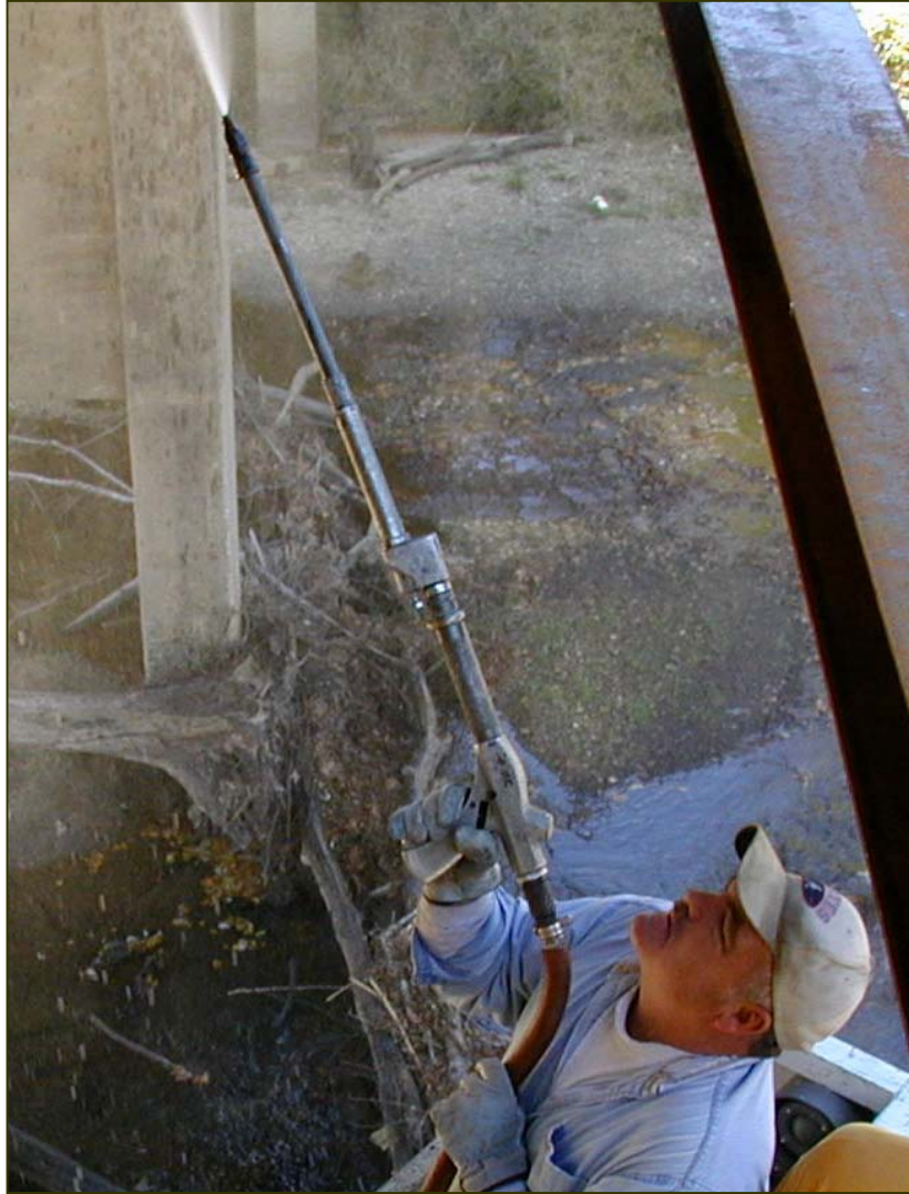
Figure 4.3: Hydroblasting the War Memorial Bridge
