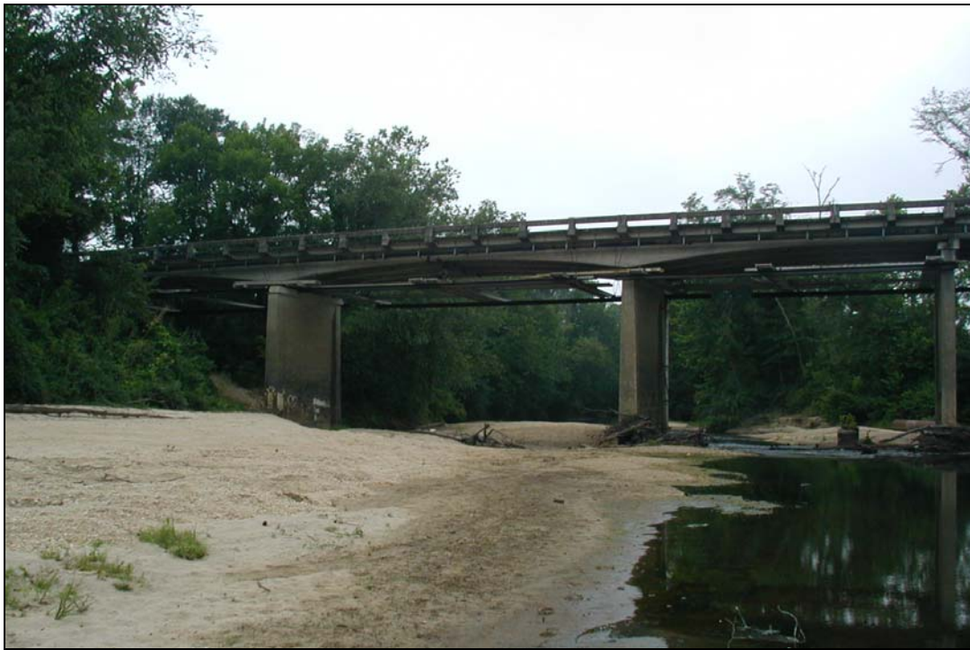
Figure 3.1: Continuous Span Portion of the War Memorial Bridge
