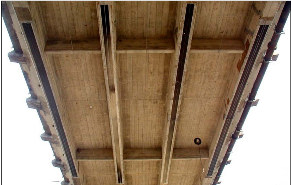
Figure 4.12: Completed Installation of Composite to Center Span Girders
