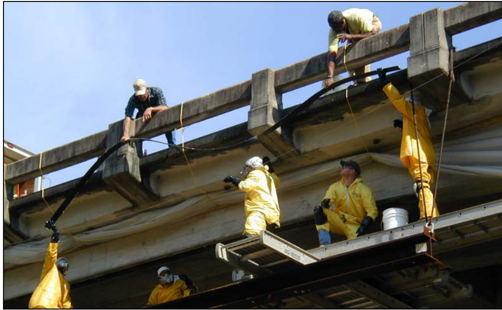
Figure 4.9: Transfer of Epoxy-Coated Strip from Bridge Deck to Scaffolding
