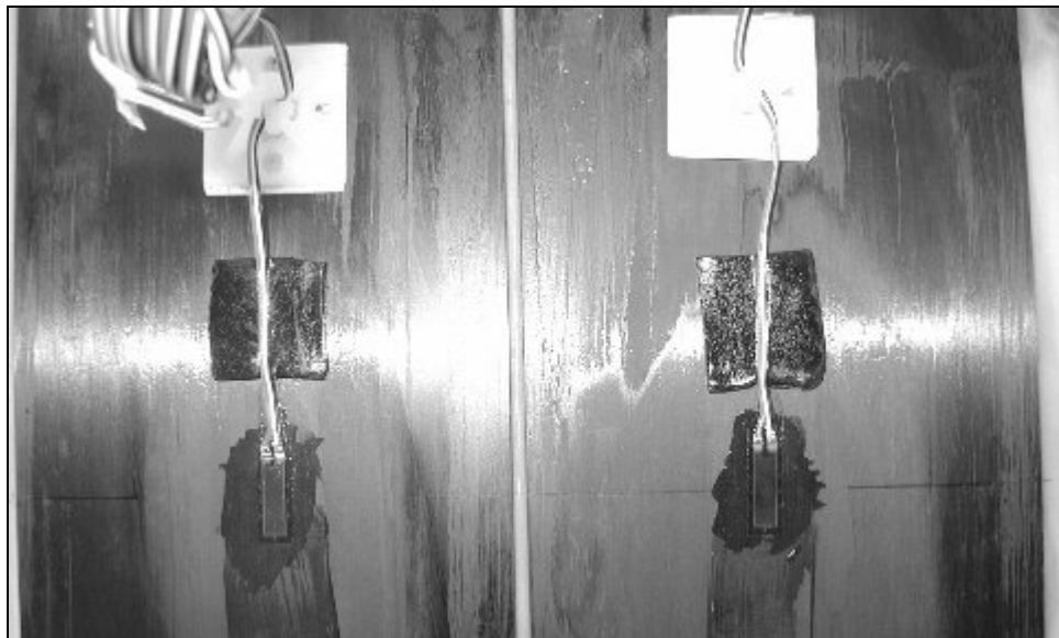
Figure 5.5: Typical Strain Gauge Installation to FRP Surface for Interior Girder
