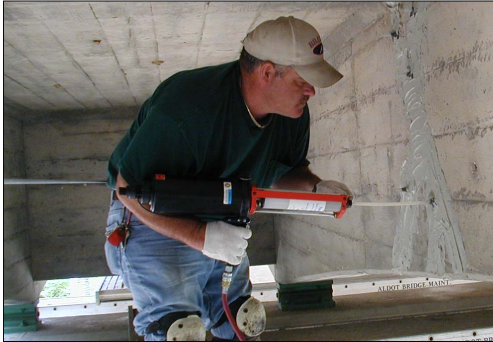
Figure 4.4: Crack Injection of the War Memorial Bridge
