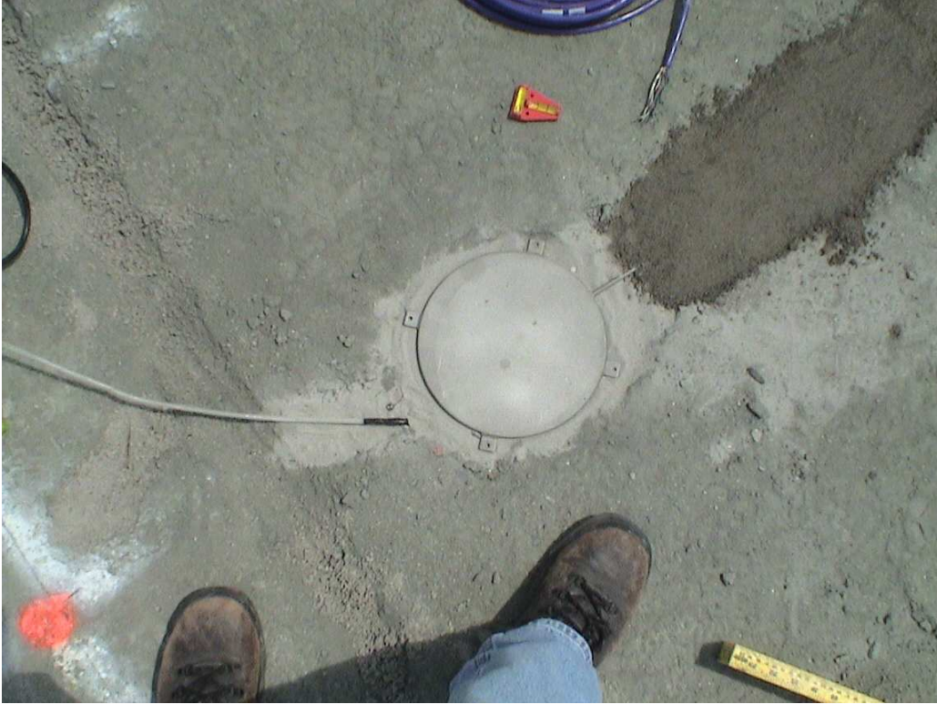
Figure 3.8 The Base Pressure Cell on Top of Base Layer.
