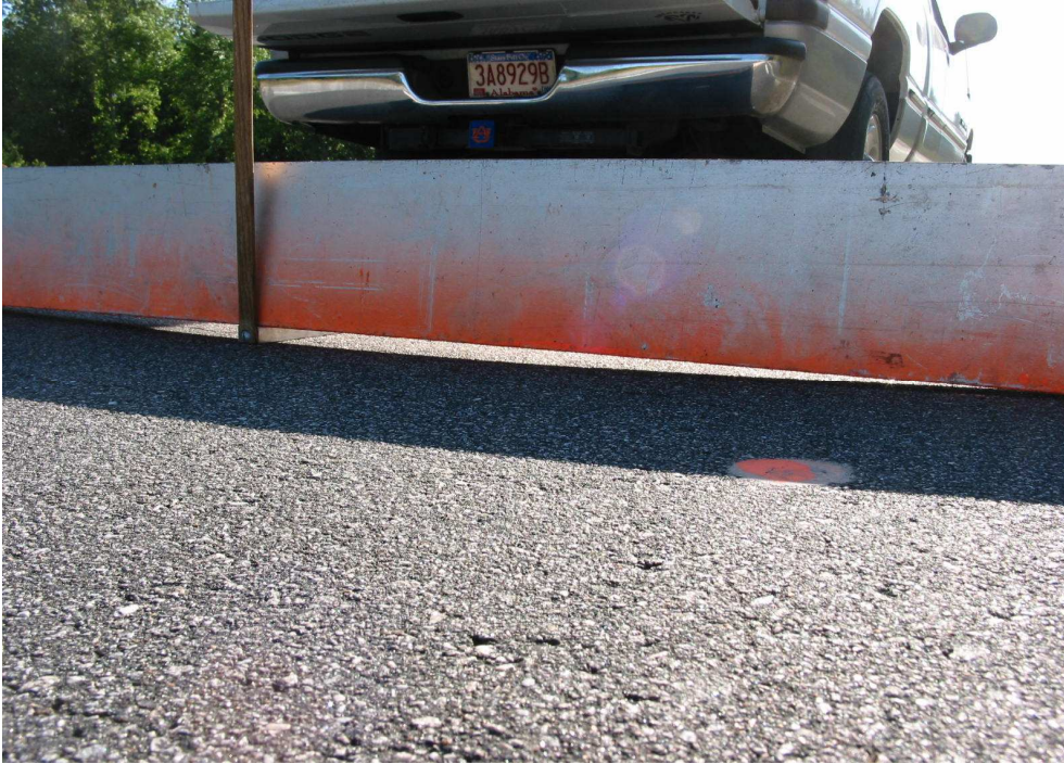
Figure 3.19 Six Foot Straight Edge Transverse Profile Measurement.
