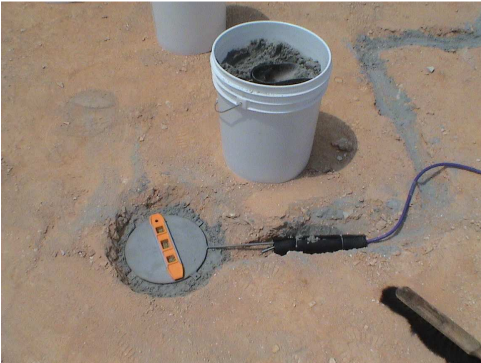
Figure 3.7 Subgrade Earth Pressure Cell Placed on the Top of Subgrade.
