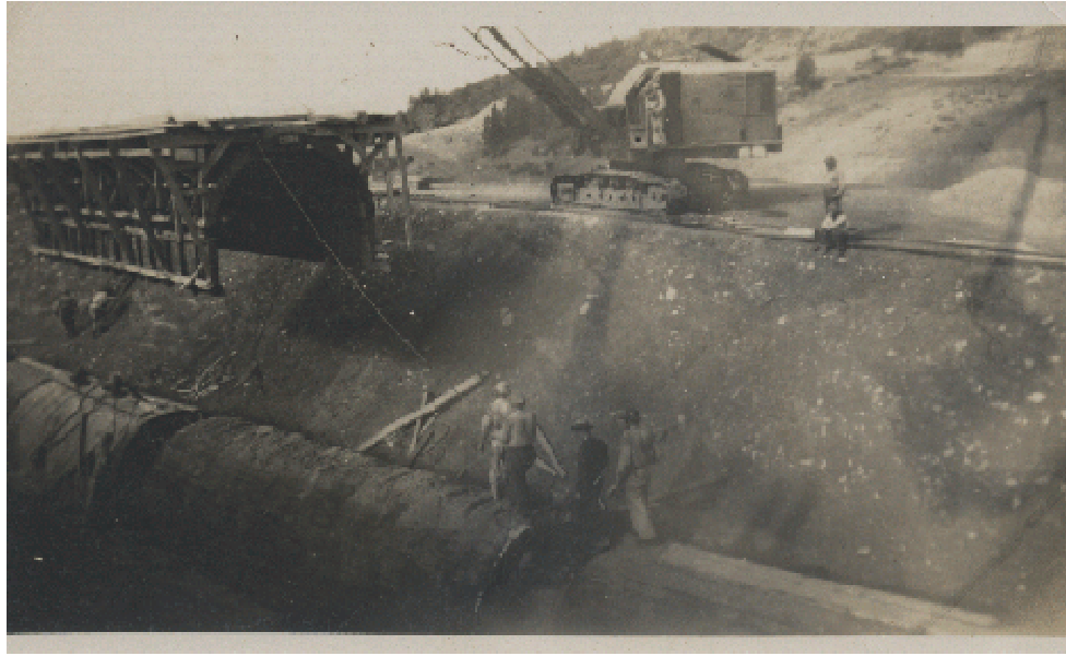
Figure 33: Laying outlet line. Note how much work is done by hand
