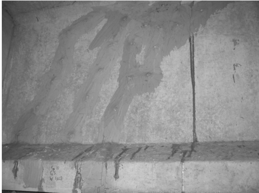
Figure 2-6: Epoxy-Injected Cracks
