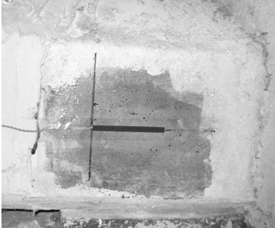
Figure 4-1: Typical Strain Gage Before Being Protected
