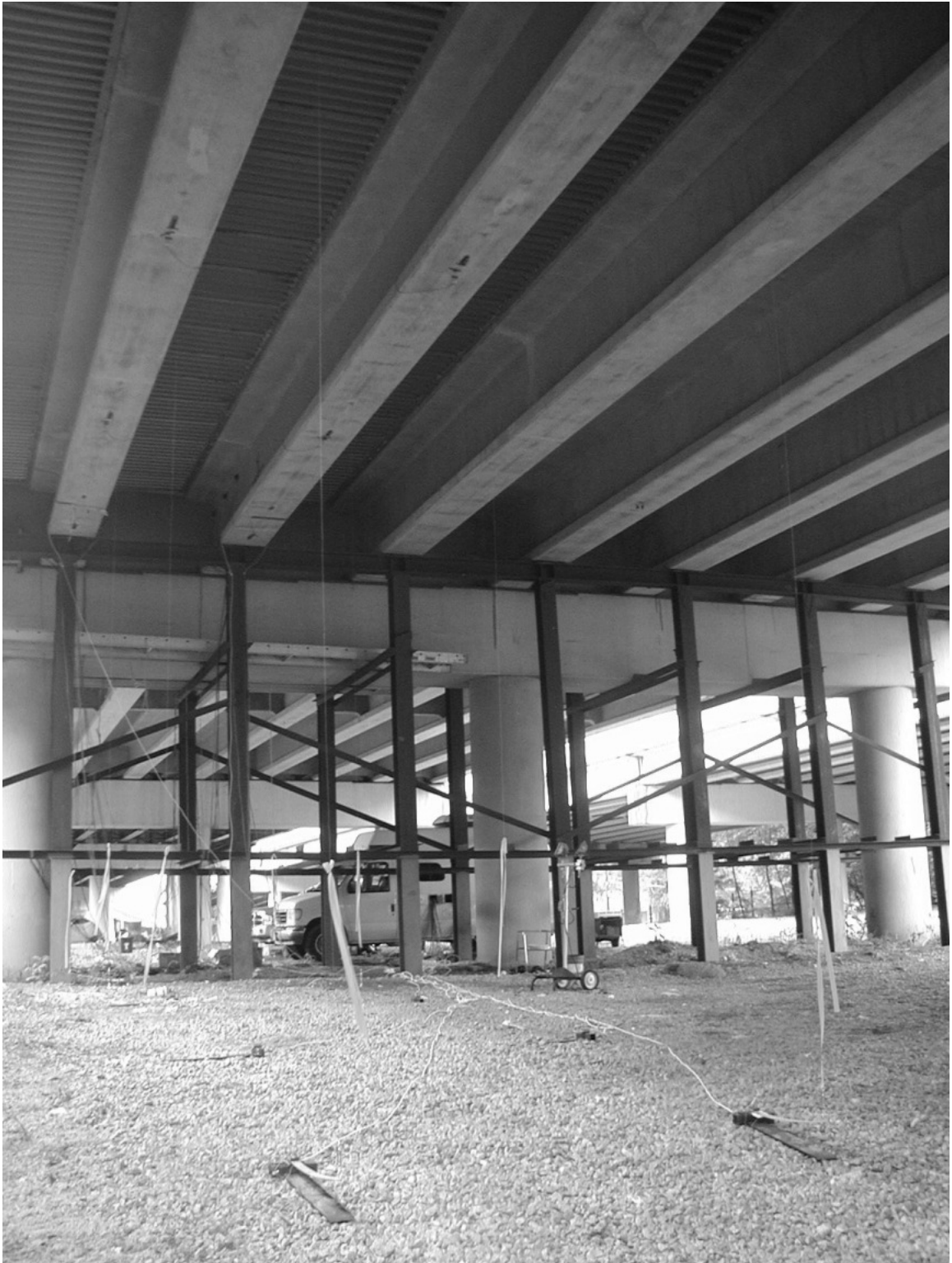
Figure 4-13: Deflectometers During Test
