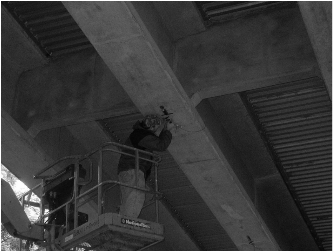
Figure 4-11: Deflectometer Bracket Being Attached to the Underside of Girder 8
