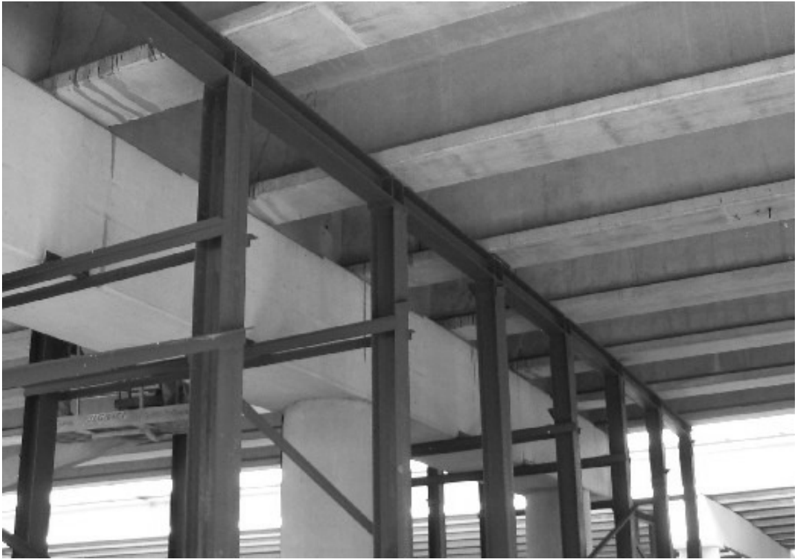
Figure 3-2: Bent 11 North View
