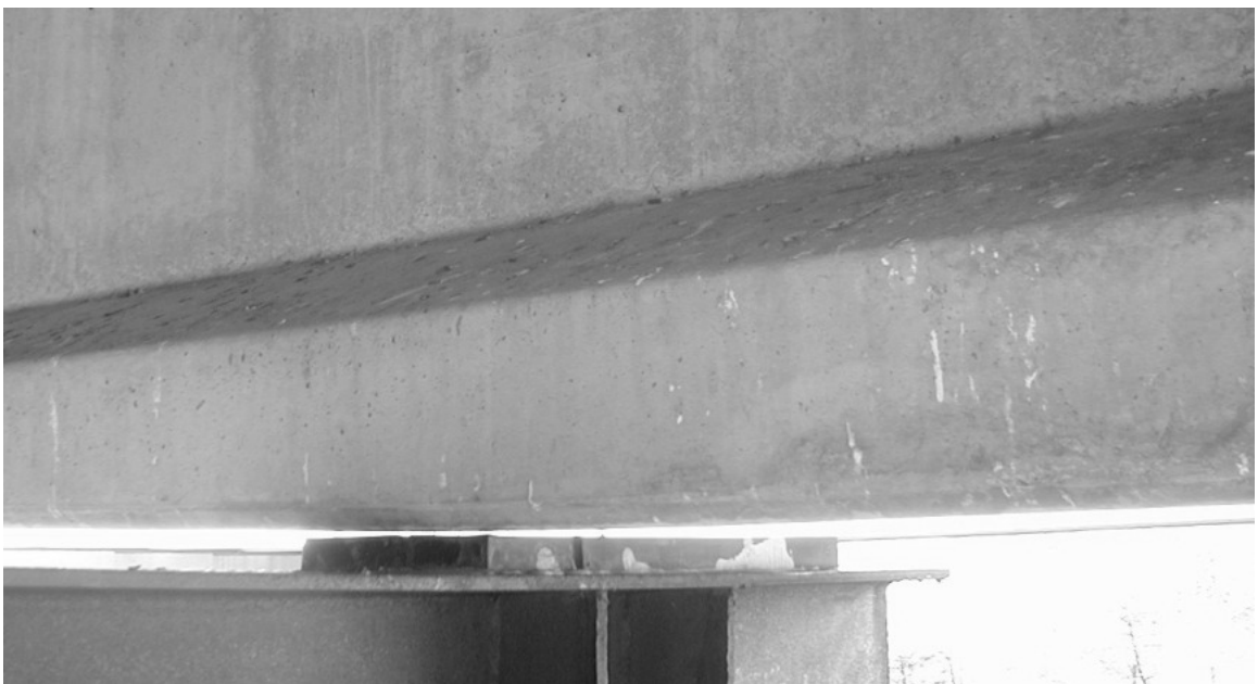
Figure 3-3: Proper Space Between Girder and False Support
