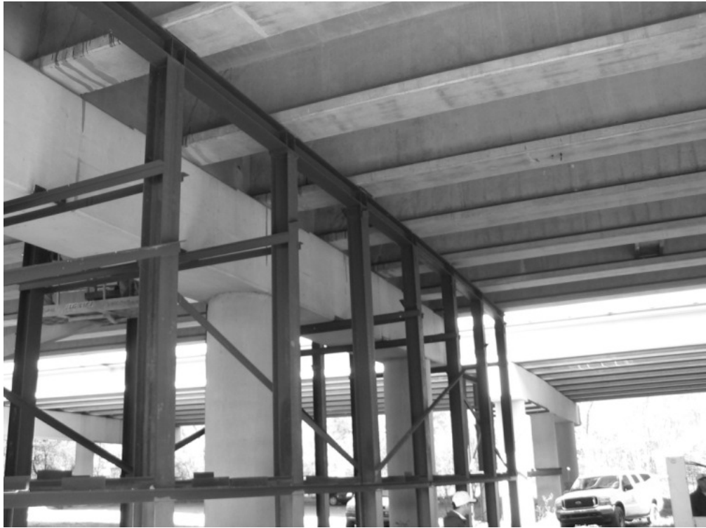
Figure 2-4: False Supports
