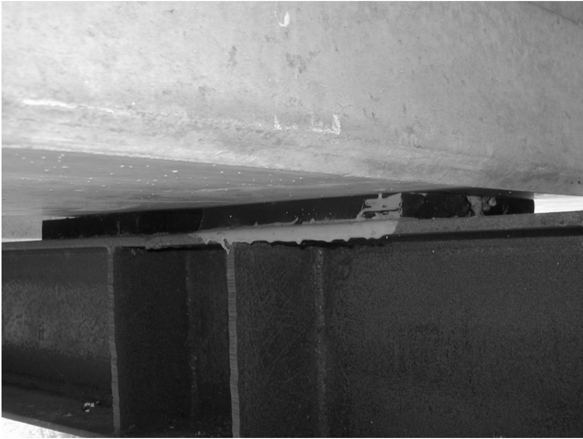
Figure 3-4: Girder Resting on Bearing Pad
