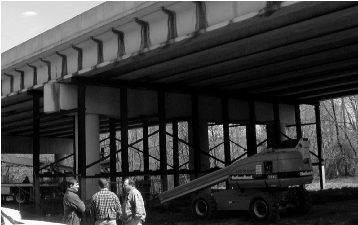
Figure 3-1: Bent 11 South View
