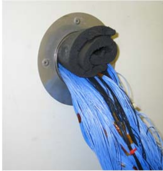
Figure 19 – Wires Passing Through the Access Hole
