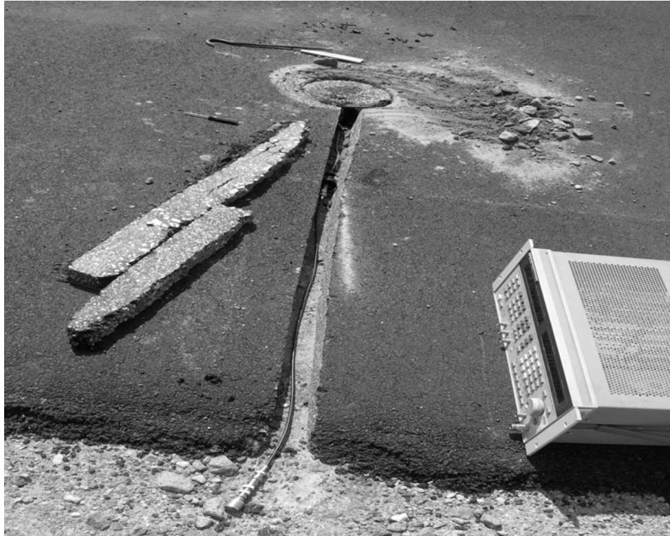
Figure 5 —Asphalt hole and trench at the NCAT test track
