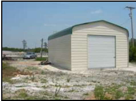
(a) Testing Facility Structure
