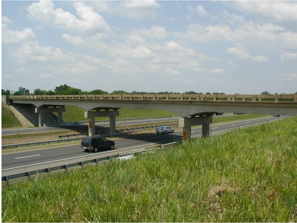
Figure 3-2: Picture of the Letohatchee Bridge
