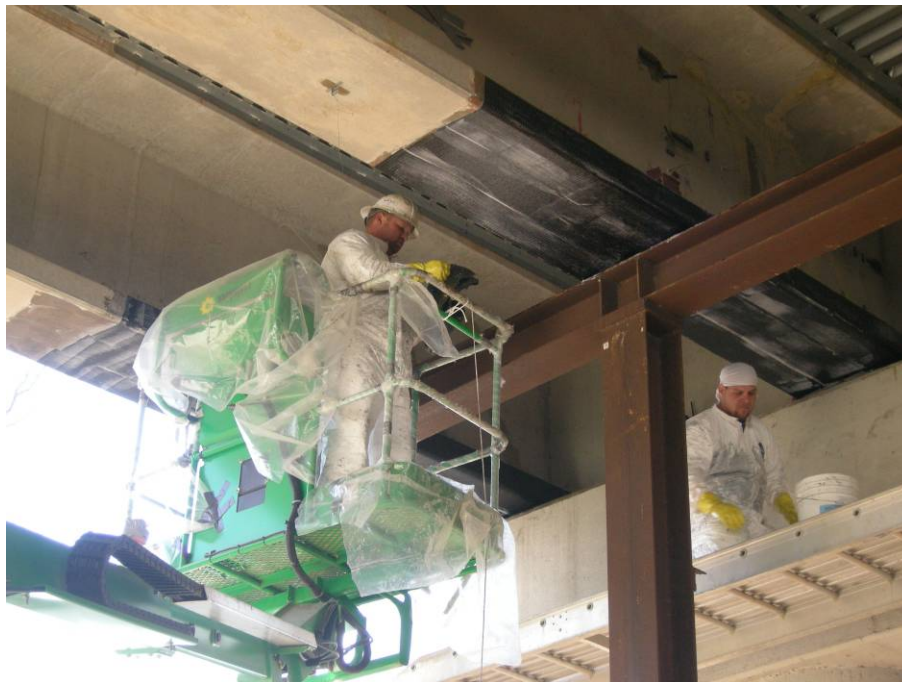
Figure 2-5: Completed Installation of a Wet-Layup EB System
