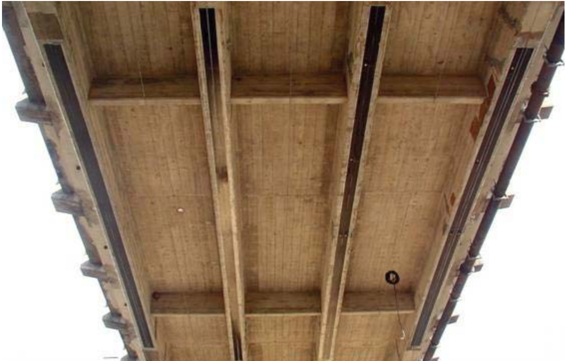
Figure 2-8: Completed Installation of a Precured System (Carmichael and Barnes 2005)
