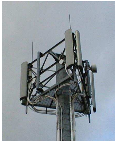
Figure 1.5: Sectorised antenna for Base stations.
