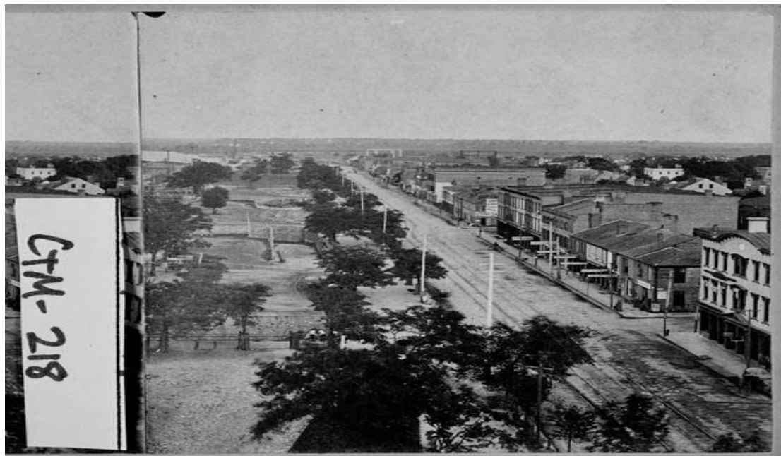
Figure 2: Savannah, 1878. View along Bay Street.; This is a stereograph;The stereograph was taken by Havens, which was located at 141-143 Broughton Street, Savannah, Georgia, at the time the stereograph was made. Courtesy of the Georgia Archives. 32
