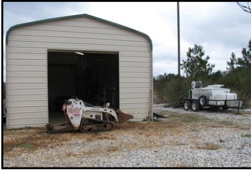
(a) Testing Facility Building
