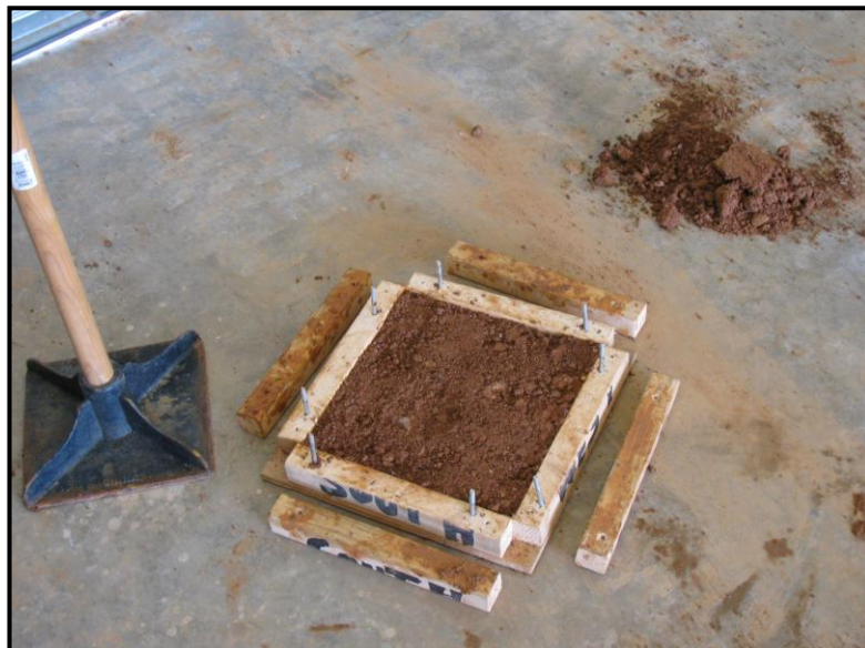
Figure 3.10 Mold used to Determine Required Compaction Rate with Hand-Tamp.
