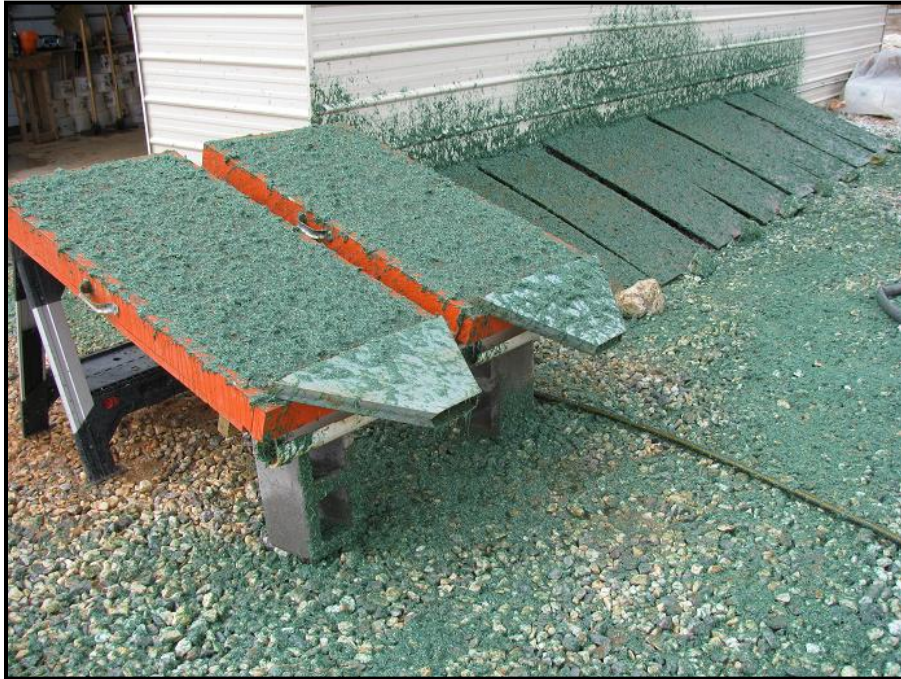
Post-Application of HydroStraw® BFM (a)
