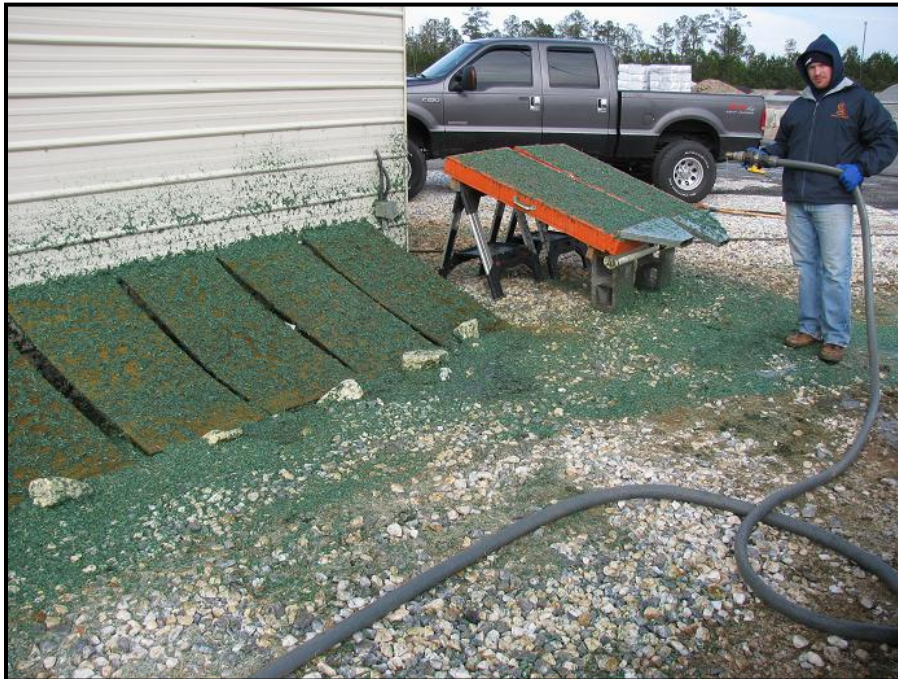
Post-Application of GeoSkin® (a)
