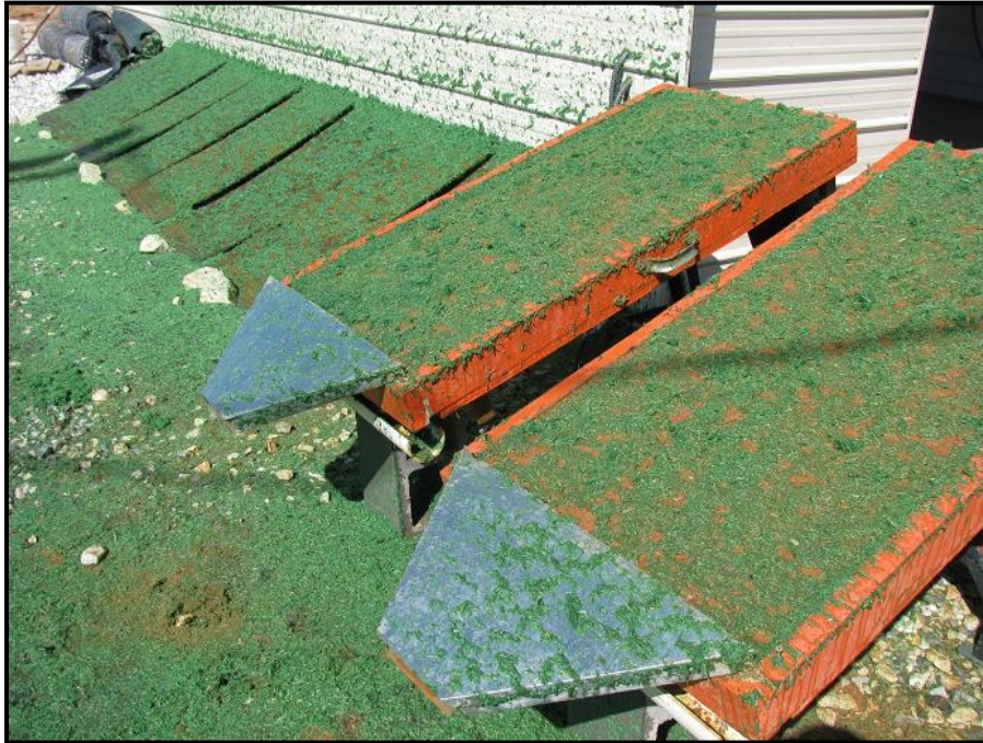
Post-Application of Excel® Fibermulch II (a)
