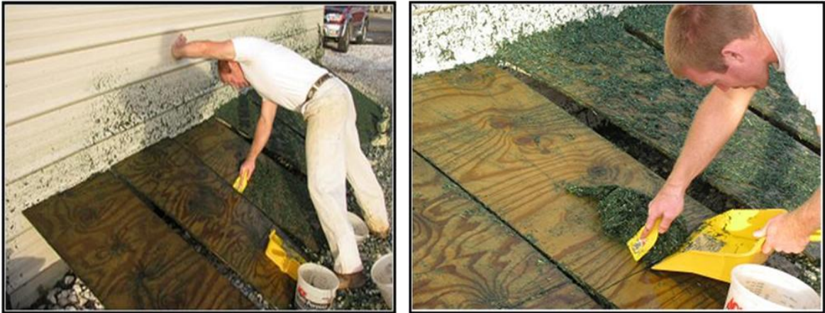
Figure 3.28 Post Application—Scraping Boards into Bucket for Weighing.
