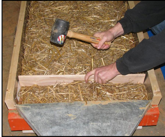
Figure 3.20 Crimping Straw.
