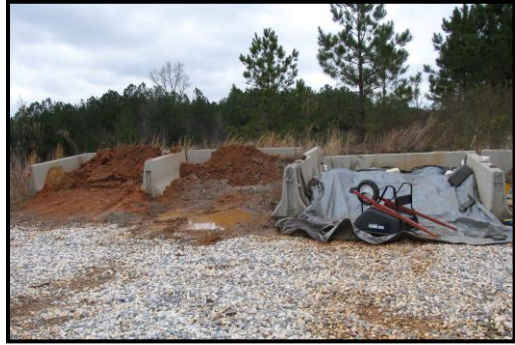
(b) Storage bins
