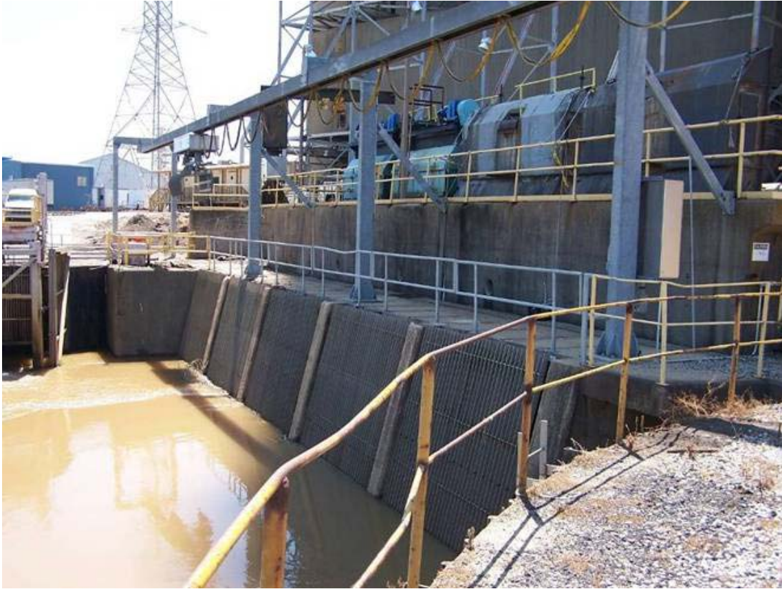
Figure 3. Plant Barry cooling water intake structure for steam generation Units 4 and 5.
