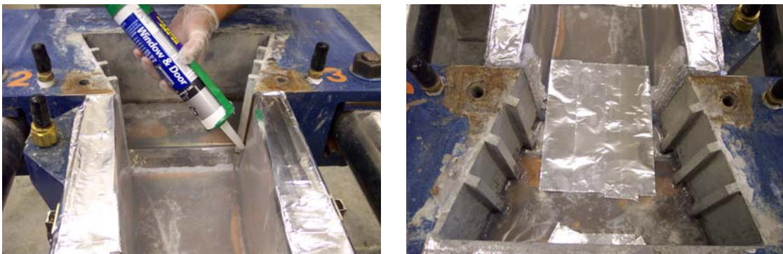
Figure 5-4: Caulking formwork and taping bottom crosshead braces
