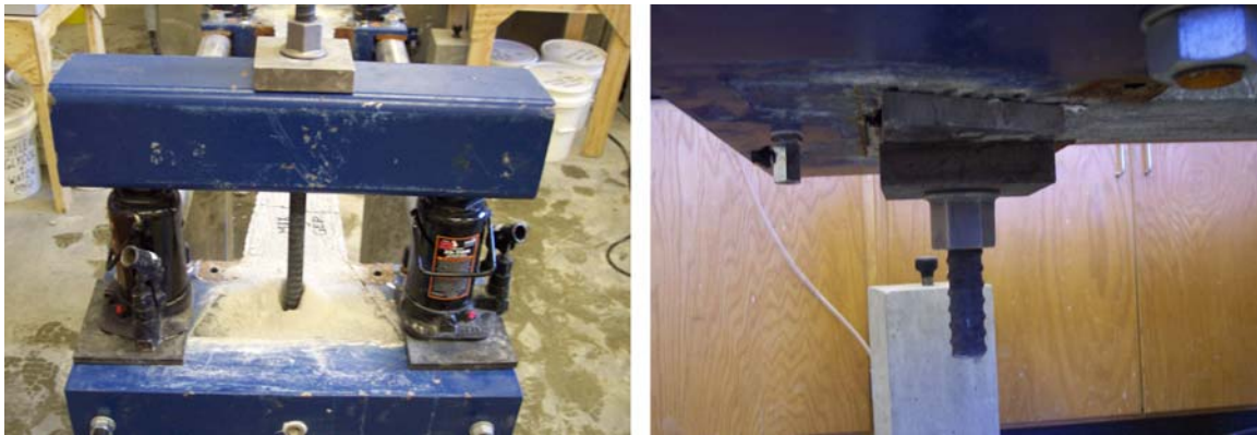
Figure C-23: Inserting and anchoring DYWIDAG bar
