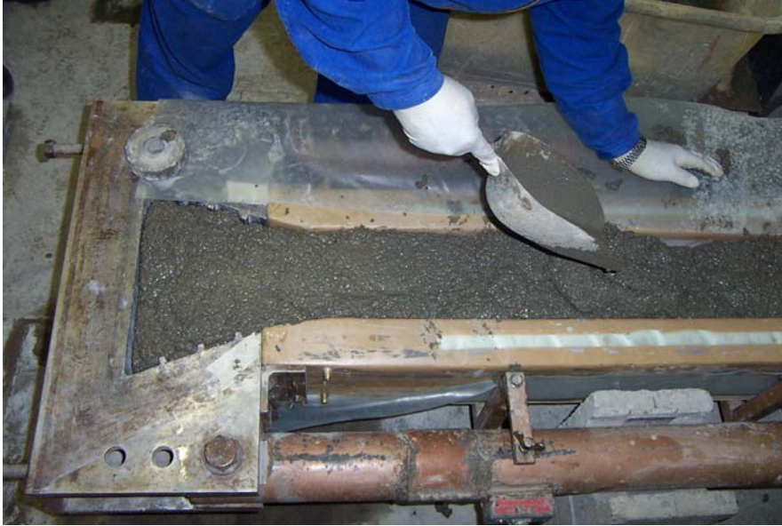
Figure A-2: Concrete placement
