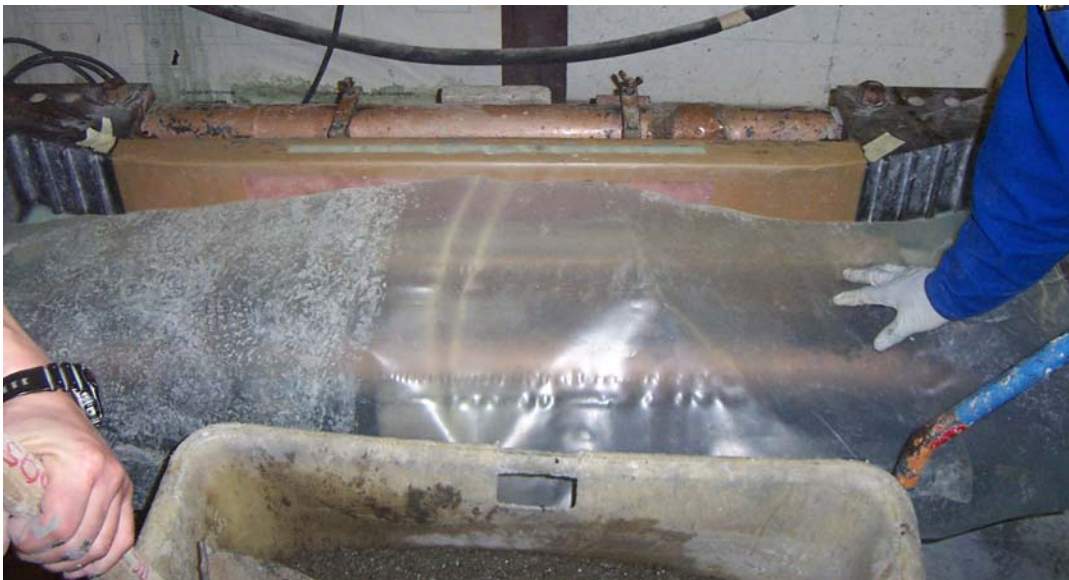
Figure A-1: Formwork preparation
