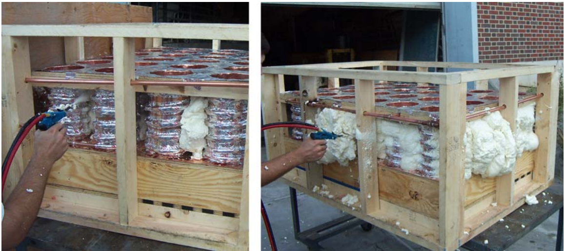
Figure D-6: Spraying foam insulation
