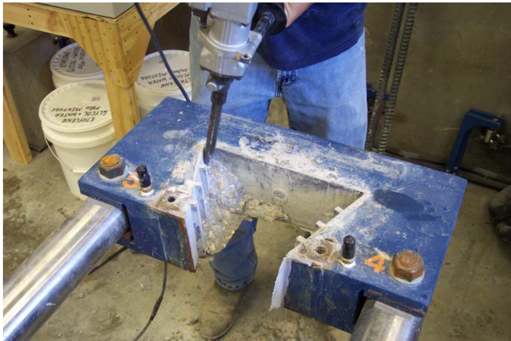
Figure C-25: Removal of residual concrete with a jackhammer
