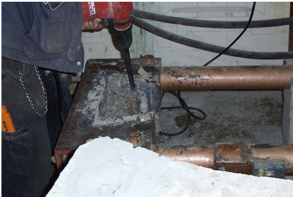
Figure A-13: Removal of residual concrete with a jackhammer
