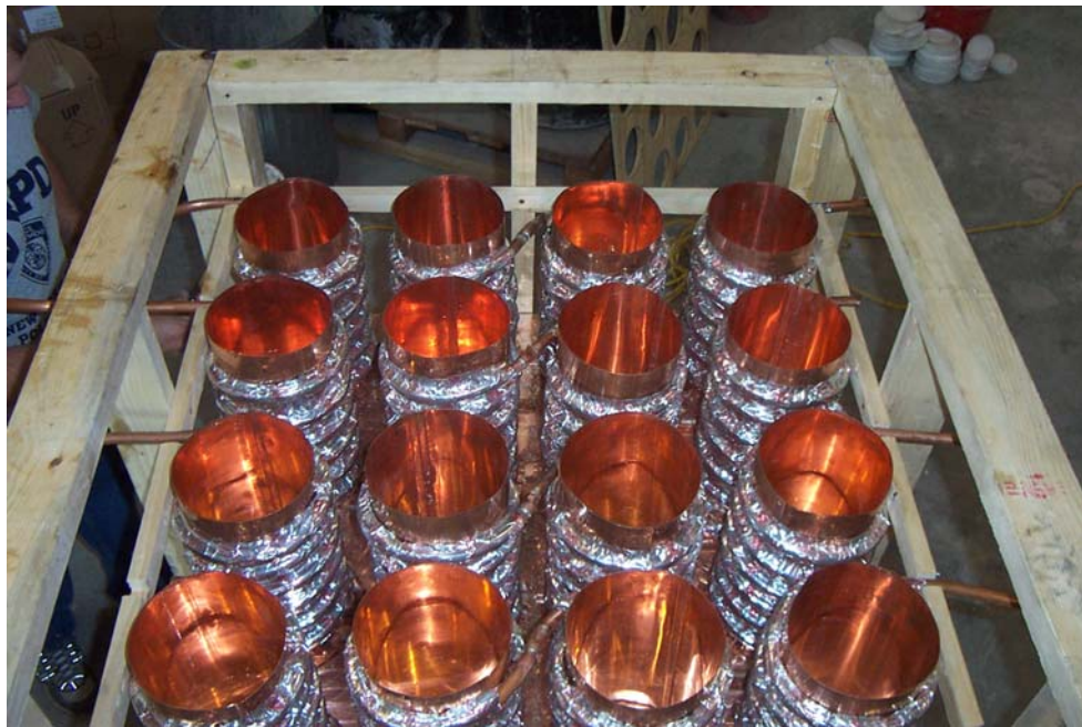
Figure D-4: Installing copper sleeves and copper tubing
