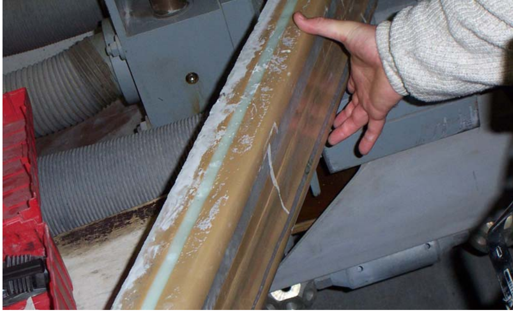
Figure A-10: Insulated formwork with copper water lines
