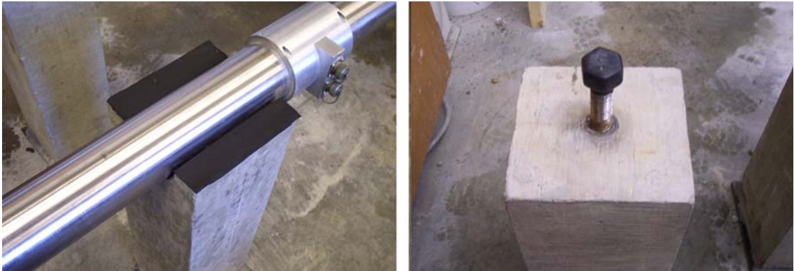
Figure C-9: Cracking frame supports
