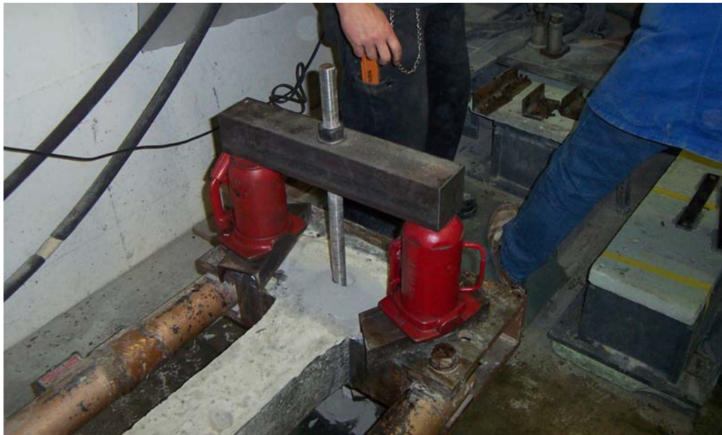
Figure A-15: Bottle jacks and steel rig
