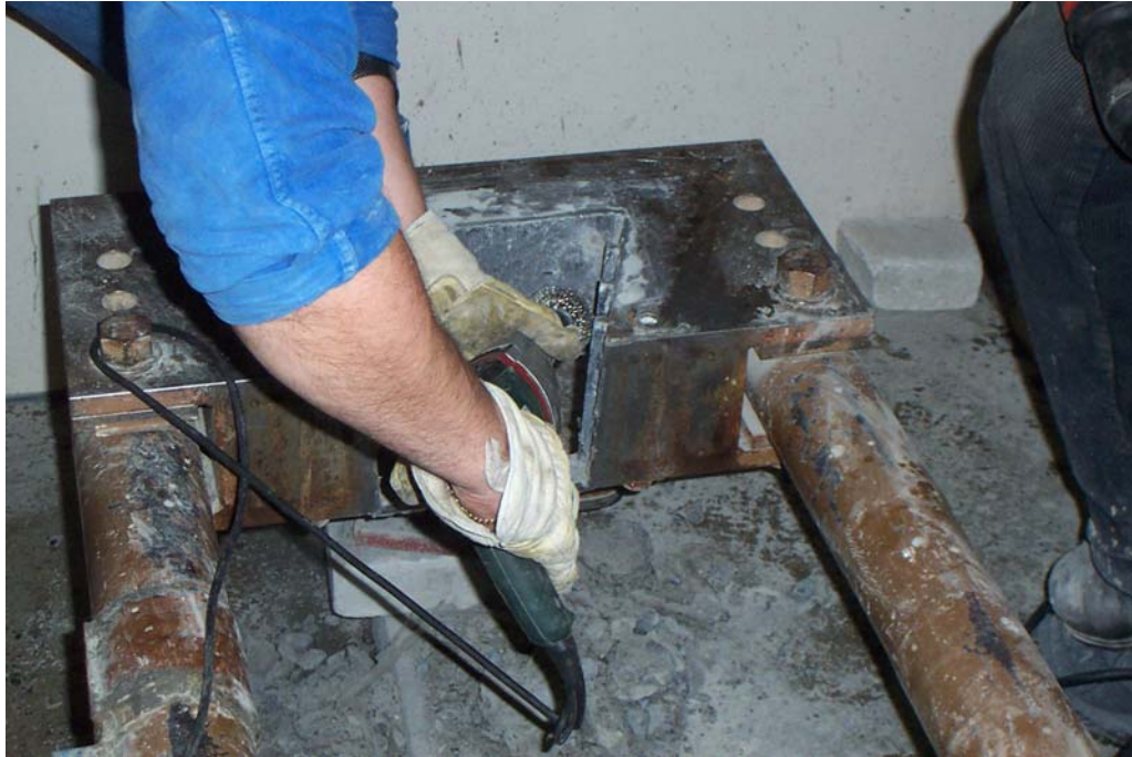
Figure A-14: Cleaning the crosshead with a steel brush
