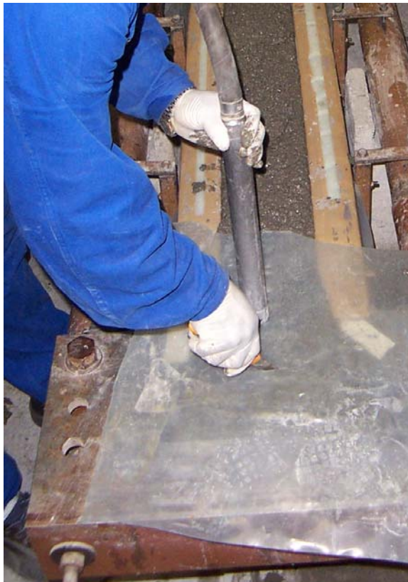
Figure A-3: Vibration of fresh concrete
