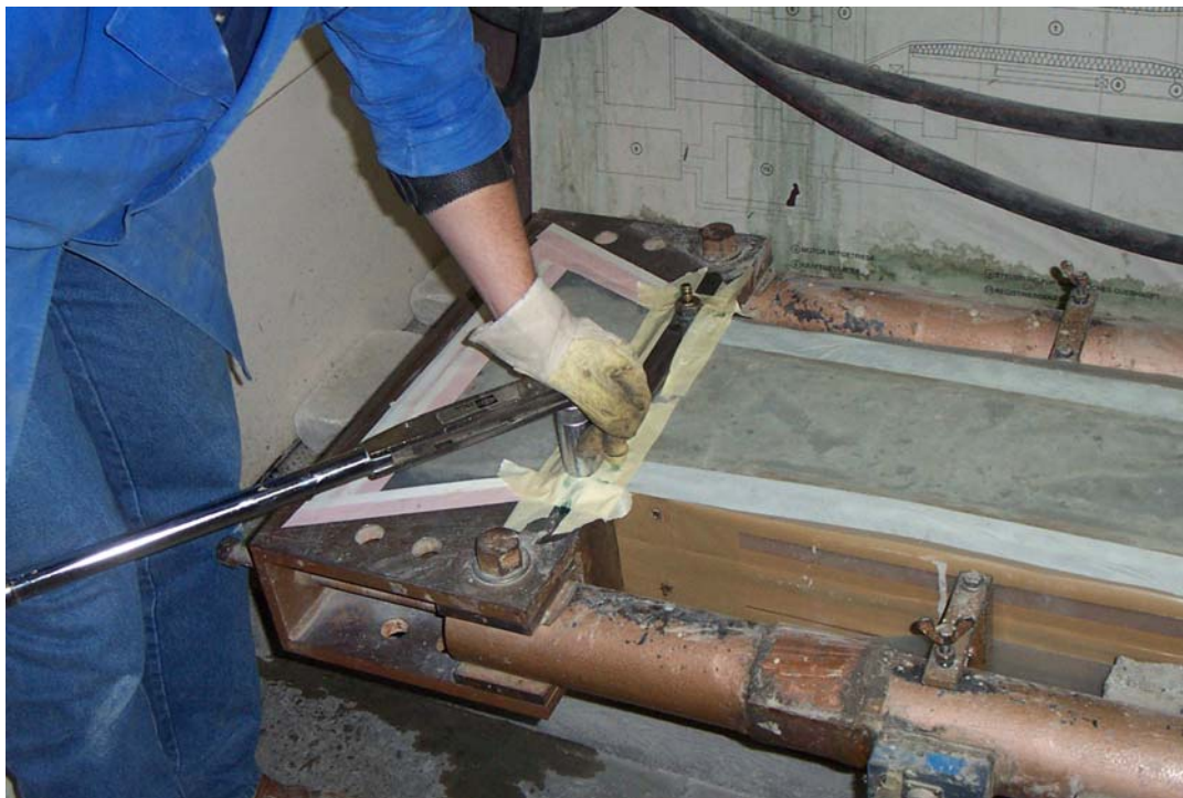
Figure A-5: Securing the crosshead braces with a torque wrench
