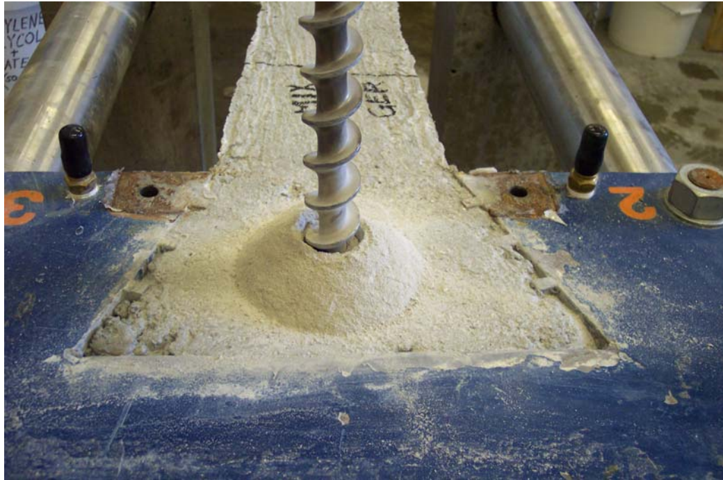
Figure C-22: Drilling a hole for a 1-in. threaded DYWIDAG bar
