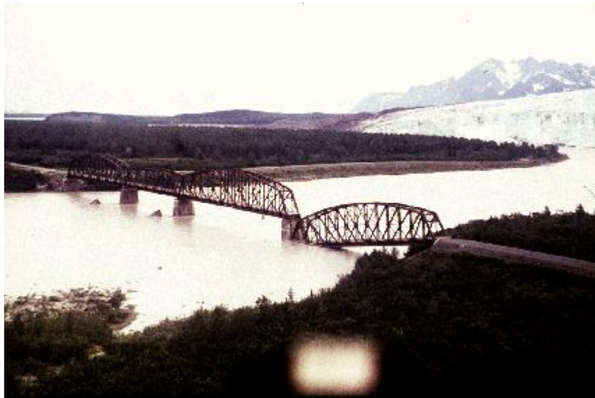
Figure 2.3: Damage to the “Million Dollar” railroad bridge due to lateral spread caused by the 1964 “Good Friday” earthquake (USGS 2006a)
