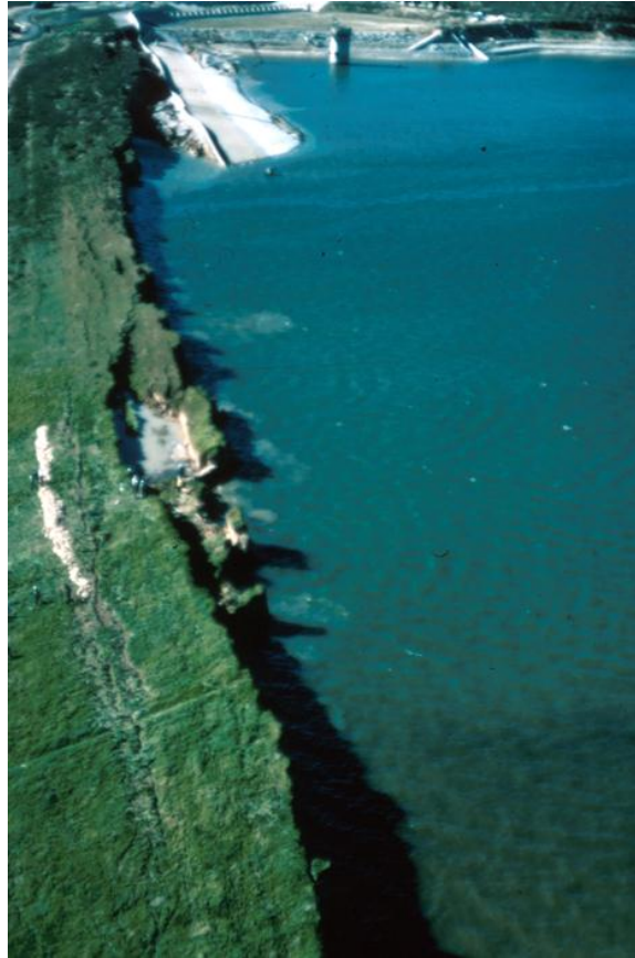
Figure 2.8: Aerial view of the Lower San Fernando Dam liquefaction-induced slope failure after the 1971 San Fernando, California, earthquake (USGS 2006b)
