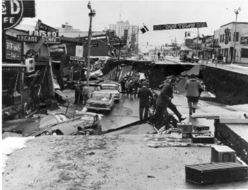
Figure 2.4: Liquefaction-induced ground movement in Anchorage, Alaska, after the 1964 "Good Friday" earthquake (USGS 2006a)
