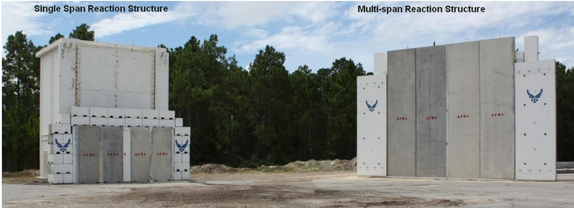
Fig. 3.24. Test set up for full-scale dynamic tests with single span reaction structure (left) and multi-span reaction structure (right)
