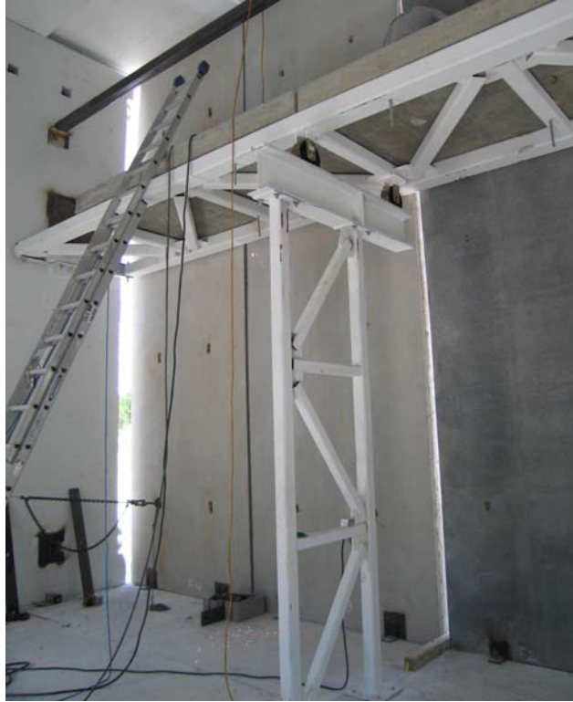
Fig. 3.39. Second floor support frame allowing interaction between the behaviors of all multi-span panels attached
