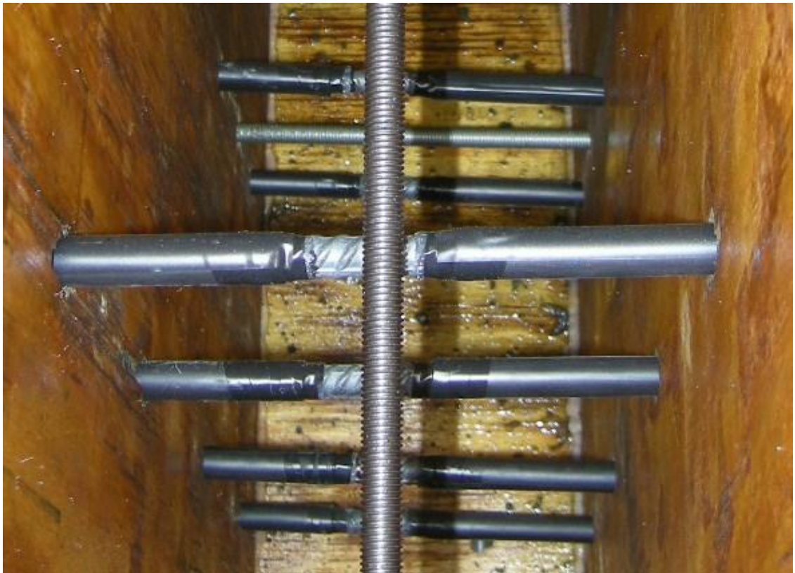
Figure 3.13: Pullout bars positioned prior to concrete placement
