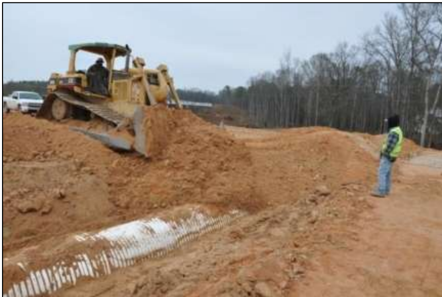
Figure 4-17: Bulldozer Backfilling PVC Pipe
