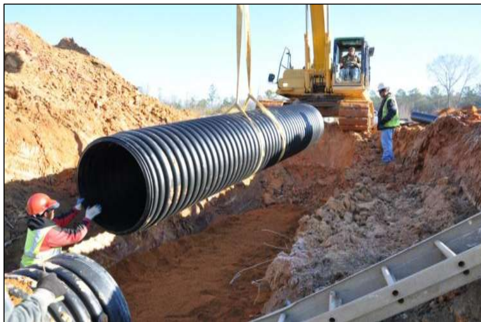
Figure D-4: Granular Backfill Installation at Station 223+00
