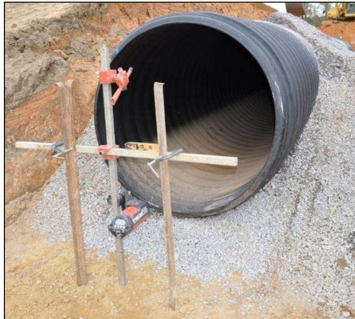
Figure 4-6: Grade Light 2500 Utility Alignment Laser
