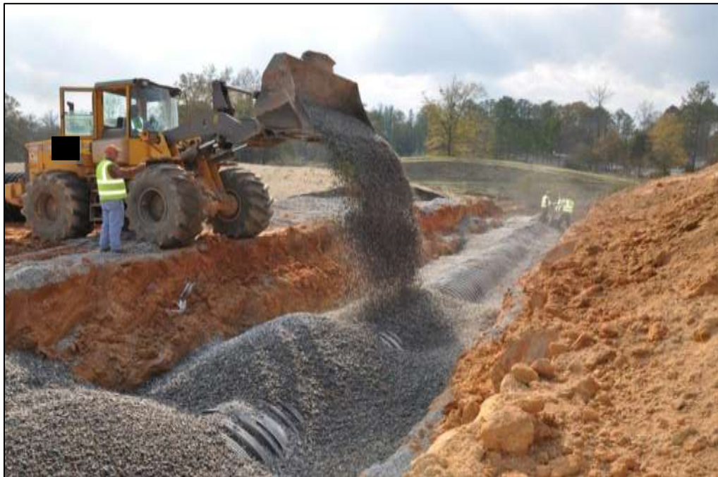
Figure C-12: Stone Backfill Installation at Station 224+00
