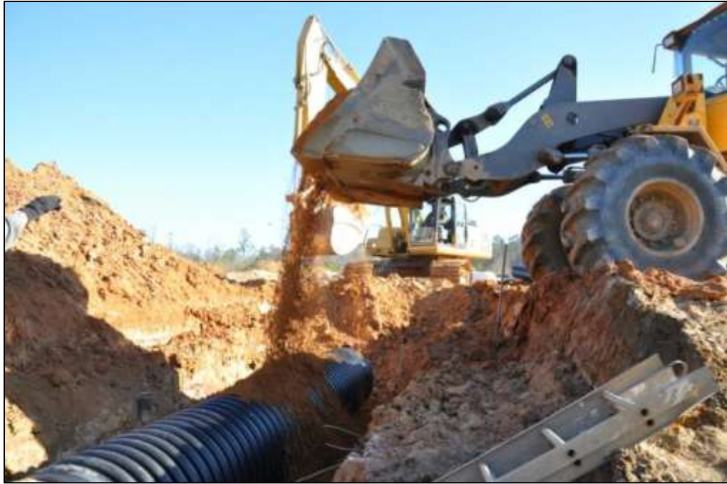
Figure D-5: Granular Backfill Installation at Station 223+00
