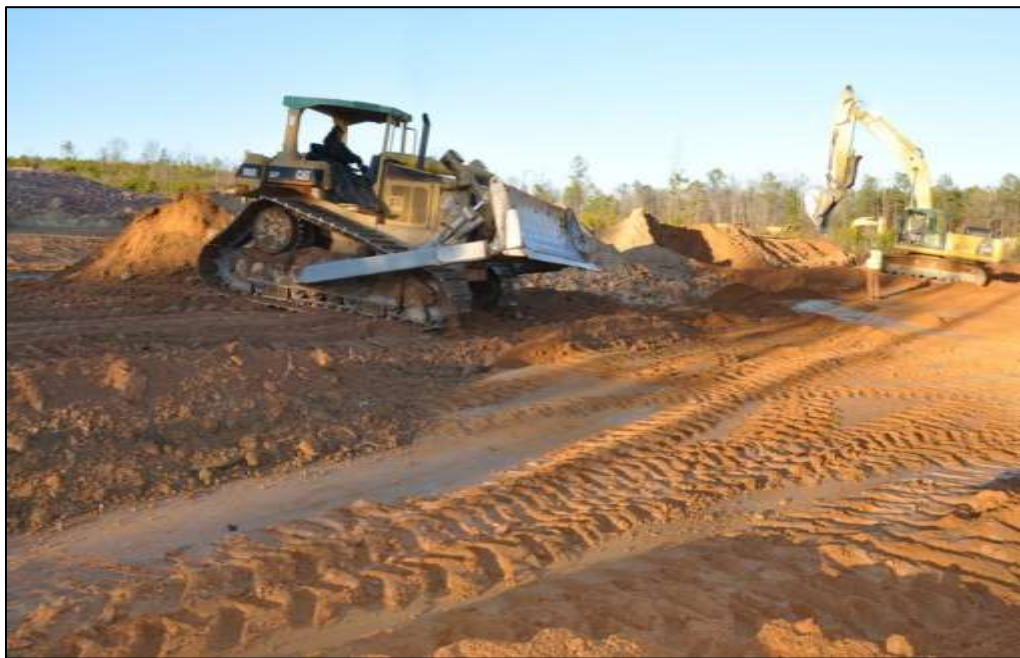
Figure D-16: Granular Backfill Installation at Station 223+00
