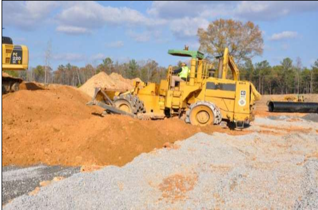
Figure C-15: Stone Backfill Installation at Station 224+00
