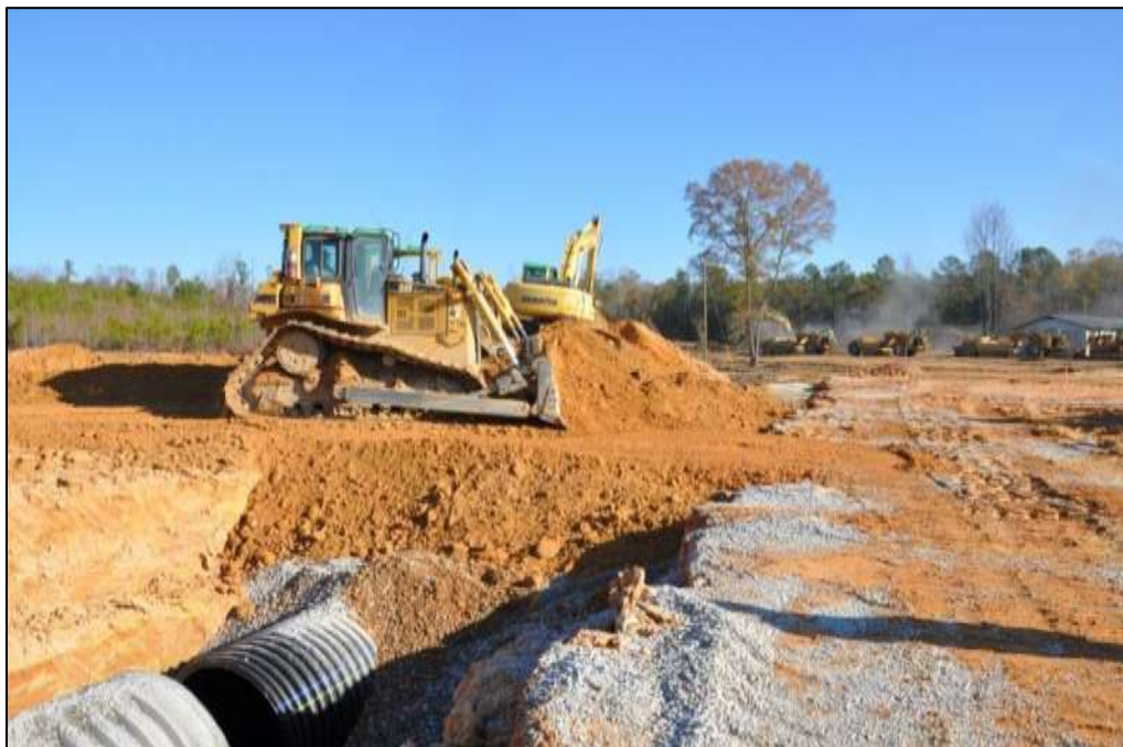
Figure C-16: Stone Backfill Installation at Station 224+00
