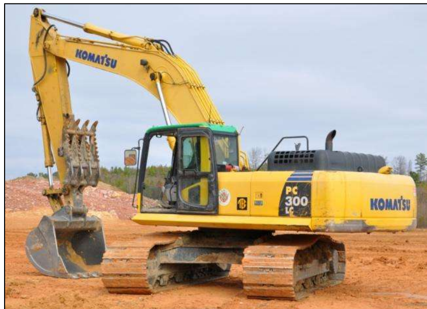
Figure 4-5: Excavator Used During Construction
