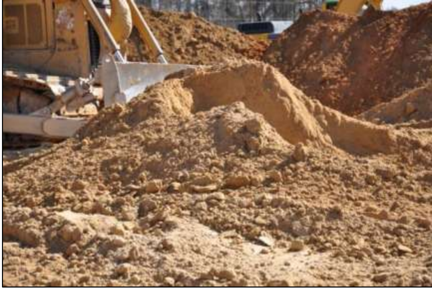
Figure 4-10: Yellow Sand with Gravel – ASTM Class III Backfill
