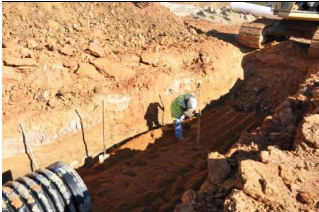
Figure D-6: Granular Backfill Installation at Station 223+00
