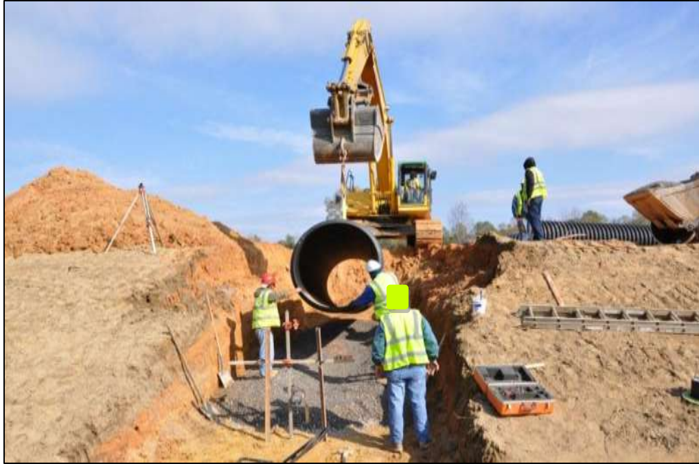
Figure C-3: Stone Backfill Installation at Station 224+00
