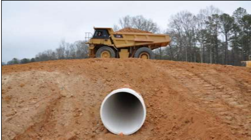
Figure 4-18: Loaded Dump Truck Crossing PVC Pipe
