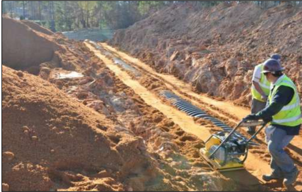
Figure D-13: Granular Backfill Installation at Station 223+00
