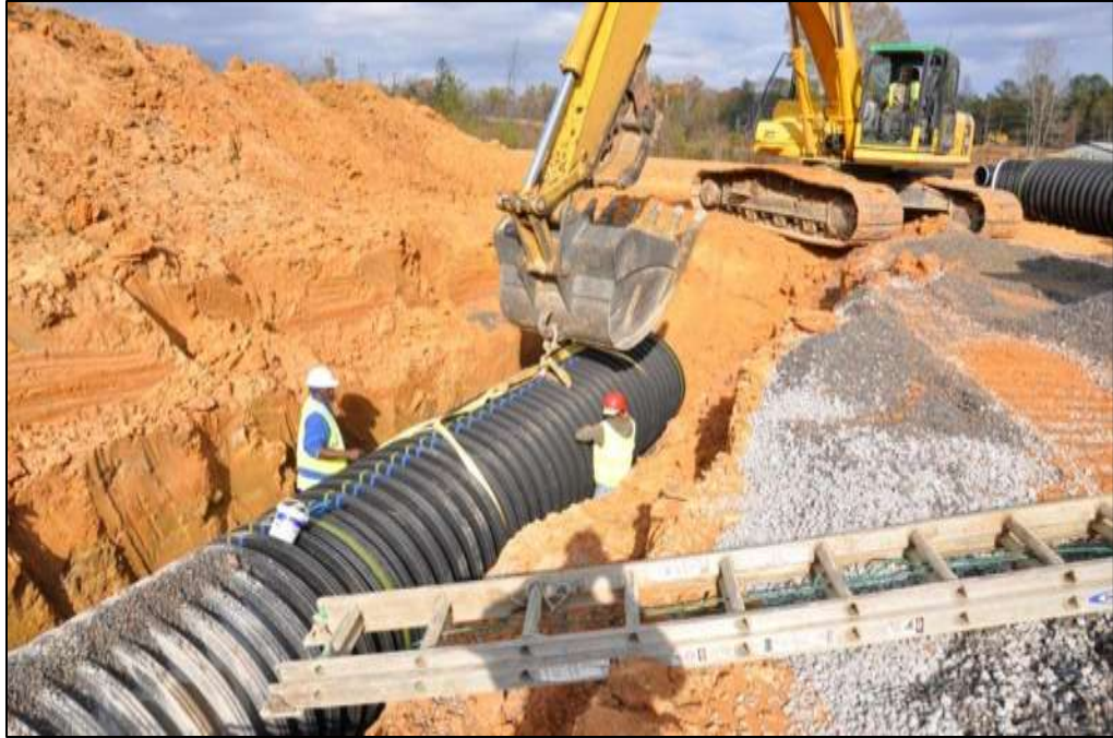
Figure C-7: Stone Backfill Installation at Station 224+00
