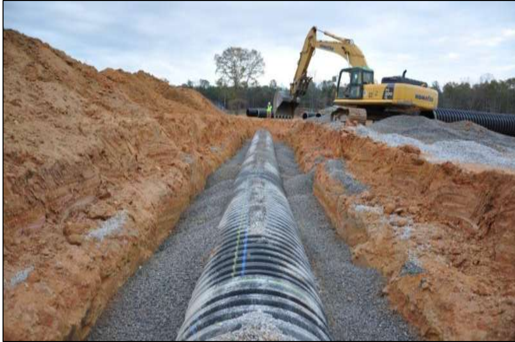
Figure C-11: Stone Backfill Installation at Station 224+00
