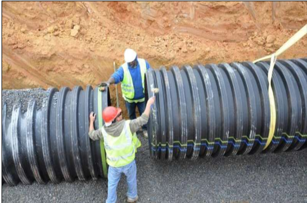
Figure C-6: Stone Backfill Installation at Station 224+00
