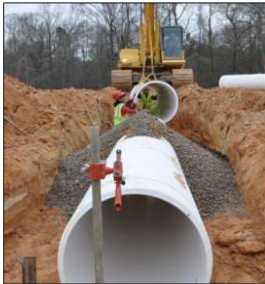
Figure 4-16: Stone Used to Hold Pipe in Place
