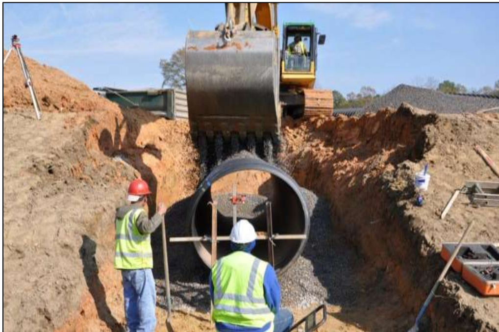
Figure C-4: Stone Backfill Installation at Station 224+00
