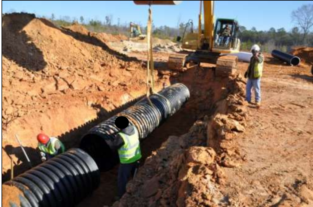
Figure D-7: Granular Backfill Installation at Station 223+00
