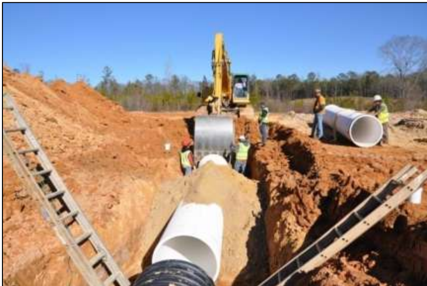
Figure 4-12: PVC Pipe Held in Place with Backfill
