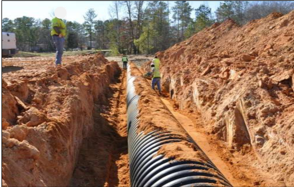
Figure D-9: Granular Backfill Installation at Station 223+00
