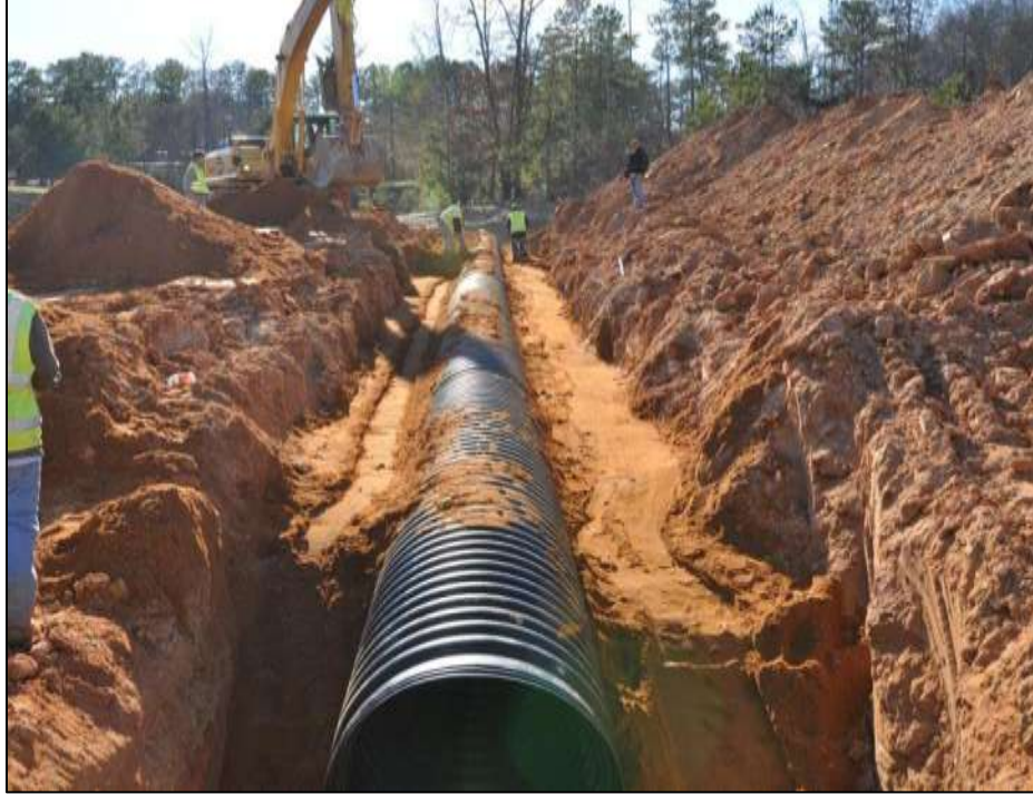
Figure D-11: Granular Backfill Installation at Station 223+00
