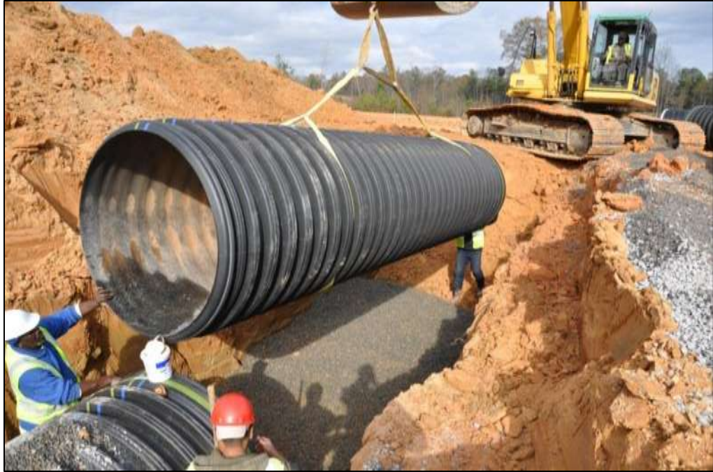
Figure C-5: Stone Backfill Installation at Station 224+00
