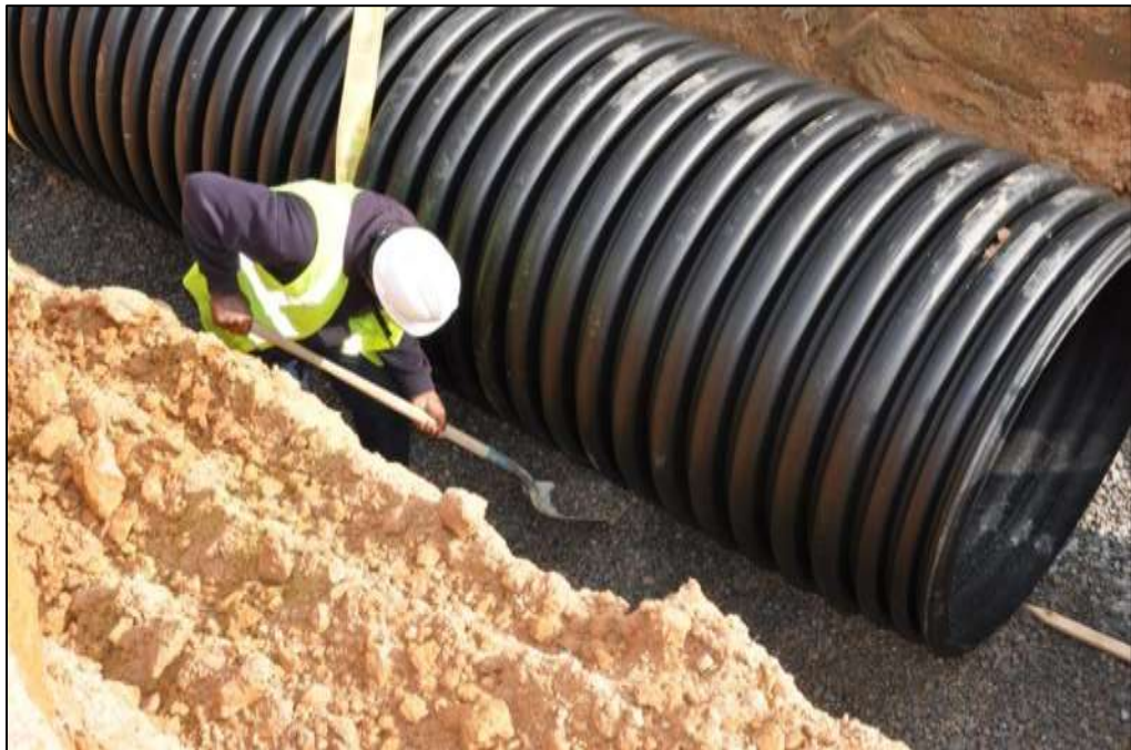
Figure C-8: Stone Backfill Installation at Station 224+00
