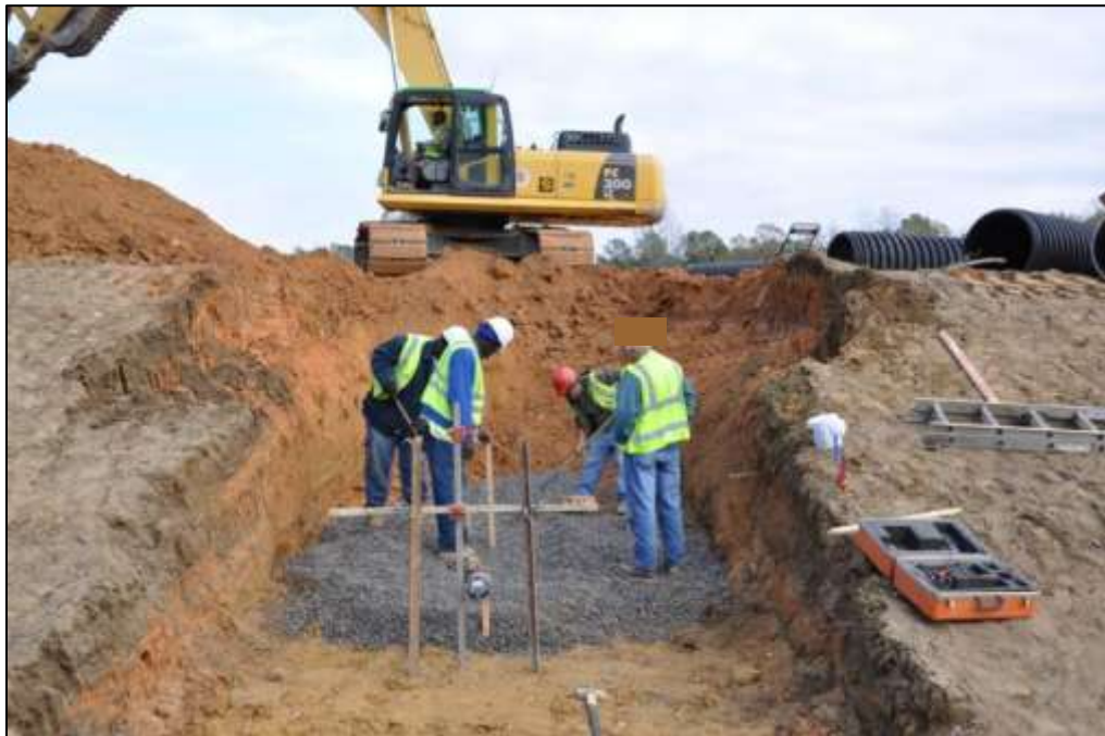
Figure C-2: Stone Backfill Installation at Station 224+00
