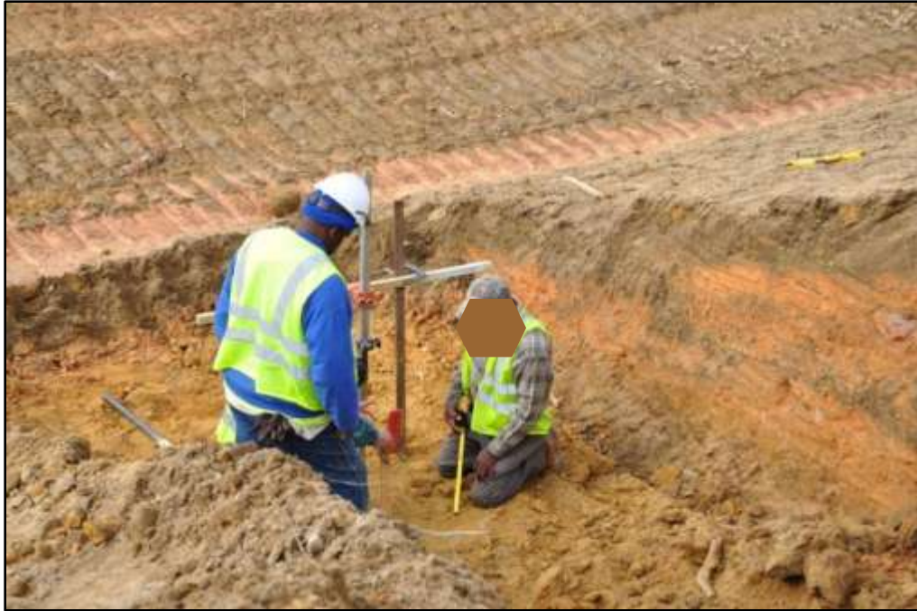
Figure C-1: Stone Backfill Installation at Station 224+00
