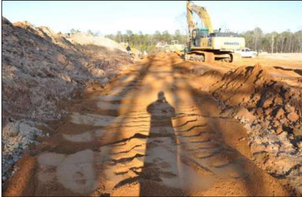
Figure D-15: Granular Backfill Installation at Station 223+00
