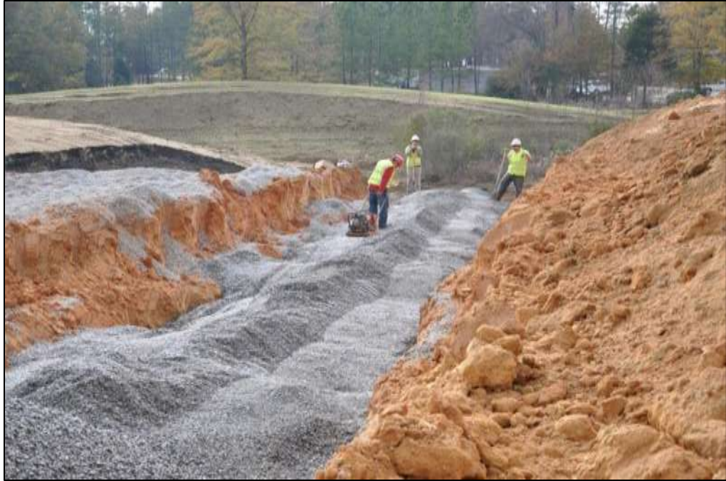
Figure C-13: Stone Backfill Installation at Station 224+00
