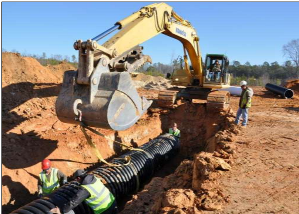
Figure D-8: Granular Backfill Installation at Station 223+00
