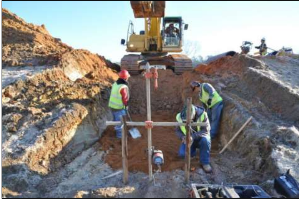
Figure D-1: Granular Backfill Installation at Station 223+00
