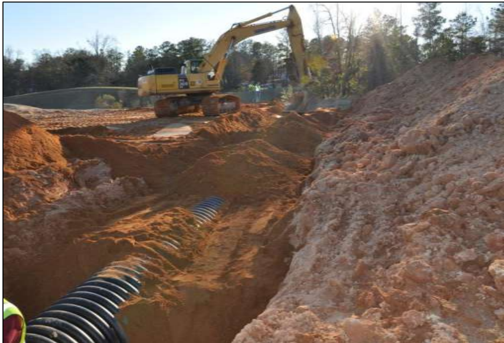
Figure D-14: Granular Backfill Installation at Station 223+00
