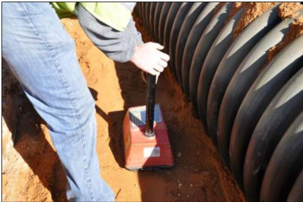
Figure D-10: Granular Backfill Installation at Station 223+00
