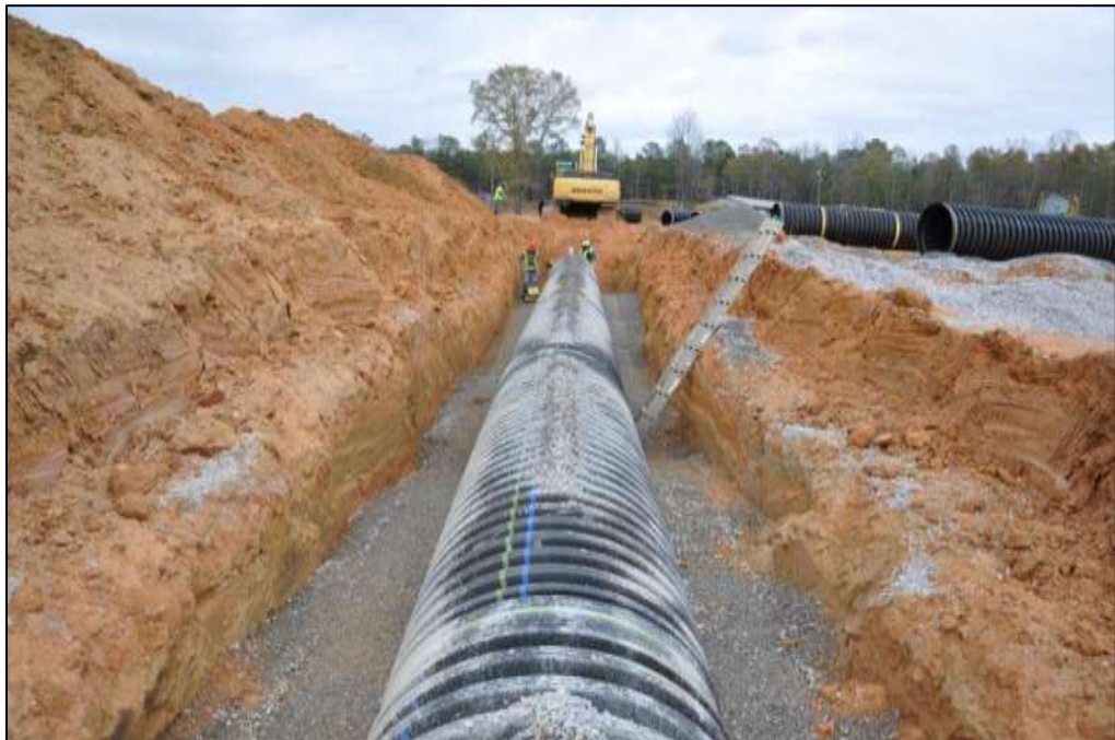
Figure C-10: Stone Backfill Installation at Station 224+00
