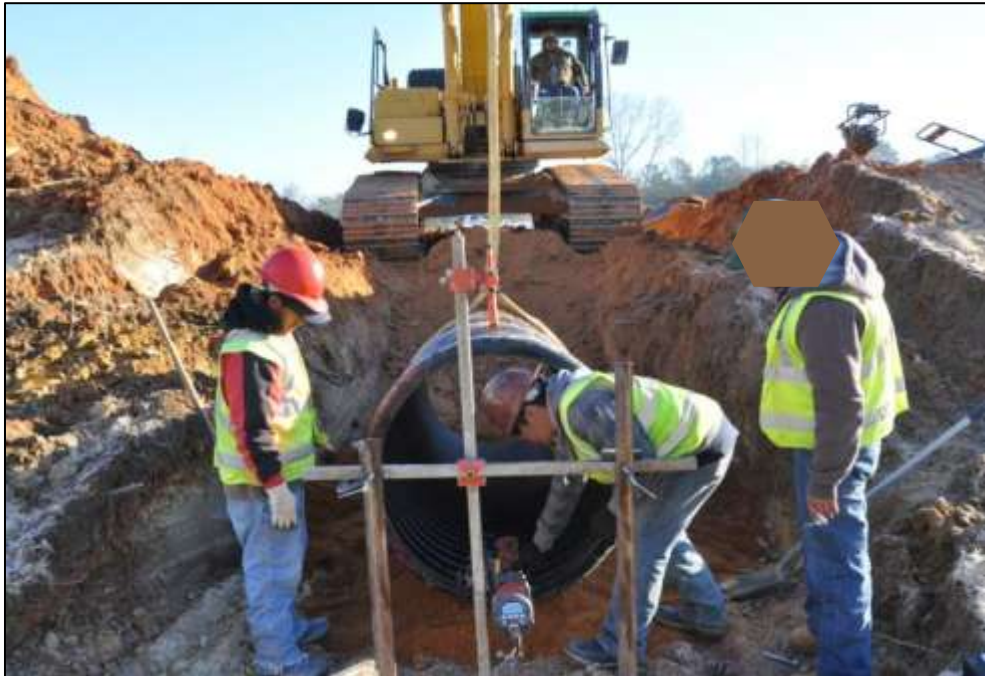
Figure D-2: Granular Backfill Installation at Station 223+00
