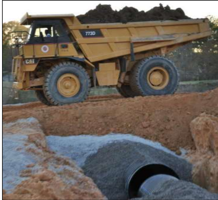
Figure 4-9: Dump Truck Crossing Pipeline
