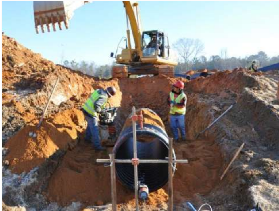
Figure D-3: Granular Backfill Installation at Station 223+00
