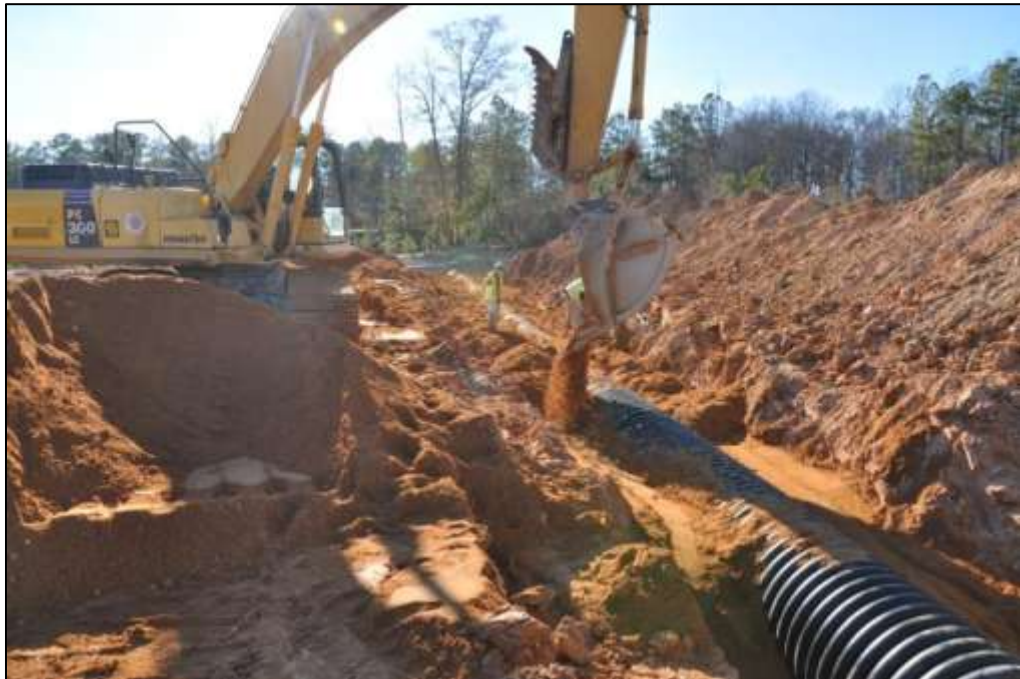
Figure D-12: Granular Backfill Installation at Station 223+00
