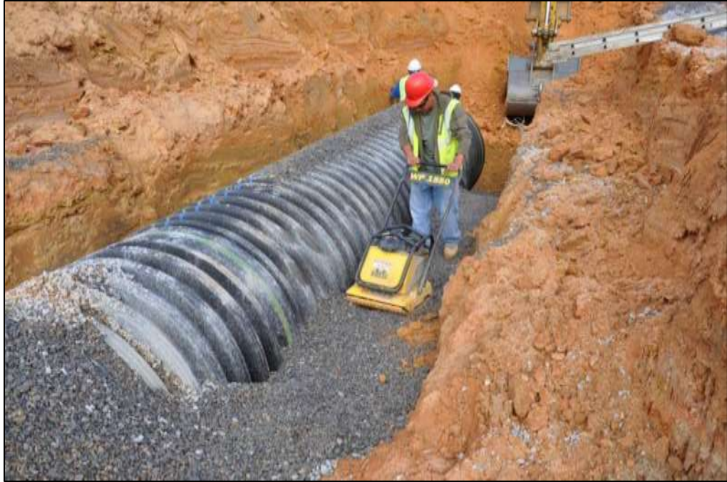
Figure C-9: Stone Backfill Installation at Station 224+00
