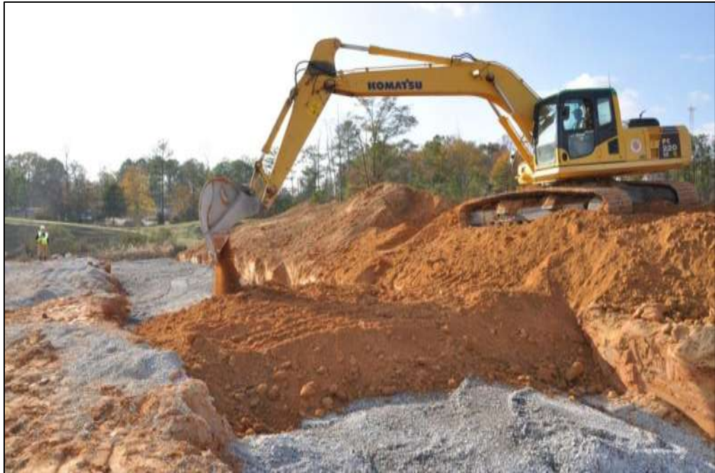
Figure C-14: Stone Backfill Installation at Station 224+00
