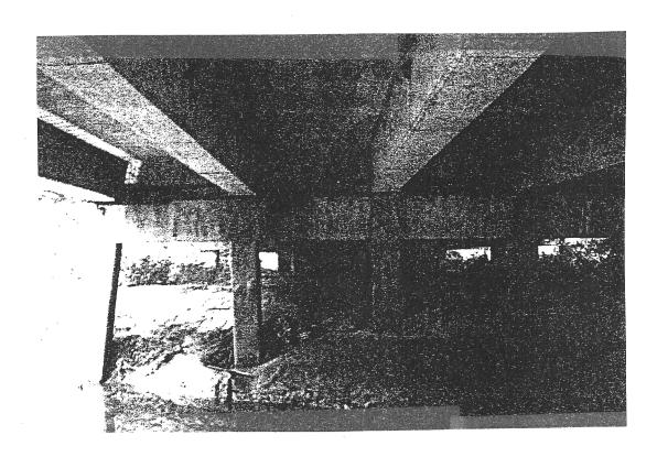
Figure 2.2 One-Story Bridge with Steel H-Pile Encased and Sway-Bracing Omitted
