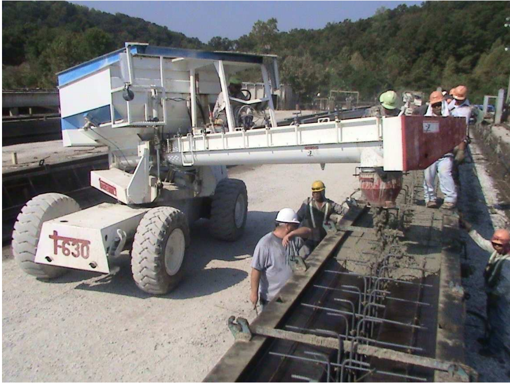
Figure 3-20: Concrete Delivery Vehicle Placing Concrete
