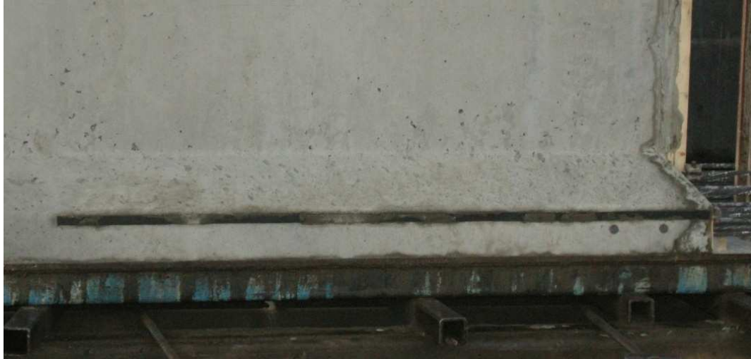
Figure 4-6: Exposed DEMEC Strip Immediately After Form Removal
