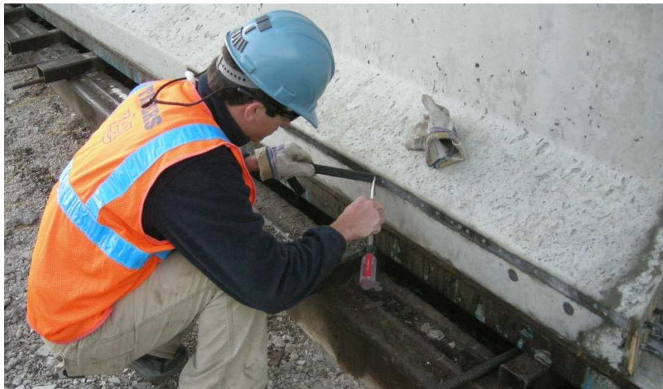
Figure 4-7: Removal of Foam Adhesive
