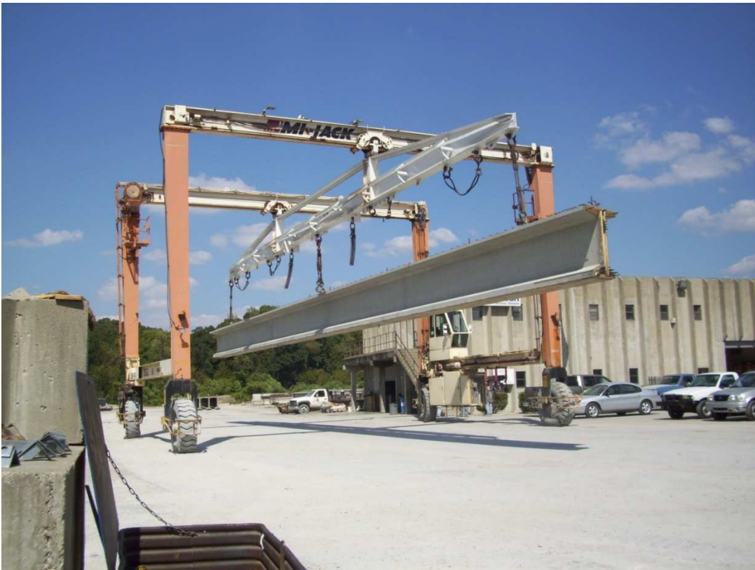
Figure 3-32: Transporting BT-54 Girder to the Storage Yard
