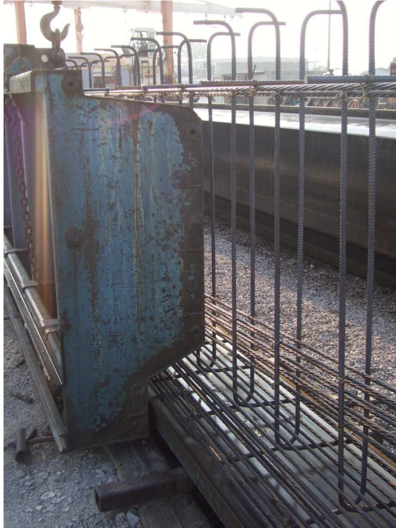
Figure 3-19: Formwork Being Put into Place
