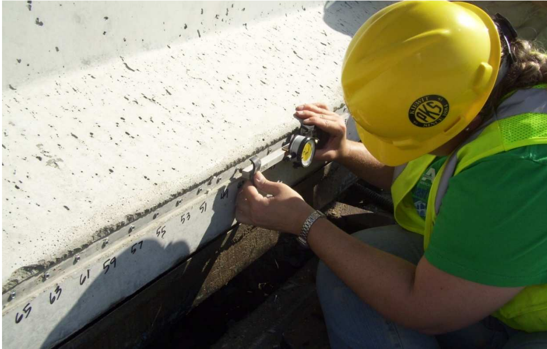
Figure 4-12: Performing DEMEC Strain Measurement
