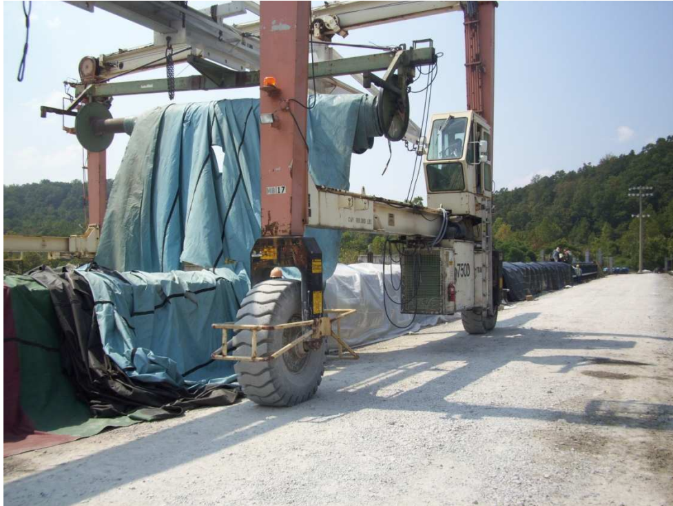
Figure 3-27: Curing Blankets and Placement of Weatherproof Tarp
