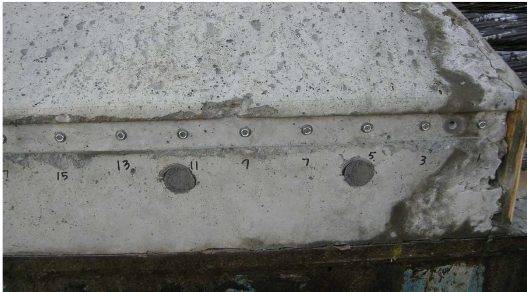
Figure 4-10: Finalized DEMEC Target Installation
