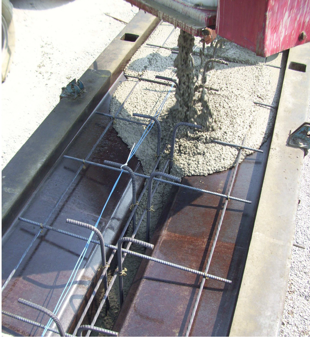
Figure 3-25: Placement of Self-Consolidating Concrete
