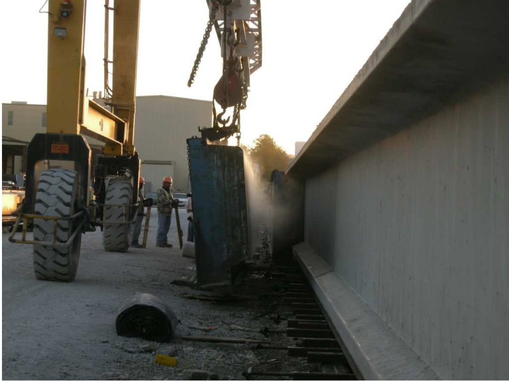
Figure 3-28: Removal of Side Forms
