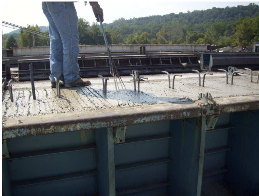
Figure 3-26: Concrete Surface Roughening
