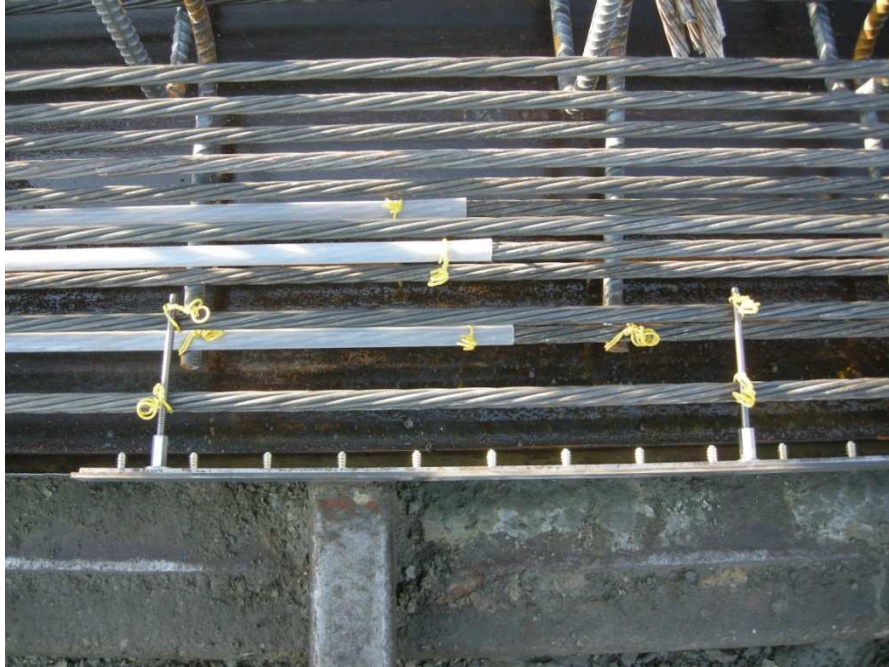
Figure 3-18: DEMEC System Tied into Steel Cage
