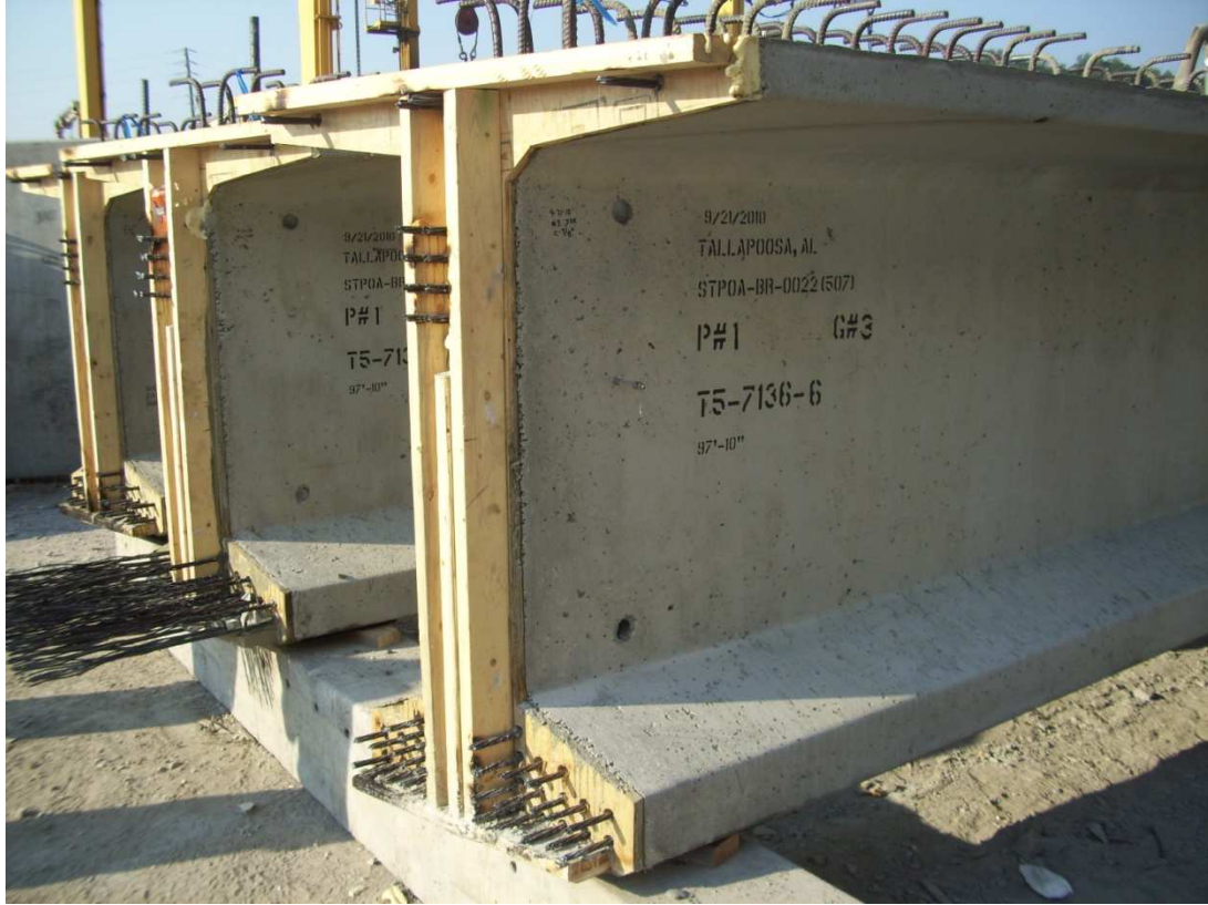
Figure 3-33: Girder Support Conditions in Storage Yard
