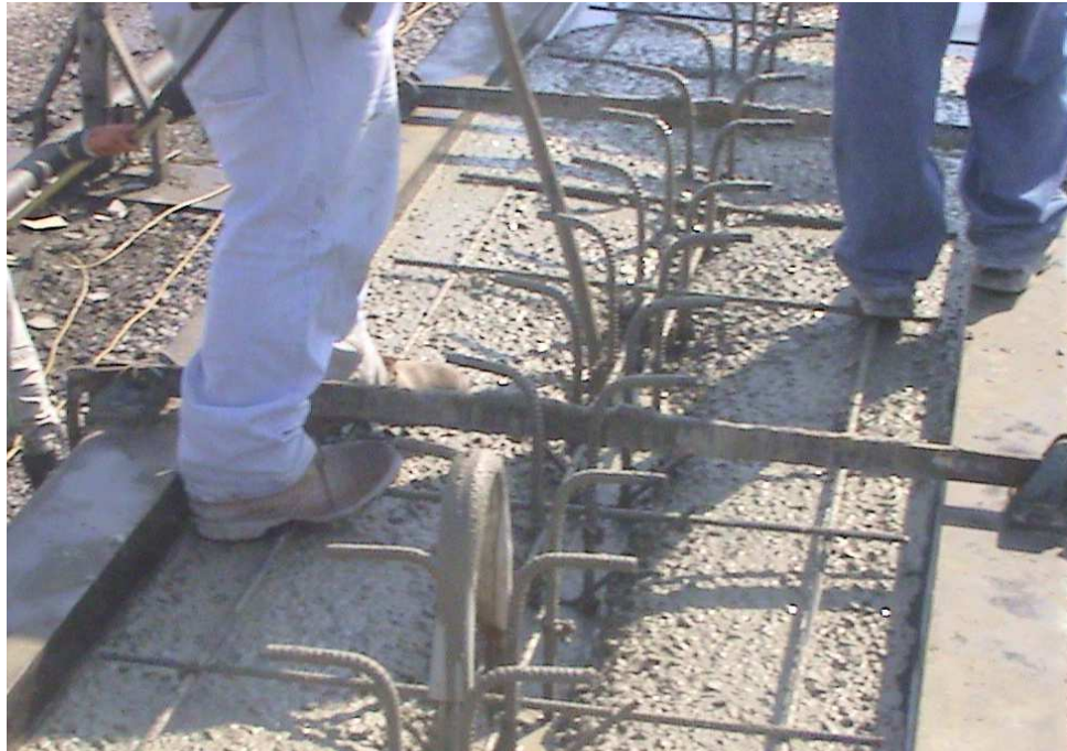
Figure 3-24: Internal Vibration of Concrete
