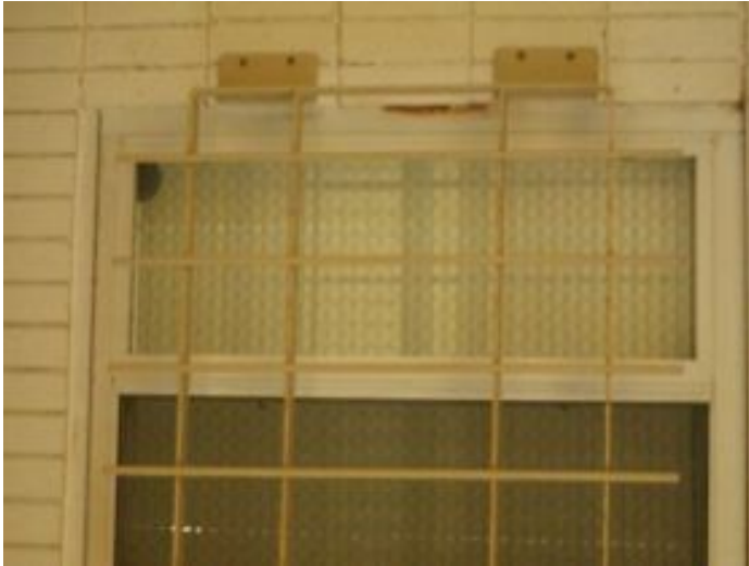
Figure 14: Security measure at the pharmacy site; all windows had bars on them.
