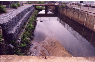
Existing Gabion Walls along Village Creek through Birmingham Airport
