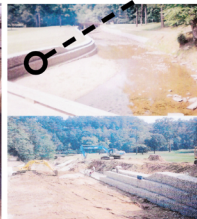
Existing Gabion Walls along Valley Creek in Birmingham
